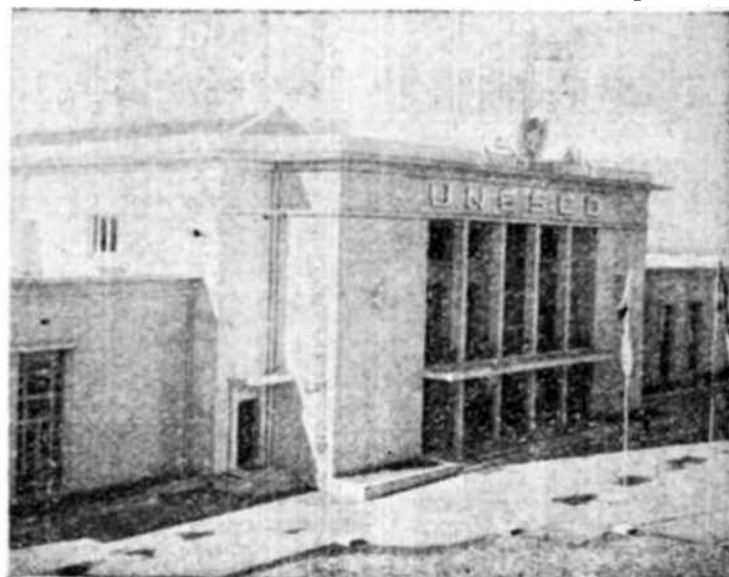
View of main Conference Hall of the "Palais de l'Unesco" in Beirut
