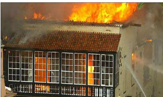
Fig. 1 The fire at Episcopal Residence of San Cristóbal de La Laguna
