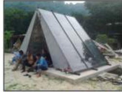
The completed installation of the pioneer project
