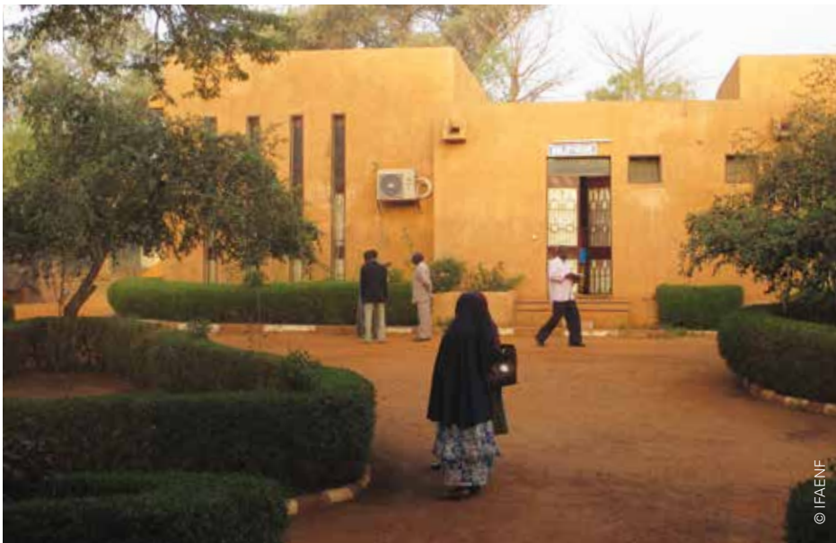
Figure 5.6 Library on the campus of the IFAENF
