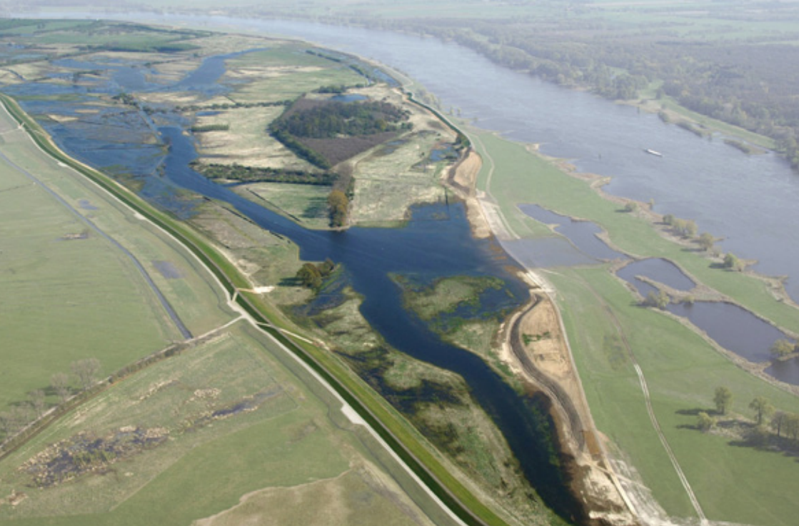
The area won by relocating the Lenzen dyke (© Flusslandschaft Elbe Brandenburg)
