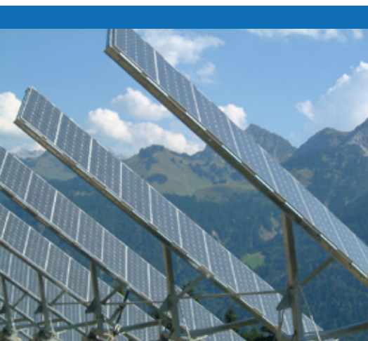
Photovoltaics at Blonz (© Gr. Walsertal BR)
