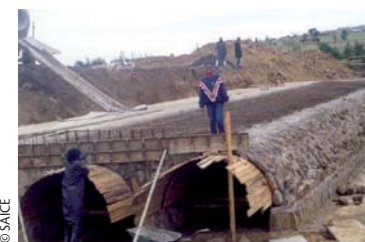
Stone arch construction.
