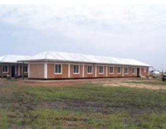
⤴ A health centre built with Stabilised Soil Blocks in Upper Nile Sudan.
