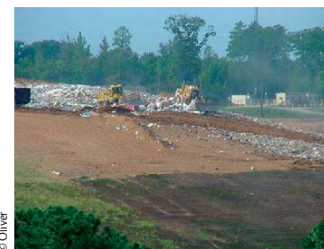
🗑️ Trash being loaded and compacted in a landfill.
