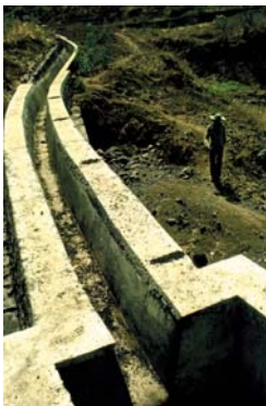
Water tank branch canal, Cape Verde.
