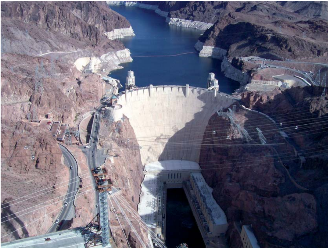
© Hoover Dam, USA.
