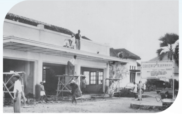
The Freedom Building, Bandung, where the Asian African Conference was held, in the process of construction
