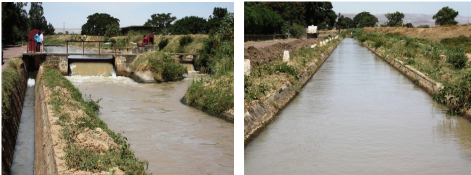
a. Flow over weir at d/s end of settling basin b. Main canal after the settling basin Figure 3.2. Wonji-Shoa scheme main canal head reach
