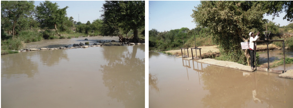
a. Temporary diversion for Golgota Scheme b. Regulating gates on main canal banks Figure 3.5. Water acquisition and control structures for Golgota Scheme
