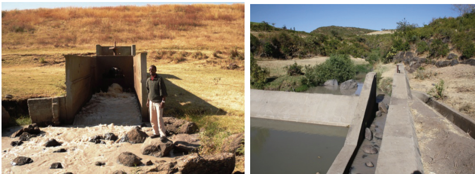
a. Wedecha Reservoir outlet b. Diversion structure to Godino sub-system Figure 3.6. Water acquisition and control structures for Wedecha Scheme
