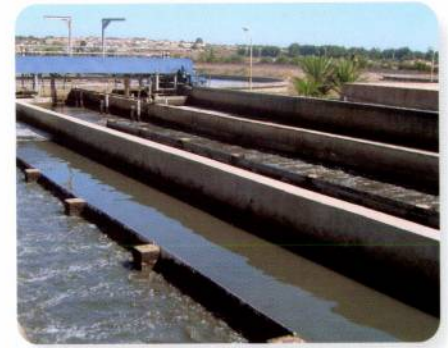
Four images of the Réghaïa wastewater treatment plant
