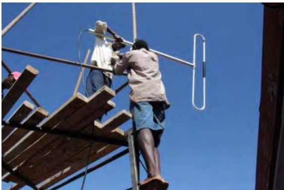
Fixing of the antenna on locally fabricated mast
