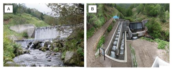
Fig. 4 Check dam before and after modification by installation of a fishway
