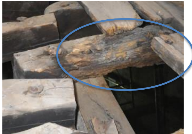
Figure 86: example of a purlin that need to be replaced because of the presence of an extensive biological decay.
