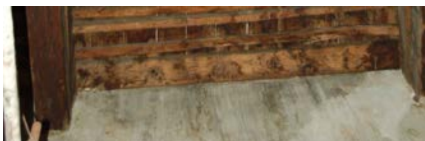
Figure 23: Rainwater leakage signs in the lateral nave close to the Orthodox side 3B
