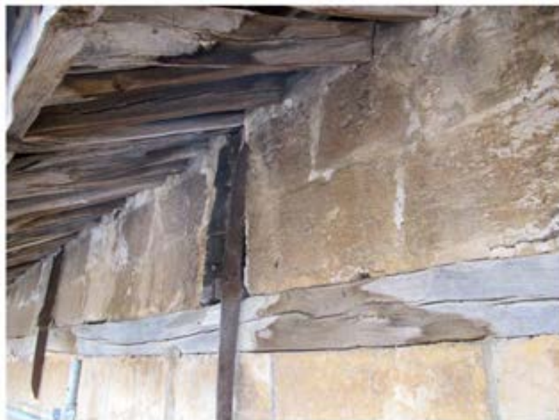
Figure 105: top portion of the wall with the wooden sleeper
