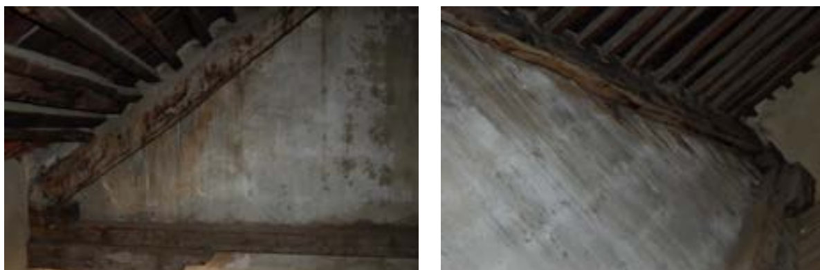
Figure 24: Rainwater leakage signs inside the central nave on the tympanum nearby the main entrance
