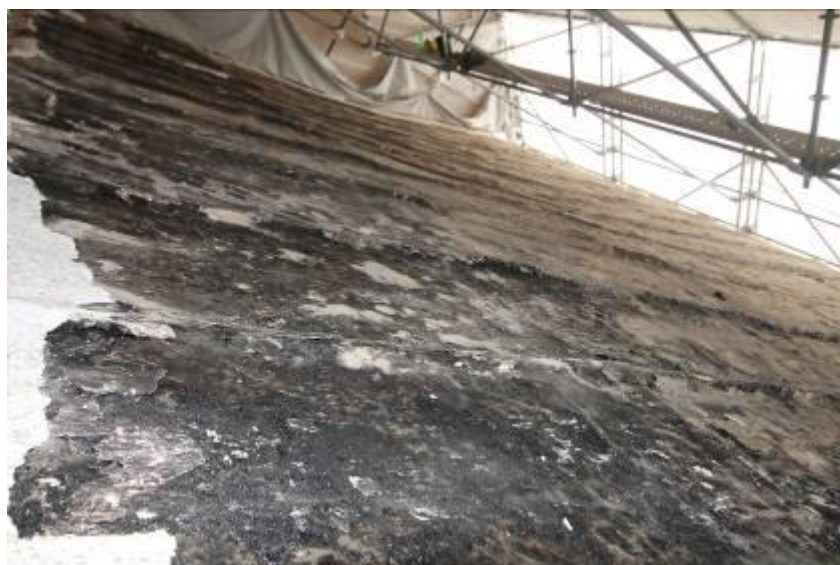
Figure 110: external surface of the roof made of bitumen and fabric
