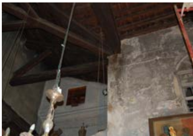
Figure 20: Damage due to the rain leakage in the Orthodox corner (2B)
