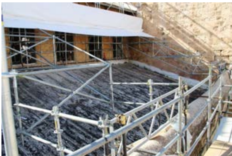
Figure 67: temporary roof above the North aisle (Franciscan side)
