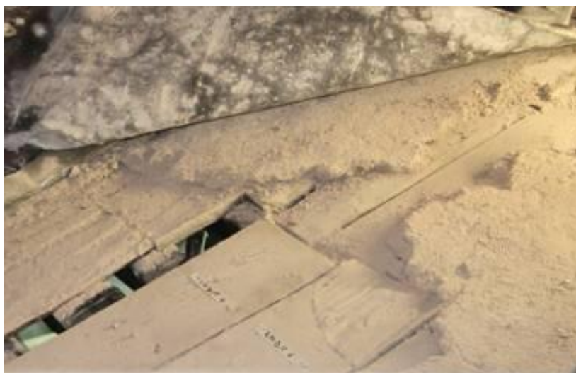
Figure 115: insulating layer made of clay and straw
