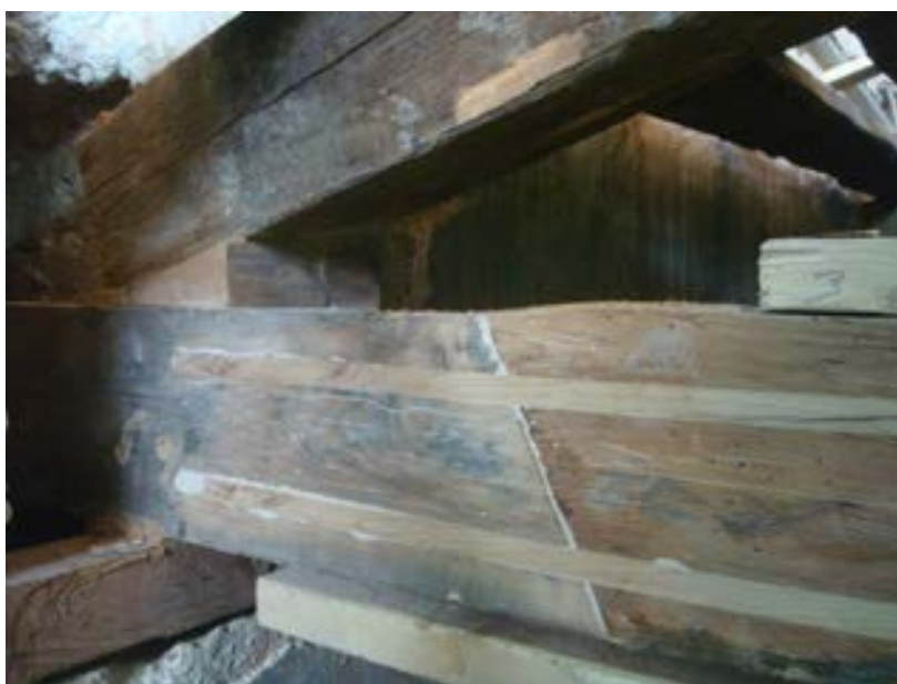
Figure 79: prosthesis already finished
