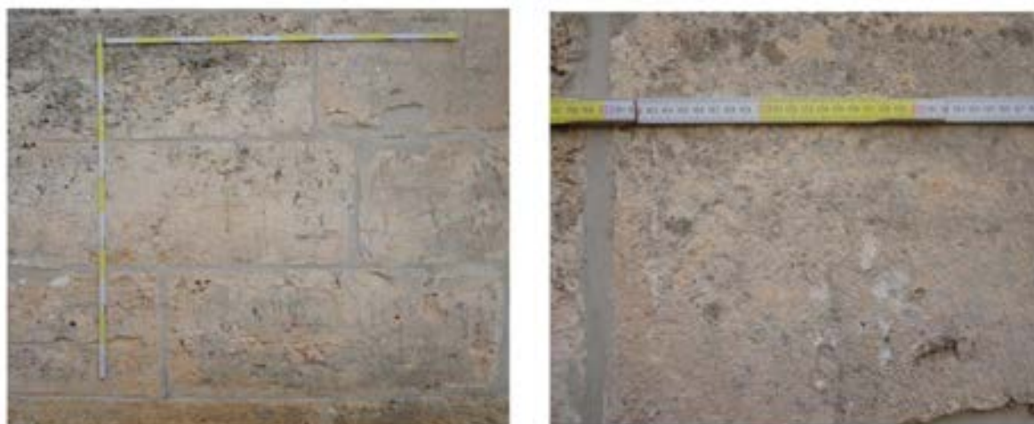
Figure 2: Building technique 1. Sample technique above. Traces of working tools at the bottom
