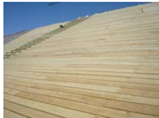
Figure 103: plywood; insulation layer (green), wooden laths and boards supporting the wool layer and the external lead sheets
