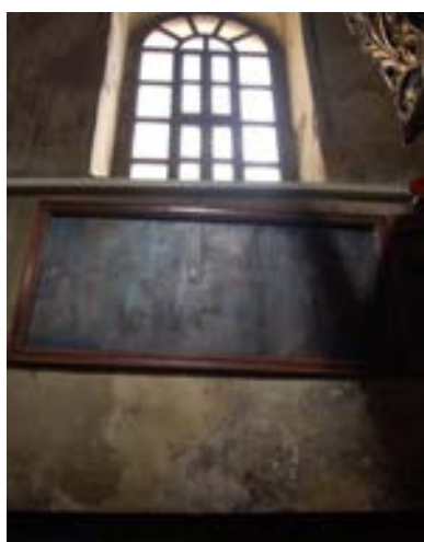
Figure 18: Damages on the wall due to the humidity on the other side (2A)
