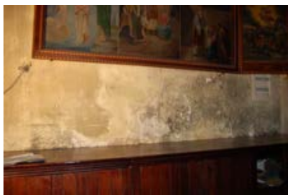
Figure 18: Damages on the wall due to the humidity on the other side (2A)
