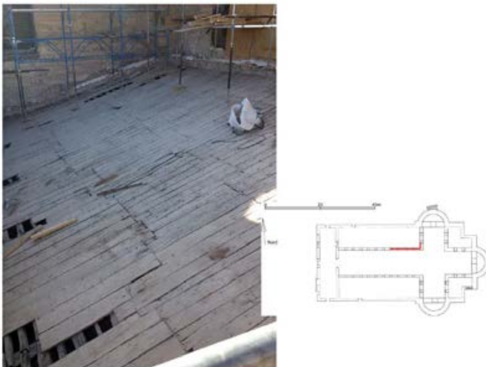
Figure 117: traces of previous roof structures in the areas between walls and present roof covering
