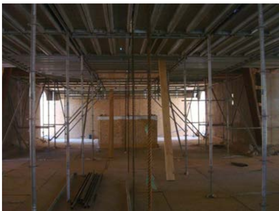
Figure 64: scaffolding in the central area – double deck and protection of the upper part of the iconostasis
