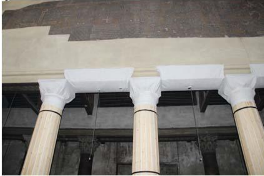
Figure 50: protection for capitals and architrave
