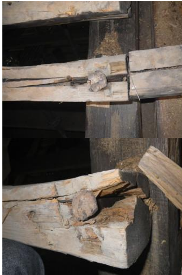
Figure 84: two examples of purlins to be replaced.
