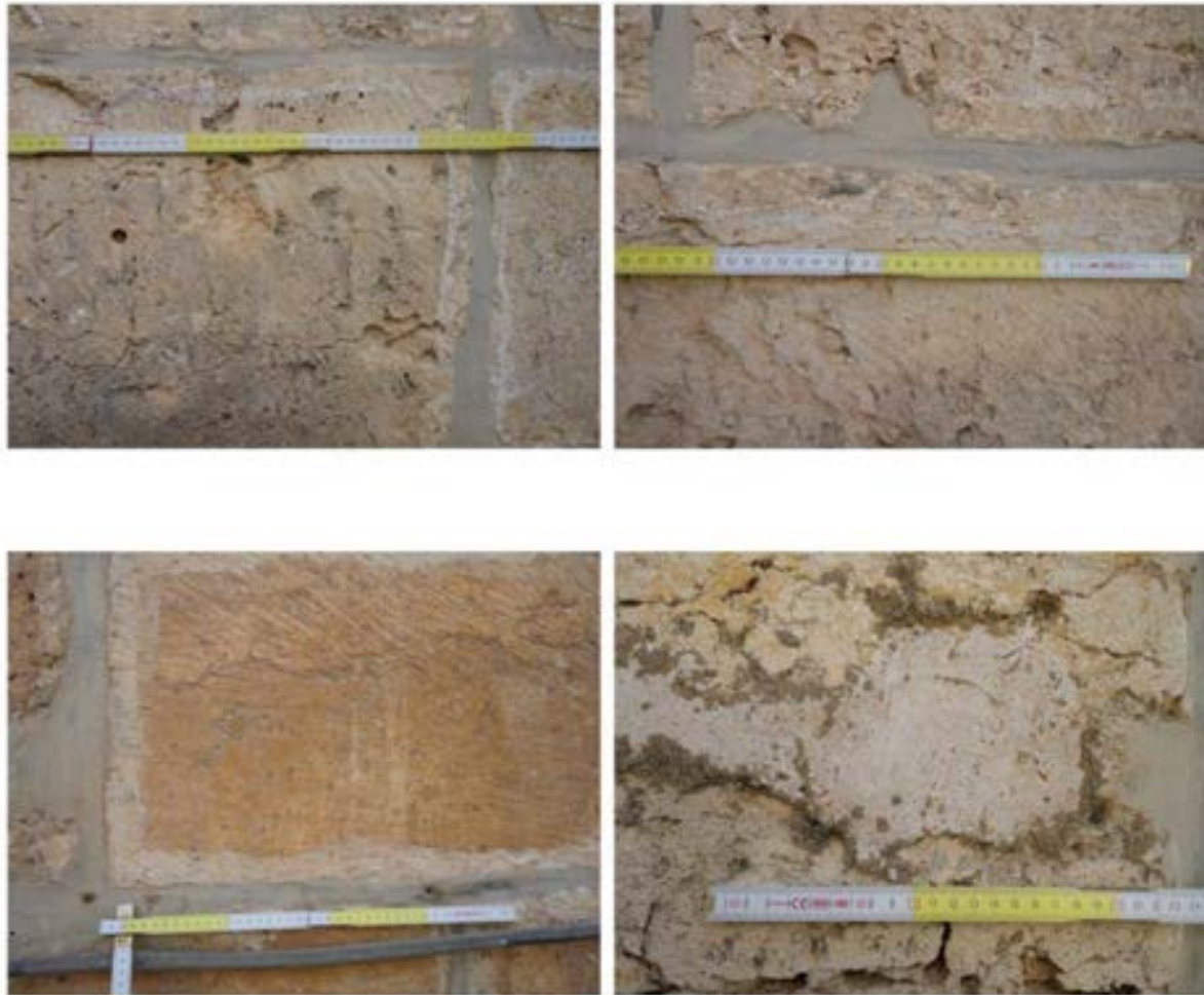
Figure 1: traces of mortar and finishing that characterize the eastern and northern walls of the apse
