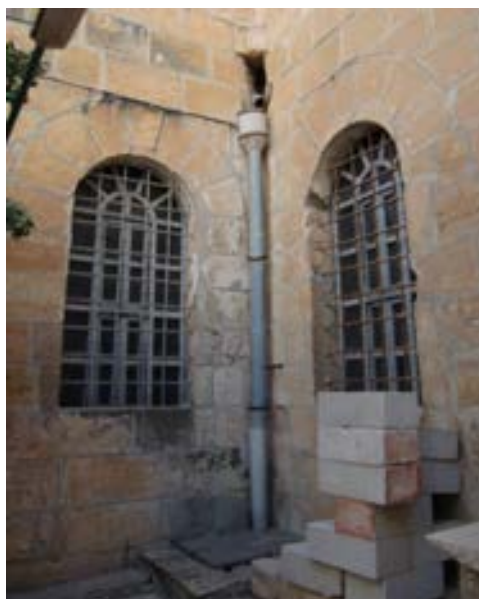
Figure 17: Pipe collecting the rainwater in 2A
