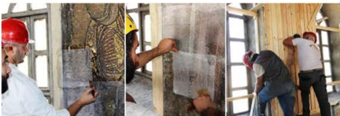
Figure 41: protection of the wall mosaics with cotton gauzes, non-woven fabric and boards
