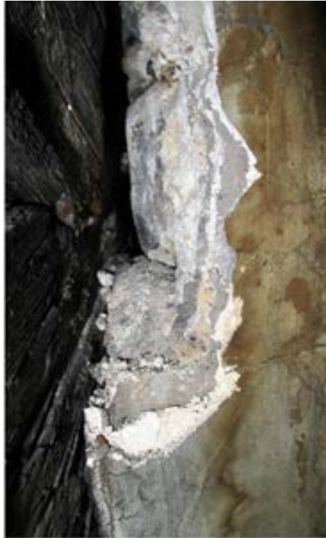
Figure 106: South wall of the nave – truss CN04, stratigraphy of the plasters
