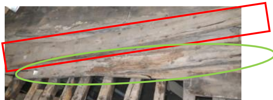
Figure 83: two adjacent boards evidencing a completely different extent of decay (both have been removed from the purlins): the board within the rectangle in red is in an excellent state of preservation and it can be kept without any additional treatment; the board within the oval in green has been attacked by fungi, and it needs to be partially or totally replaced (the decayed surface is >50% of the board surface).
