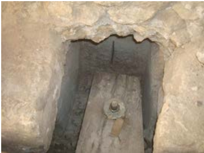
Figure 119: the original space around the truss head
