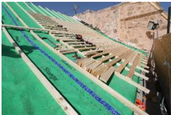
Figure 103: plywood; insulation layer (green), wooden laths and boards supporting the wool layer and the external lead sheets
