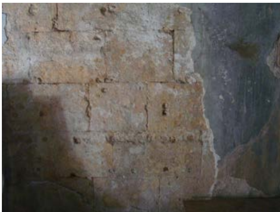
Figure 120: Holes hosting the metallic devices to hang the marble slabs on the walls
