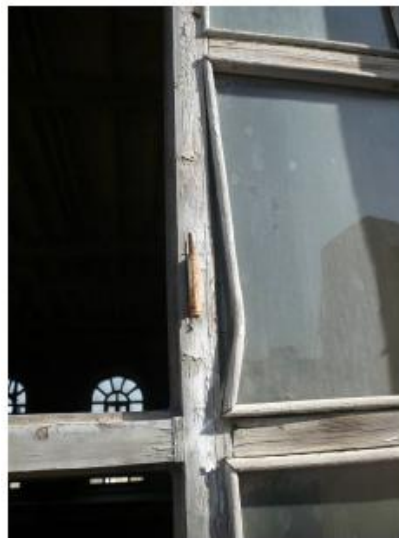
Figure 9: deformation of wood frame due to the weathering
