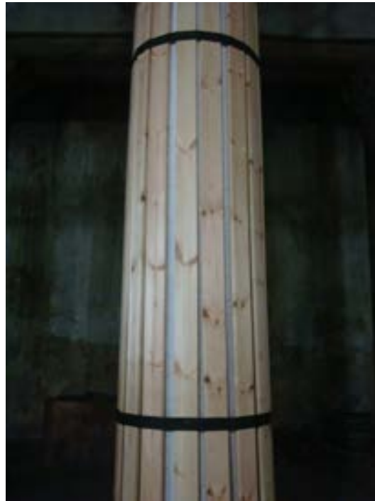
Figure 48: a detail of the protective system for the painted columns
