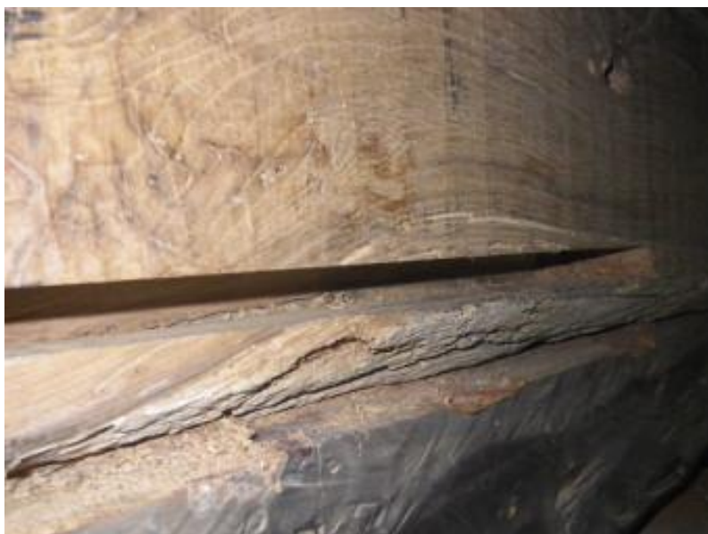
Figure 78: groove to host the steel bars and resin
