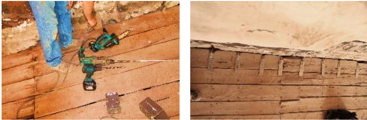
Figure 99 (from left to right): drilling a hole in the wall and insertion of resin, insertion of steel bar and connection steel plates-boards
