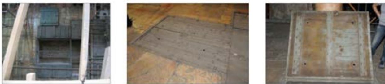
CHECKING OF WOODEN HATCHES, CHANGING OR STRENGTHENING THE WOODEN PLANKS COMPROMISED.
