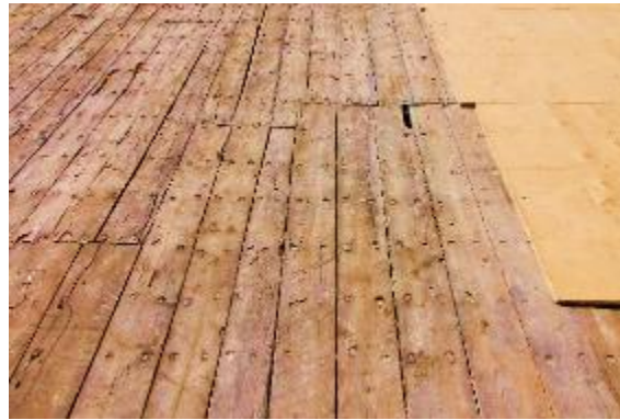
Figure 102: plywood connected directly with the existing boards
