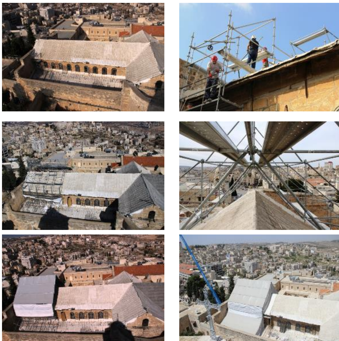
Figure 71: images of the temporary roof
