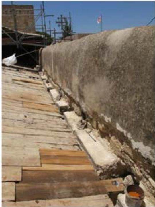
Figure 118: traces of the original drainage and rainwater collection system
