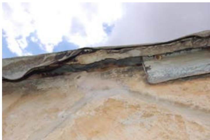
Figure 13: Lead and bitumen covering the roof
