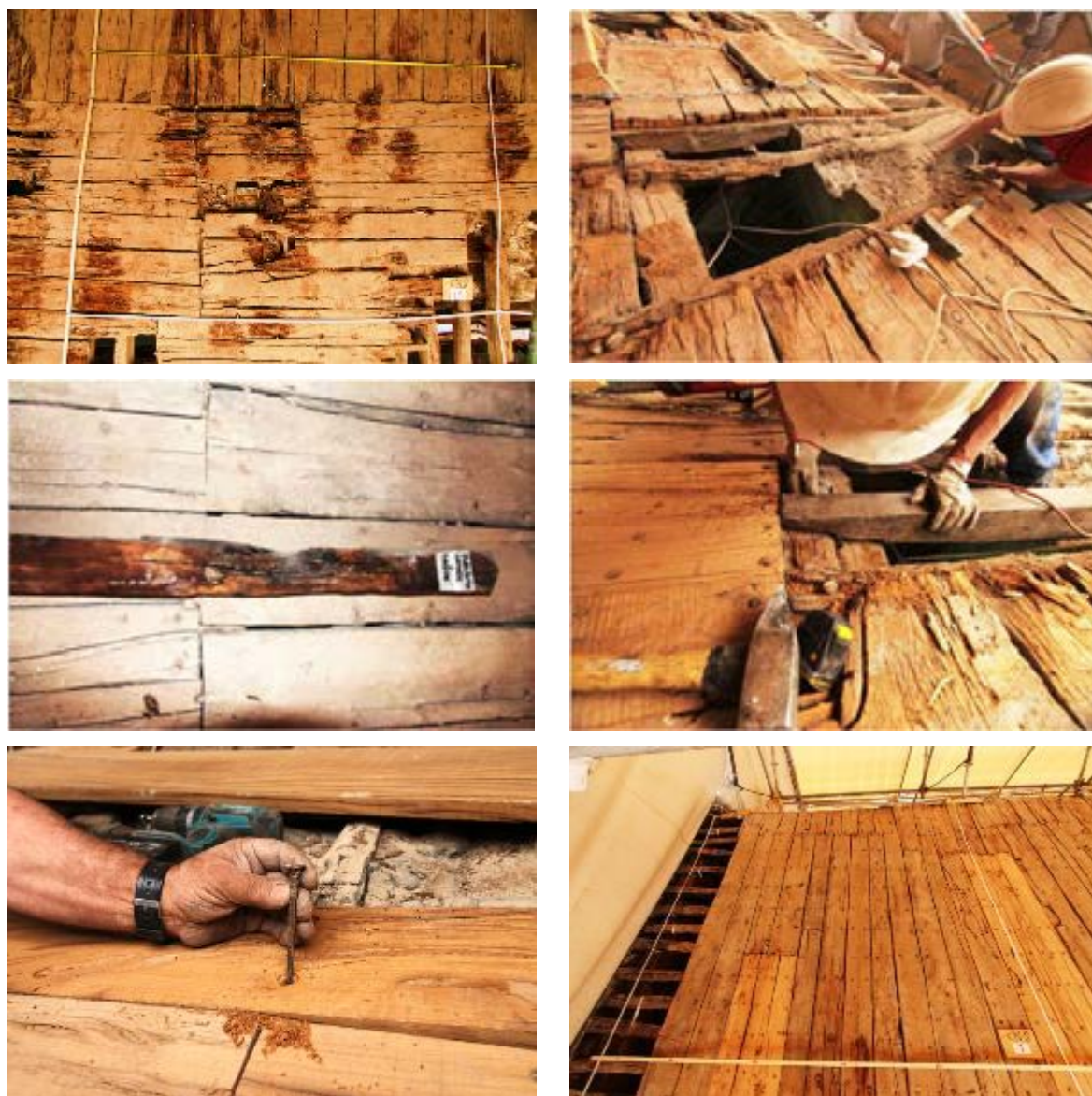
Figure 89 (from the top – from left to right): delimitation of the area with timber elements to be replaced, removal of purlins and boards, damaged purlins catalogued, replacement of a new purlin, replacement of the new board, the area at the end of the intervention
