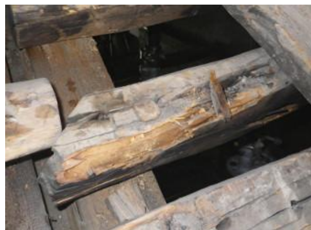
Figure 87: a purlin where a more accurate diagnostic analysis is needed to ascertain its effective static efficiency.
