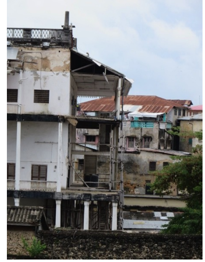
Collapsed porch - south eastern corner of the Beit al Ajab/House of Wonders.
