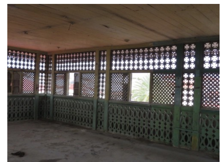
Grade I Tippu Tip House. Roof-top tea house with fine stick-and-fretwork screens.
