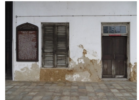
Main façade. Note weathering to walls.
