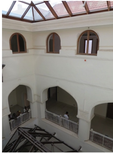
Enclosed courtyard, Mambo Msiige. The old first floor roof structure has been retained. New glazed roof over on raised parapet.
