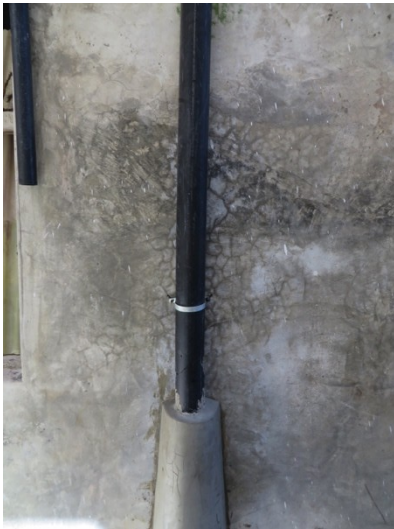
Renovation utilizing Portland cement. A detrimental practice - Kiponda.
