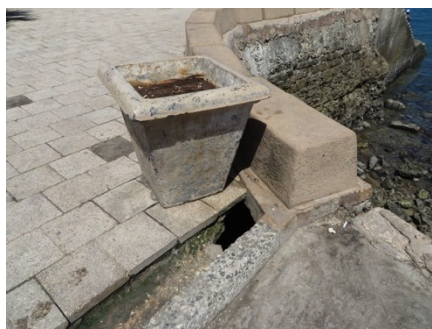
Mizingani Road, end of Forodhani Gardens sea wall. Here the sea has weakened the wall.
