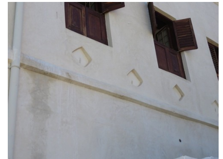
Remedial patrices inserted into façade of a renovated building at the Royal Tombs, Mizingani Road.
