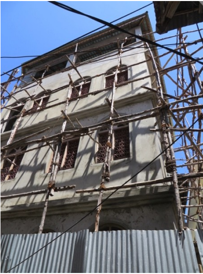
Renovation utilizing Portland cement. A detrimental practice - Malindi.
