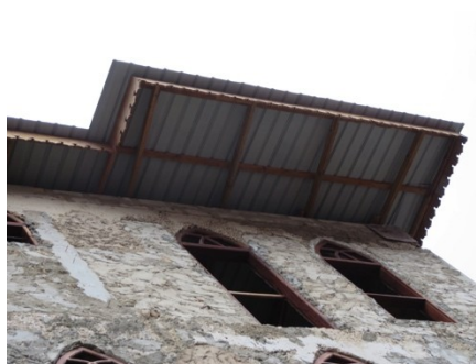
Incorrect material use (roofing) at restoration.
