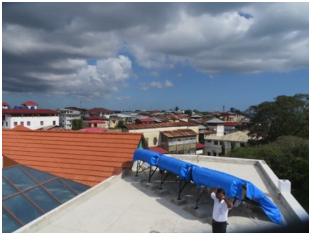
Roof top solar hot water installation - Mambo Msiige.
