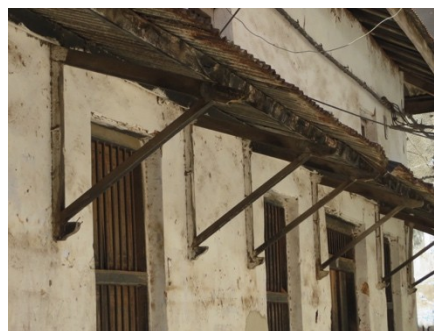
Typical cantilevered roof - Kiponda.
