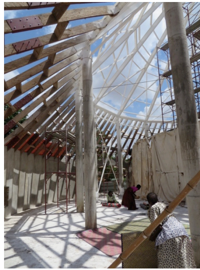
Mazibu Azaala Mpanga. Steel and timber construction.
