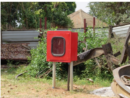
Temporary fire hydrant.
