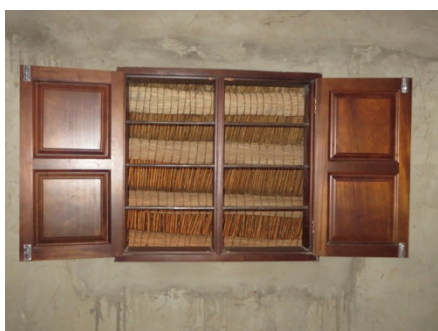
Teak windows in cement rendered concrete block walls, Gazimbye.
