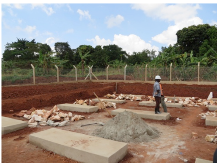
Installation of a solar photo-voltaic installation. Footings for the panels.
