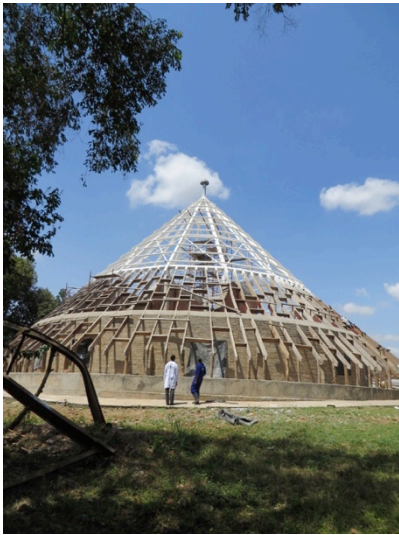
Reconstruction structure, Mazibu Azaala Mpanga with fire retardant
