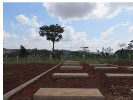
Footings for the Photo-voltaic panel installation.
