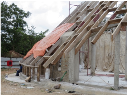
Reconstruction structure, Mazibu Azaala Mpanga. Eve detail.
