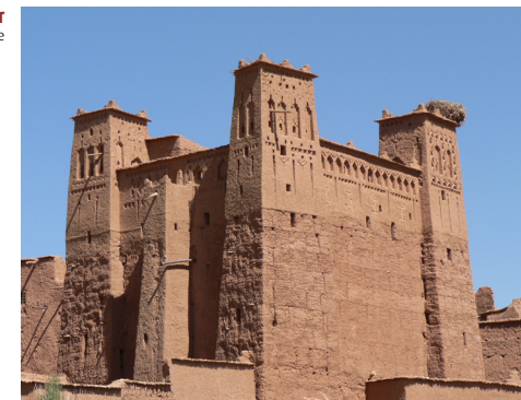
One of the fortified houses of the Ksar © Sébastien Moriset, CRAterre
