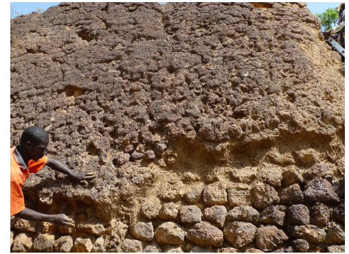
Conservation of earth plaster covering the laterite blocks © David Gandreau, CRAterre
