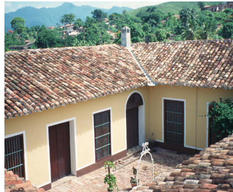
Patio of a house built in «mampuesto» (earth and rubble) © Wilfredo Carazas-Aedo, CRATerre
