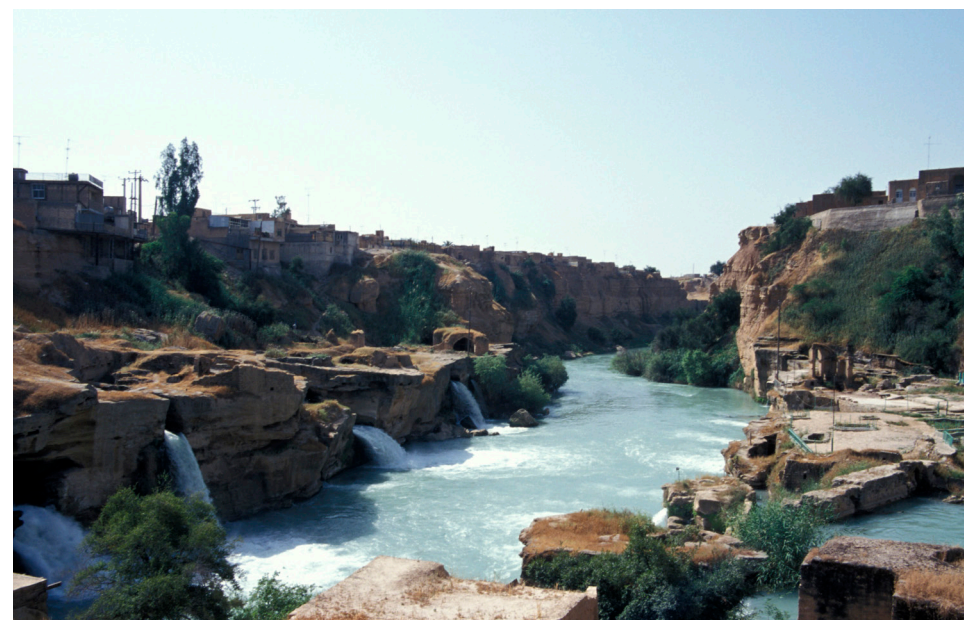
Historical hydraulic system of Shushtar, the water passes through underground canals and mills before cascading into the basin
