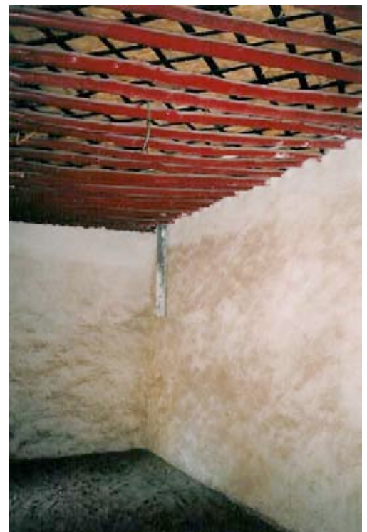
The Main Fortress (“Bahrain Fort”) Traditional Roofing System Used in Conservation (October 2003)
