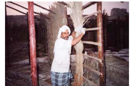
F11- P30- CONSERVATION OF THE TRADITIONAL BARASTAJ ON THE UPPER LEVEL OF THE MAIN FORTRESS ("BAHRAIN FORT") (DECEMBER 2003)
