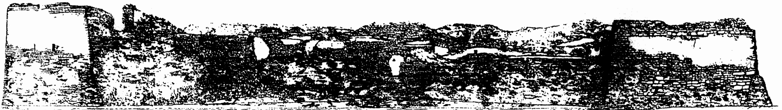
West Elevation before restoration
