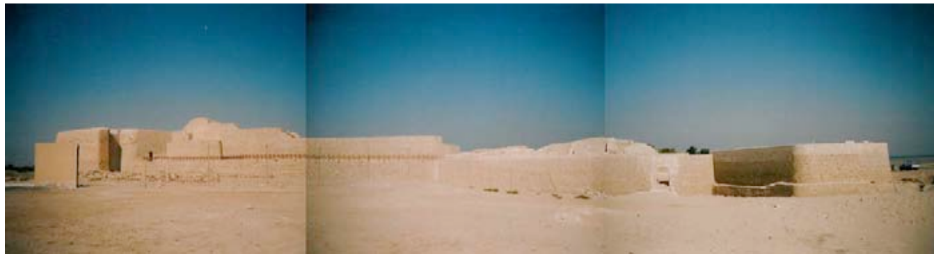
General Panoramic View of Site, towards the West (October 2003)
