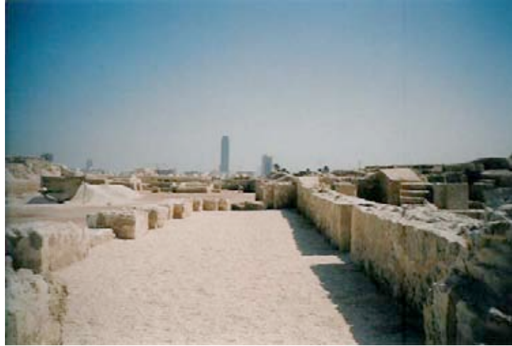
The Main Fortress (“Bahrain Fort”) – First Enclosure – Madbasa covered for protection (October 2003)
