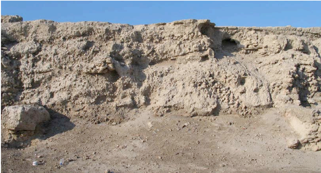
Section at the South of Islamic sector, facing South (approx. height : 4 m)
