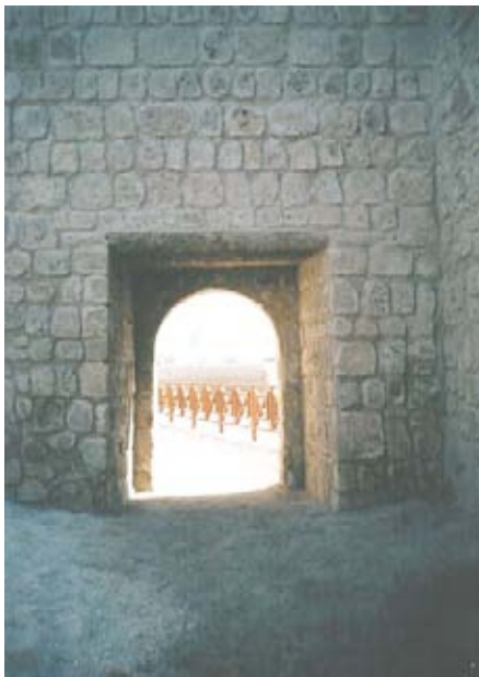
The Main Fortress (‘Bahrain Fort’) Location with possible excessive conservation (October 2003).
