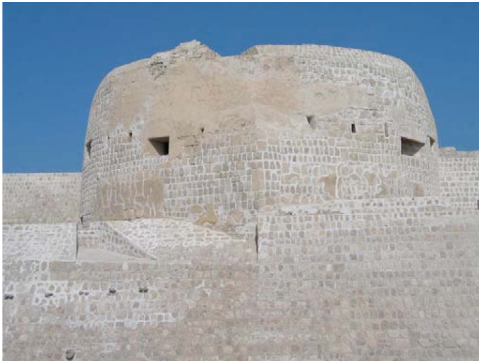
Figure 19 – The « Spur Tower » on the south side of the Main Fortress (« Bahrain Fort »)
