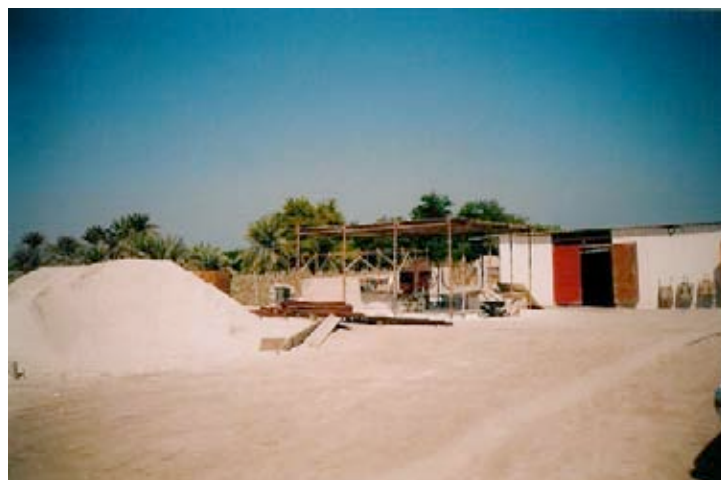
Workers Shed near the Main Fortress (“Bahrain Fort”) (October 2003)
