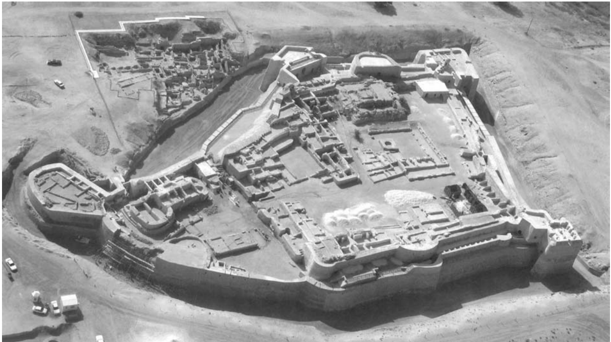
Aerial view towards the south of Bahrain Fort
