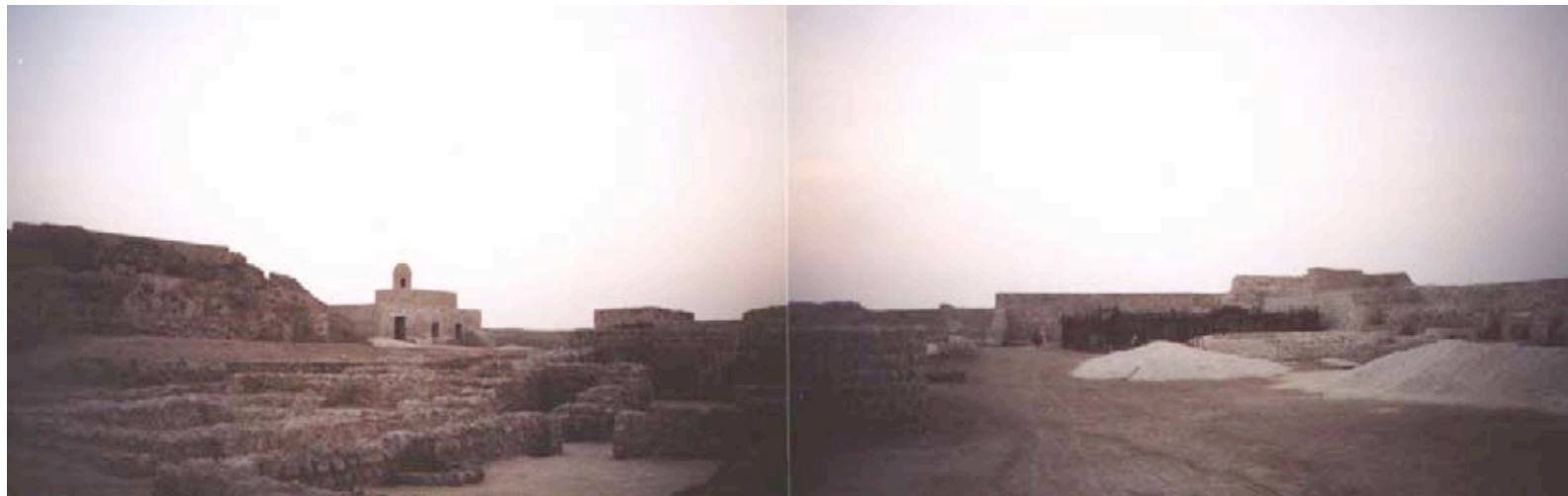
Panoramic View on the Upper Level of the Main Fortress (“Bahrain Fort”), toward the West (December 2003)
