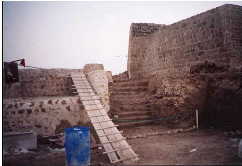
Current Conservation / Consolidation works at the Main Fortress (“Bahrain Fort”) (December 2003)
