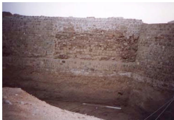
The Main Fortress (“Bahrain Fort”). Original wall layer from second and third stages (December 2003)
