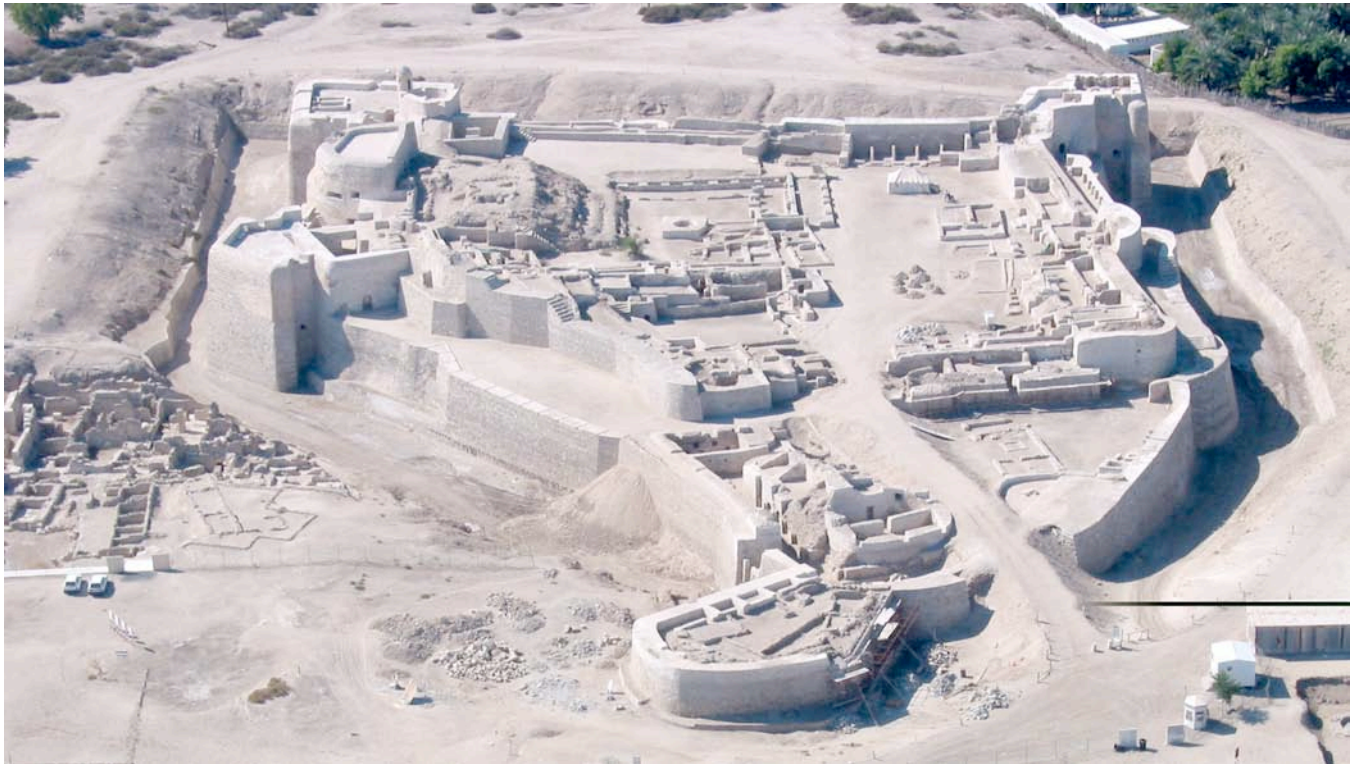
Figure 12 – The Main Fortress (« Bahrain Fort ») under restoration in 2002, towards the west
