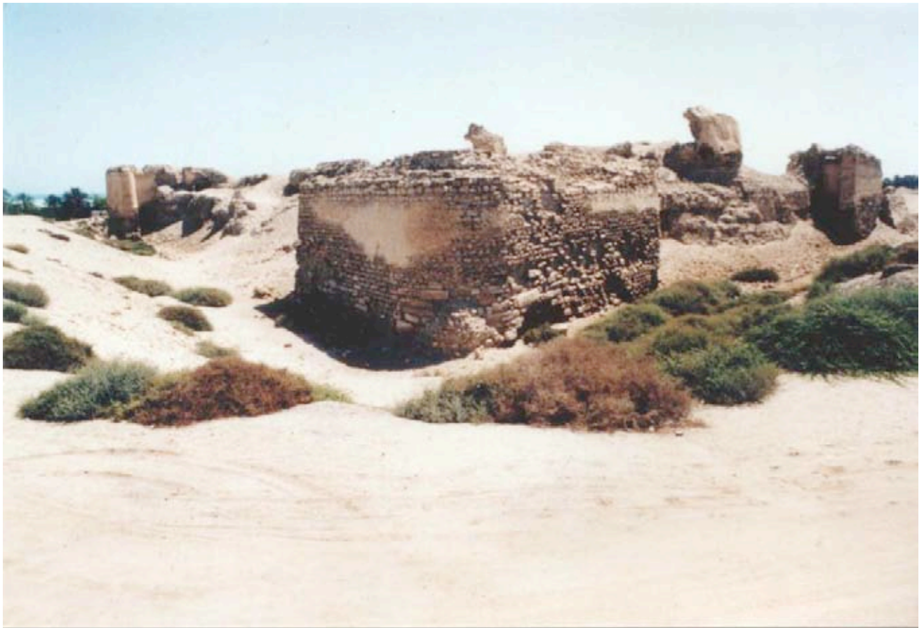
Figure 5 – The Main Fortress (« Bahrain Fort ») in the 1980s, before its restoration
