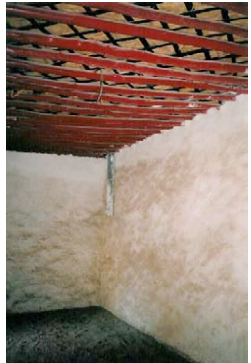
The Main Fortress (“Bahrain Fort”) Traditional Roofing System Used in Conservation (October 2003)
