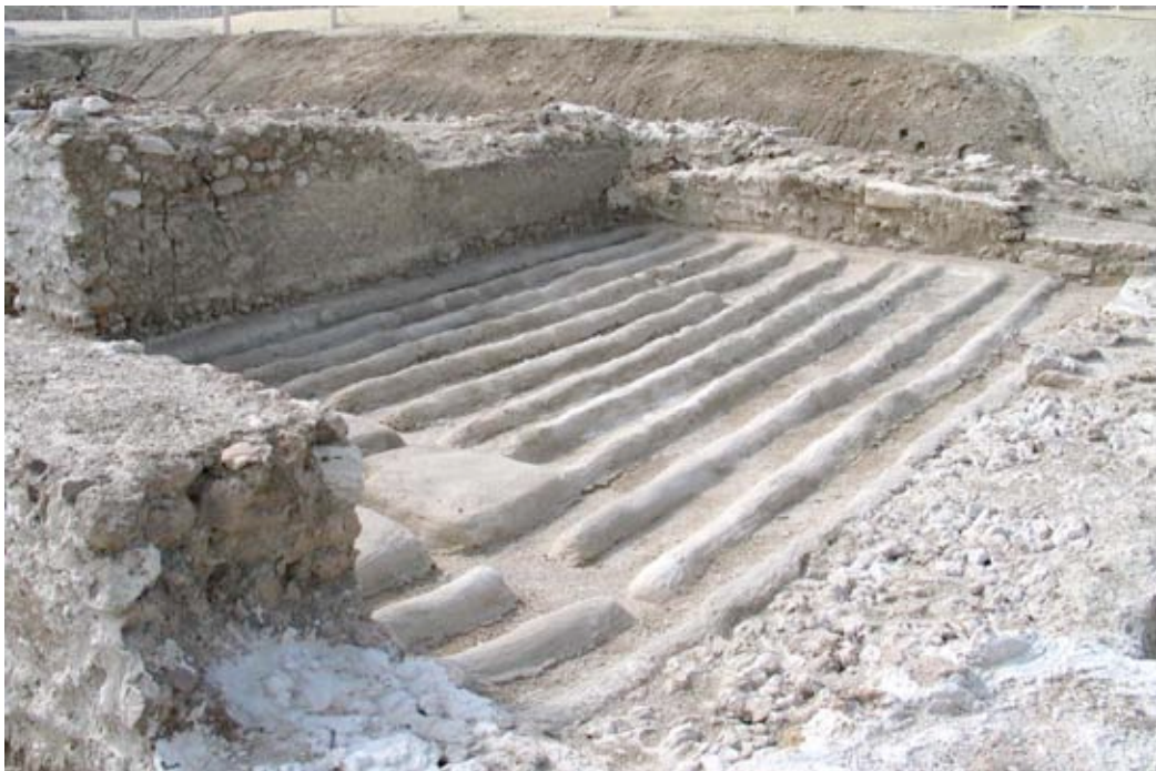
E — One of the madbasa (date-incubator), with renovated coating (January 2005)
