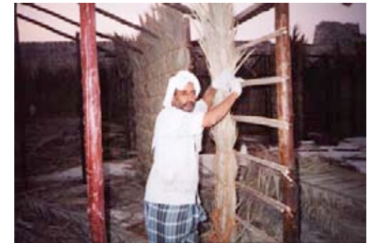
F11- P30- CONSERVATION OF THE TRADITIONAL BARASTAJ ON THE UPPER LEVEL OF THE MAIN FORTRESS ("BAHRAIN FORT") (DECEMBER 2003)
