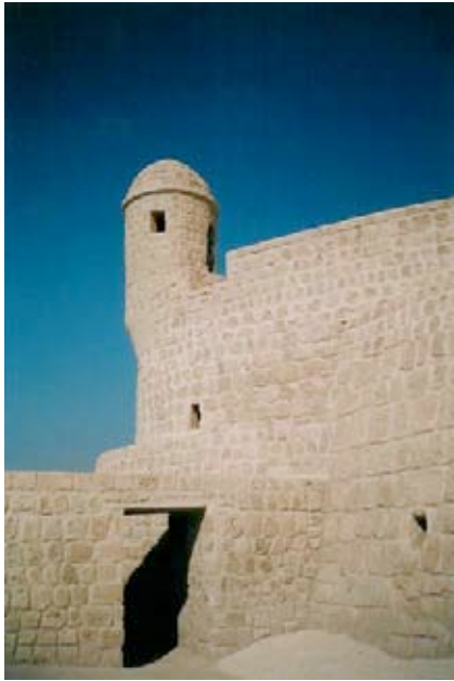
The Main Fortress (‘Bahrain Fort’) – First Enclosure Conservation (October 2003)
