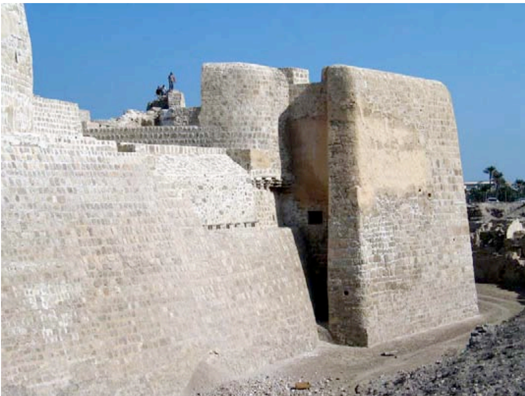
B – The southeastern bastion, towards East
