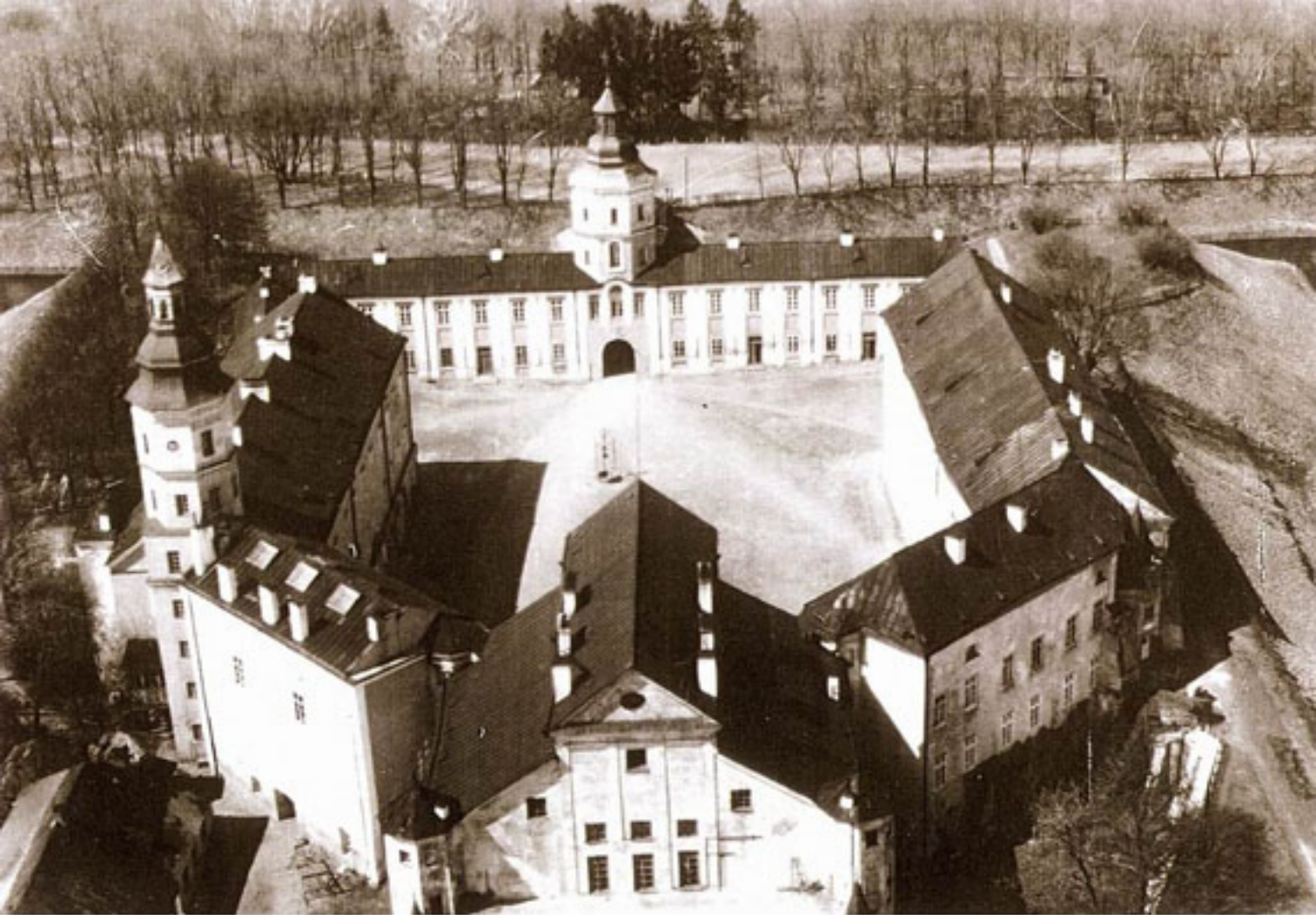
Castle in Nesvizh. Aerial view from the east
