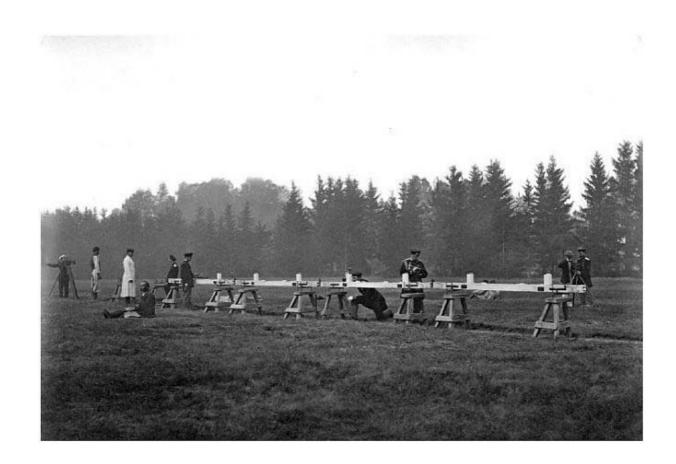
**Figure 12.** The measurement of baseline, (Picture is a courtesy of Museum of Pulkova)
