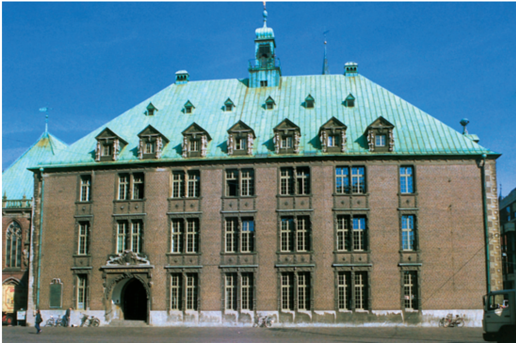
New Town Hall, main façade facing the cathedral and view from Domshof
