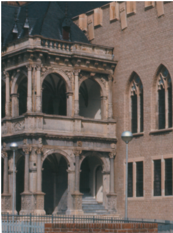
The façade of the Town Hall of Cologne
