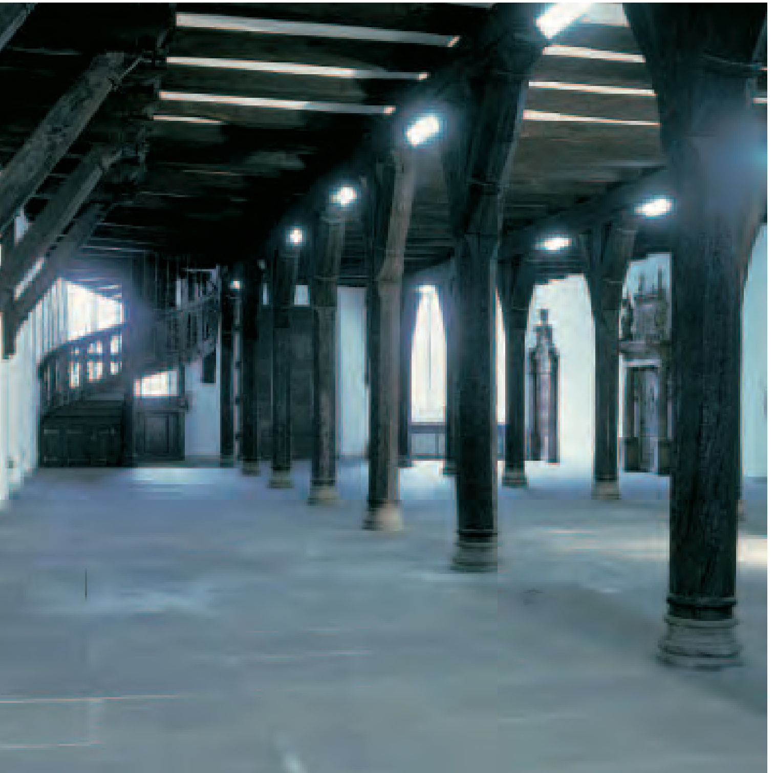
Old Town Hall, Lower Hall
