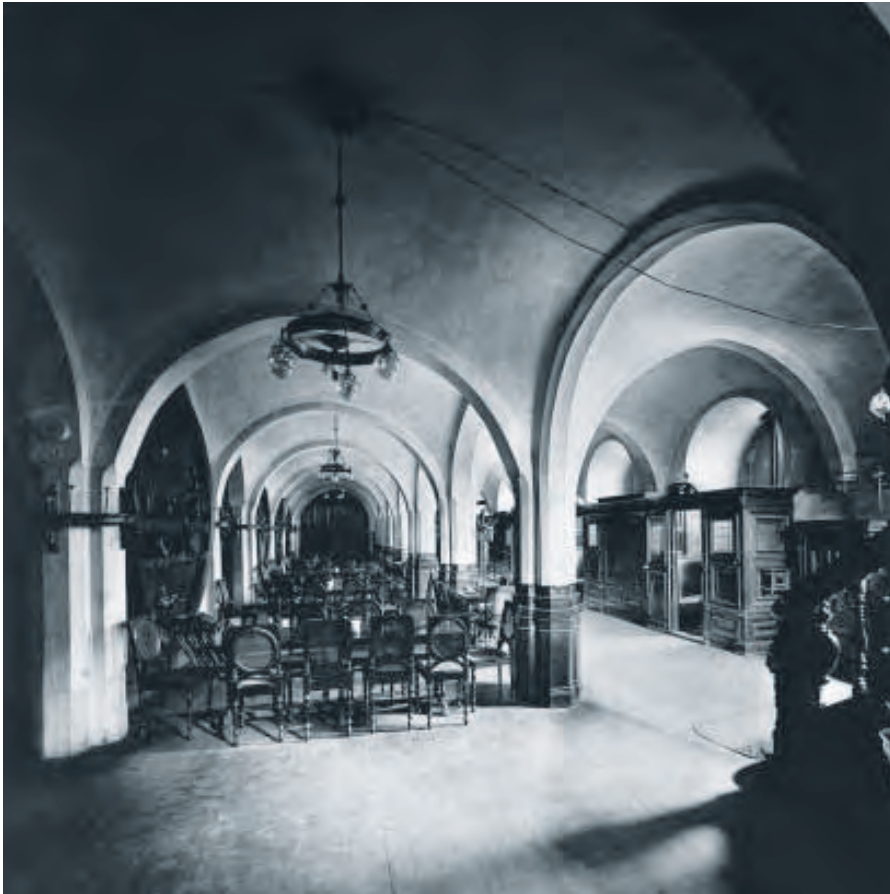
Cellar, overall view of the main cellar, looking eastward
