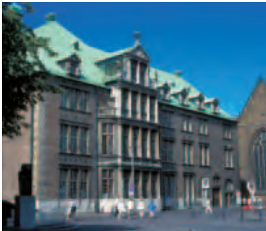
New Town Hall, south front adjoining Old Town Hall, main front facing the cathedral and view from Domshof
