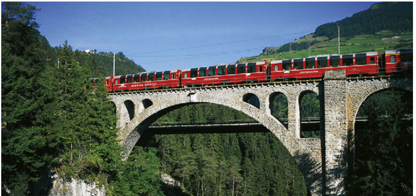
Albula line > The Solis Viaduct, the bridge with the greatest span on the Albula line. P. Donatsch
