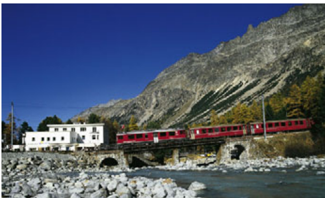
Bernina line > Morteratsch station and the steel bridge across the Ova da Morteratsch. A. Henkel
