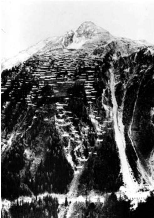
Muot avalanche baffle > Photograph 1905. Rhaetian Railway
