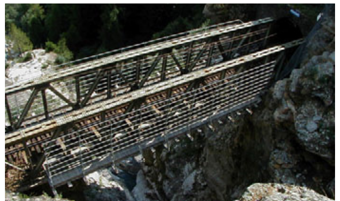
Bernina line > The lower Cavagliasco Bridge. The original stonework bridge had to be replaced by an army emergency bridge in 2002 due to earth movements. Rhaetian Railway
