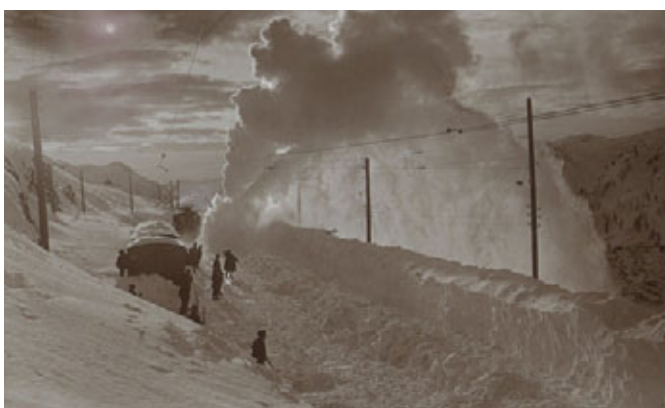
Bernina line > Historical photograph of snow clearance at the Alp Grüm station. Rhaetian Railway
