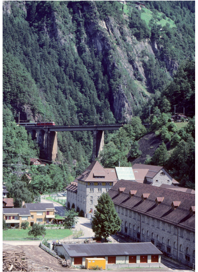
Gotthard Railway > North ramp at Amsteg Swiss Federal Railways power station. Photograph 1988. H.P. Bärtschi
