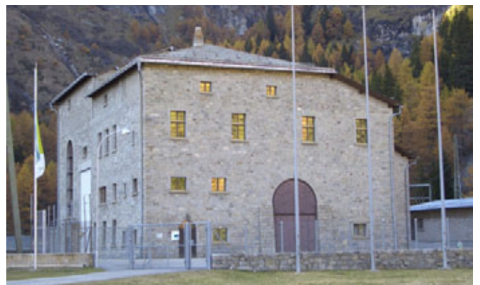
Cavaglia power station > The building complex, reflecting the lines of a house in 'Engadin style' was also designed by Nicolaus Hartmann the Younger. L. Dosch
