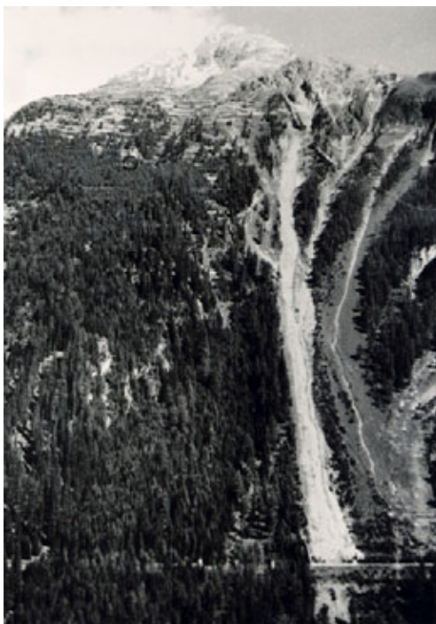
Muot avalanche baffle > Photograph 1957. Rhaetian Railway
