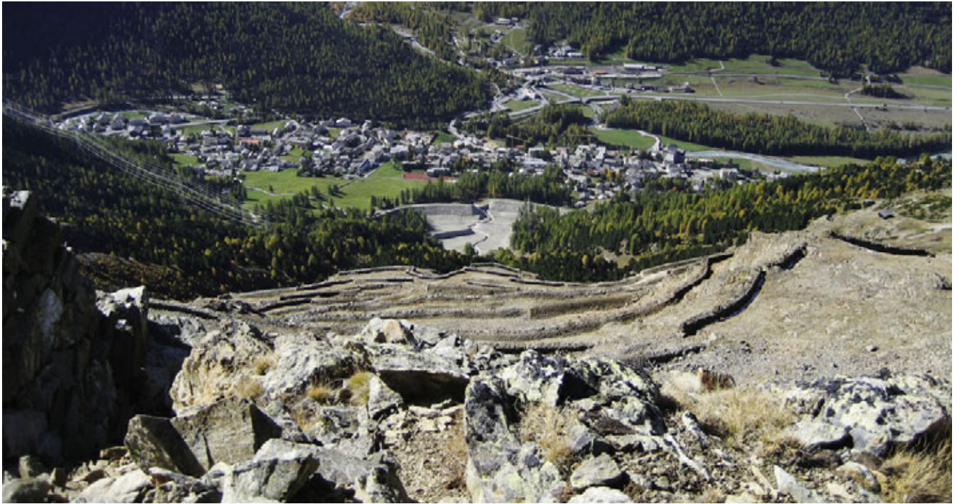
Pontresina > Two protective embankments have been built above the village; the thawing of the permafrost made this measure necessary. E. Süsskind
