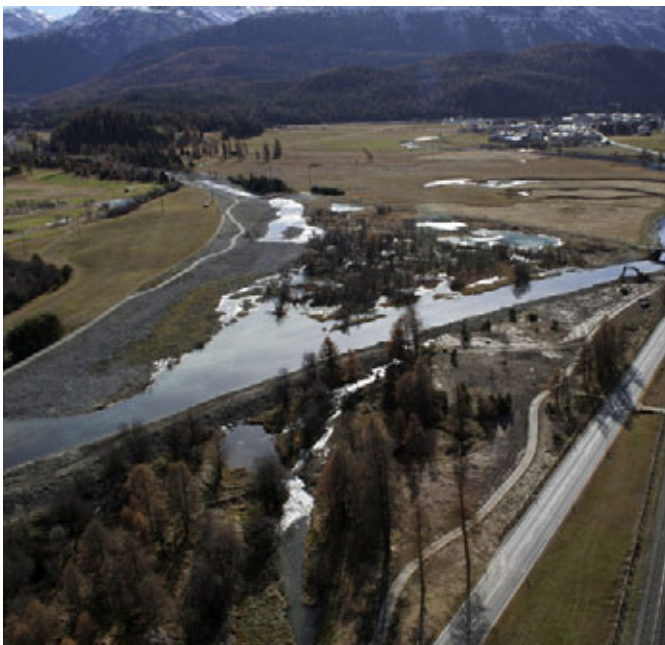
Samedan > Renaturalisation of the river has created natural habitats. Tiefbauamt Graubünden, Chur
