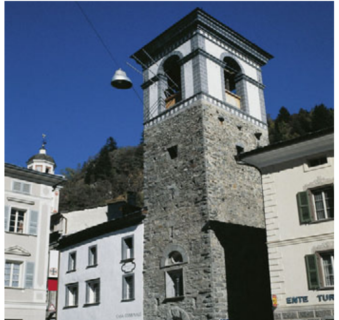
Poschiavo > Torre di Municipio. Built as a defence tower for the episcopal bailiff in the first half of the 13th century. Later the seat of the Olgiati family. Converted for use as the Rathaus in the mid 16th century. The belfry was added in 1651. Denkmalpflege Graubünden, Chur
