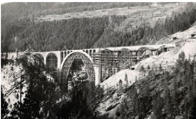
Davos–Filisur line > Wiesen Viaduct. The imposing framework was constructed by the legendary Richard Coray. Taken in 1908. Rhaetian Railway
