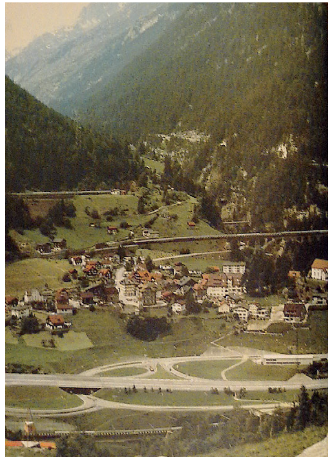
Gotthard Railway > The transport landscape around Wassen: 19th century railtrack with loops at three different levels; late 20th century motorway. Photograph about 1980. Illustration from: EGGERMANN ANTON [et al.]: Die Bahn durch den Gotthard , Zurich 1981.
