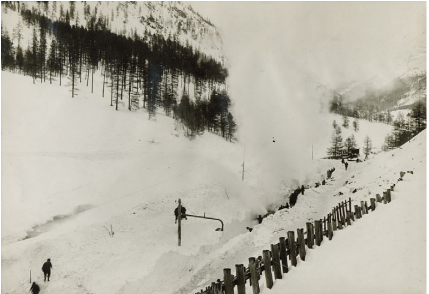
Albula line > Crasta Mora avalanche 23.12.1919. The top layer of avalanche snow had to be shovelled away before the steam snow blower could start work. Rhaetian Railway
