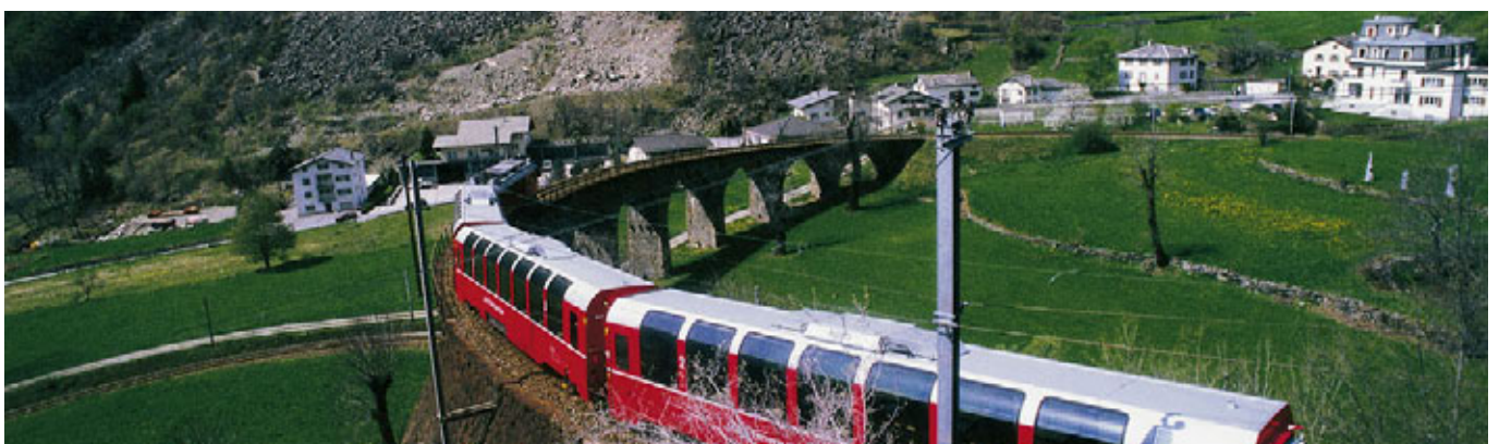
Bernina line > The Brusio circular Viaduct describes a quarter circle and has nine openings each with a diameter of 10 m in a curve of 70 m radius with a gradient of 70 ‰. P. Donatsch
