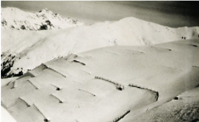
Albula line > The avalanche walls and snow catchers above Muot are almost snowed under. Rhaetian Railway
