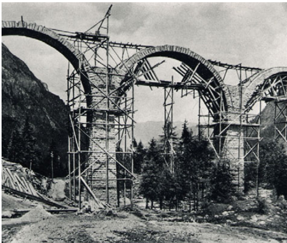
Albula line > The Albula Viaduct III ⑥, under construction, 1902. Rhaetian Railway
