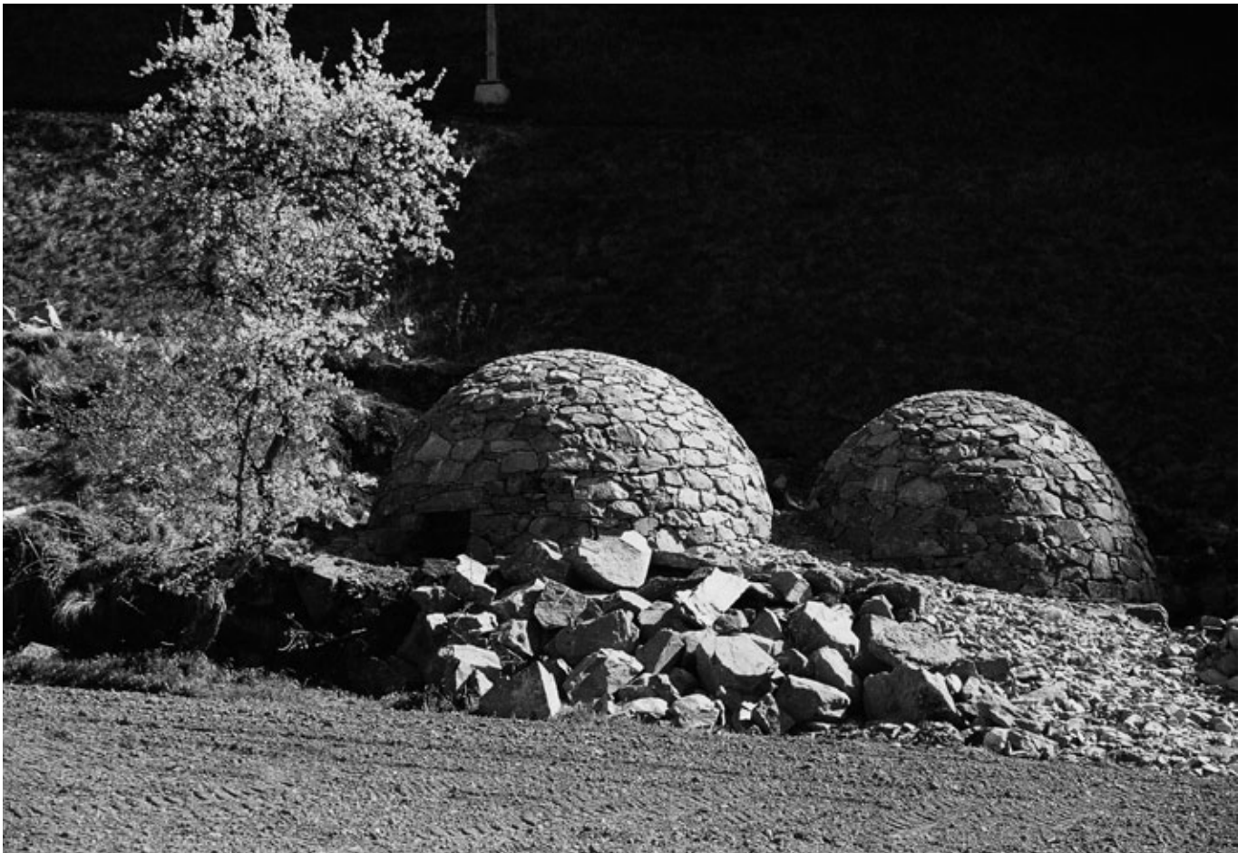
Brusio > A “crott” or “scéle”, an air cooled domed cellar below the railway embankment. D. Giovanoli
