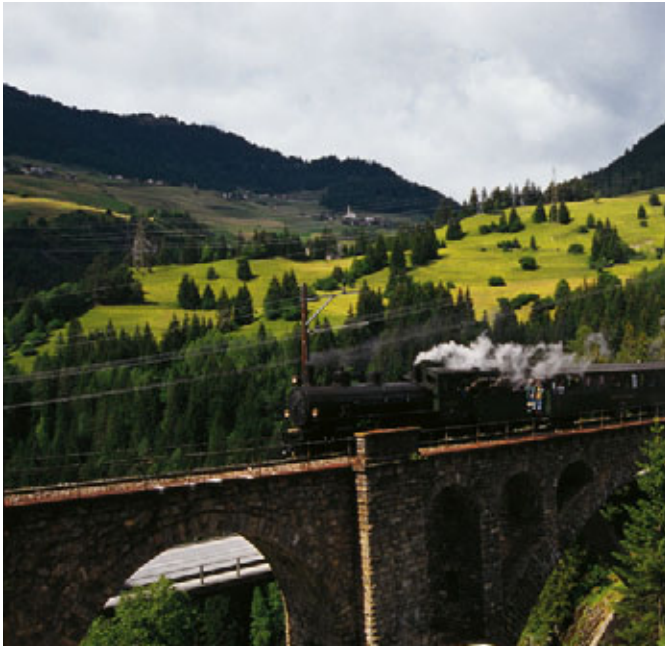
Schin gorge > Solis Viaduct on the Albul line, behind it the dry meadows and the terrace villages of Zorten, Lain and Muldain. Foto Geiger
