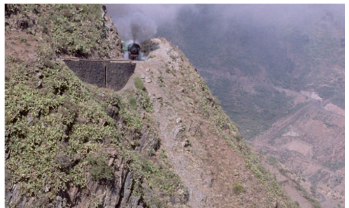
Eritrea Railway > Alignment at Embatalla. Photograph 2004. H.P. Bärtschi
