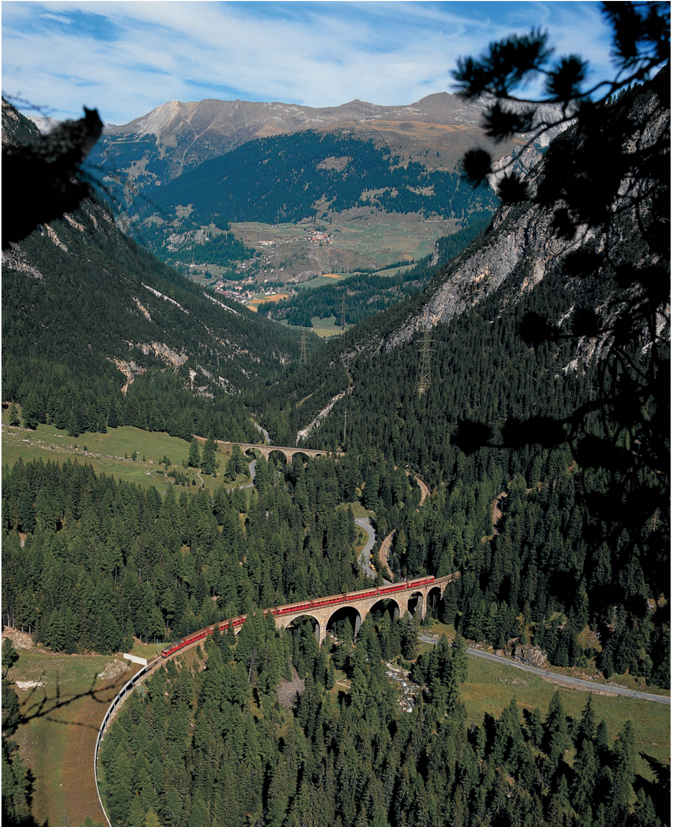
Albula line > The steep climb between Bergün/Bravuogn and Preda called for a complicated alignment with numerous engineering structures. A Rhaetian Railway passenger train crossing the Albula Viaduct III. Foto Geiger
