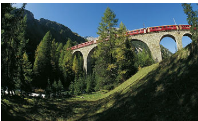
Albula line > The Albula Viaduct III, the bridge with the second largest cubature on the Albula line. Foto Geiger
