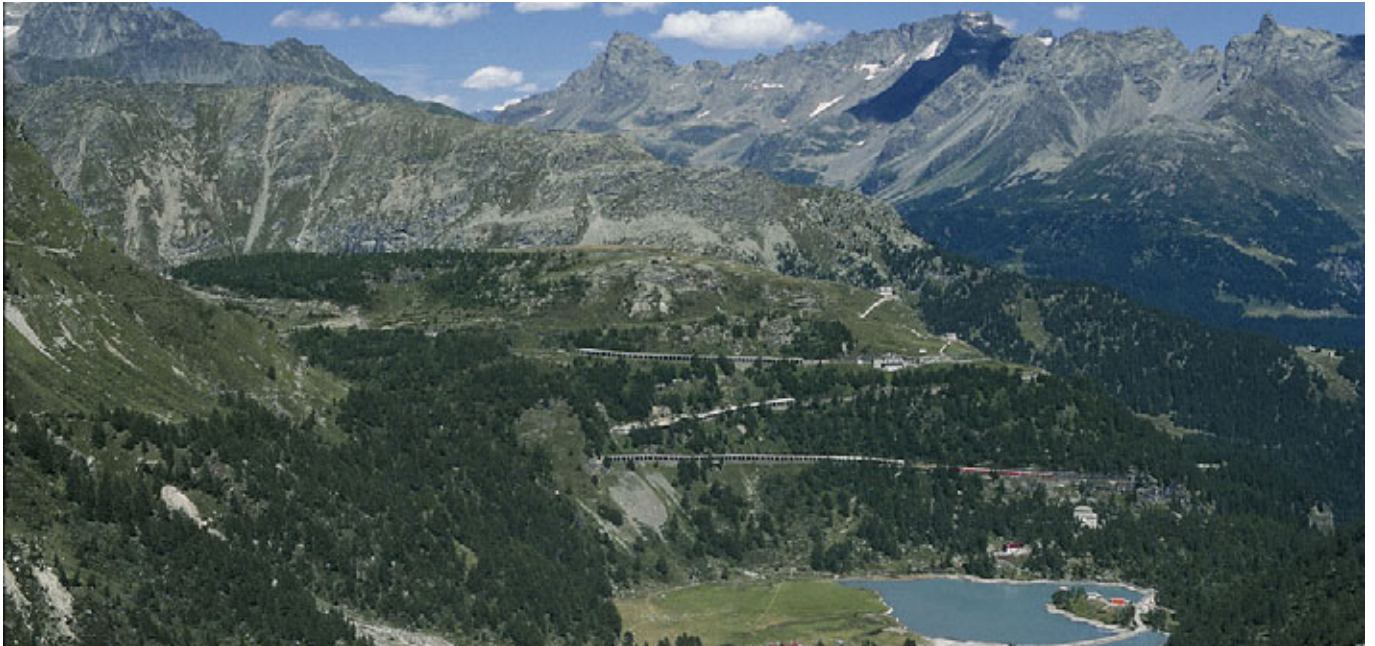
Bernina line > The layout of the line as it climbs Alp Grüm is more reminiscent of the zigzags of a pass road than a railway track. T. Keller
