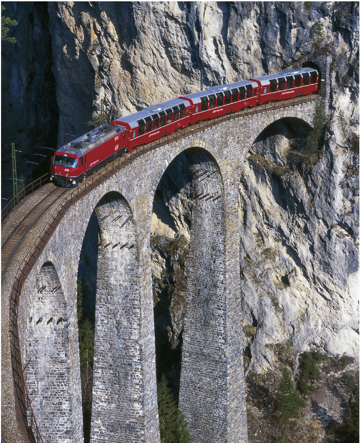
Albula line > The Rhaetian Railway Bernina Express on the Landwasser Viaduct near Filisur. P. Donatsch / Rhaetian Railway
