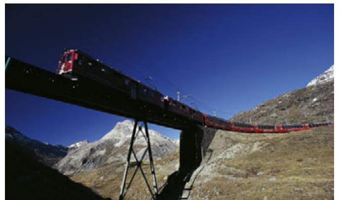
Bernina line > The upper bridge over the Bernina stream with stonework abutments, simple girders and hinged columns. T. Keller
