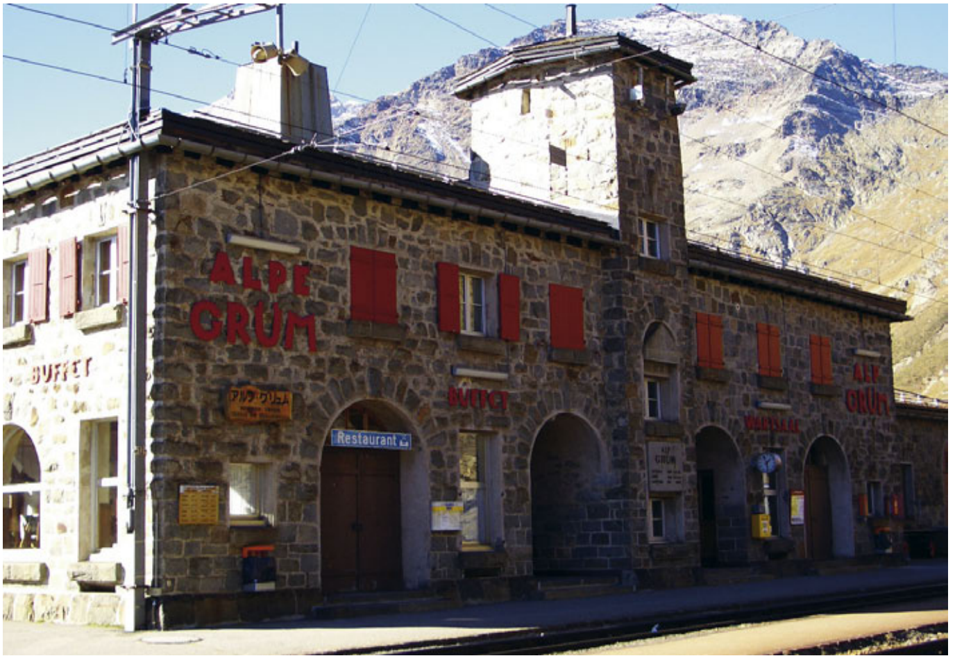
Bernina line > Alp Grüm reception building and guest house, 1923. L. Dosch
