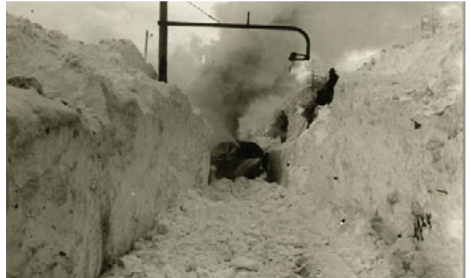
Albula line > The Crasta Mora avalanche buried the track and tore down the catenary in Val Bever 23.12. 1919. A steam snow blower removing the compact snow brought down by the avalanche. Rhaetian Railway
