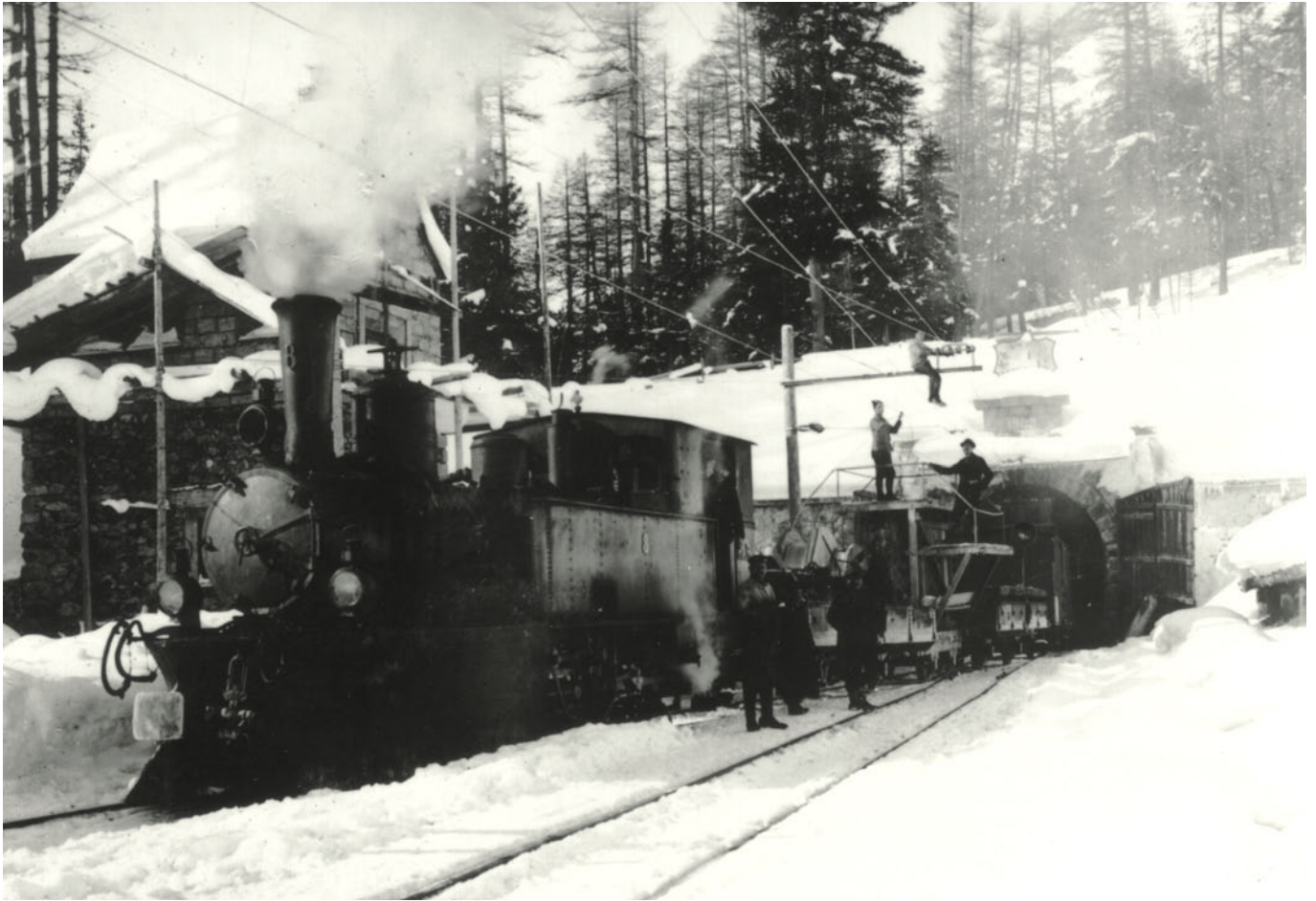
Electrification of the Albula line > Spinas portal of the Albula tunnel, G 3/4 steam engine in front of a Kummeler & Matter assembly train. Archives Hermann Kummeler)
