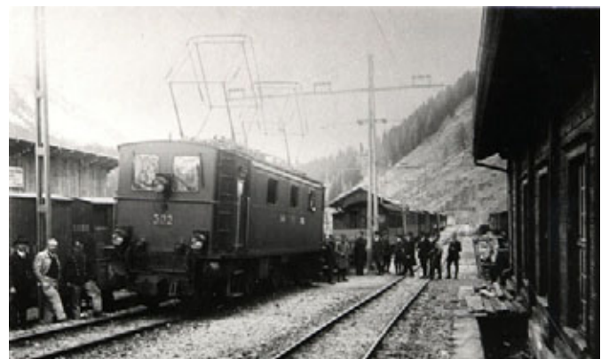
Electrification of the Albula line > The trial-run train in Bergün/Bravuogn station. Photograph about 1919. Collection G. Brüngger
