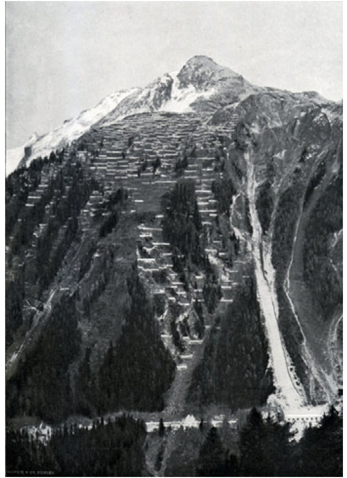
Albula line > When it was built, the largest avalanche baffle in Switzerland: Muot. Bottom right the Chanaletta gallery, 1907. Rhaetian Railway
