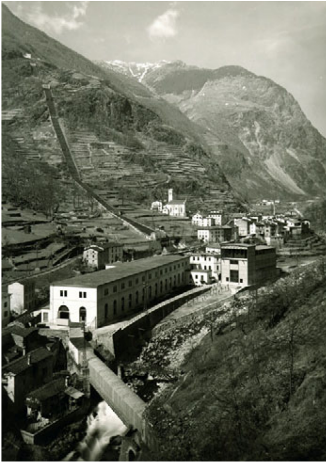
Campocologno > Six penstocks of the largest storage power station in Europe of the time ran from the Scala gallery to the Campocologno station. Photograph before 1933. A. Steiner/Rhaetian Railway
