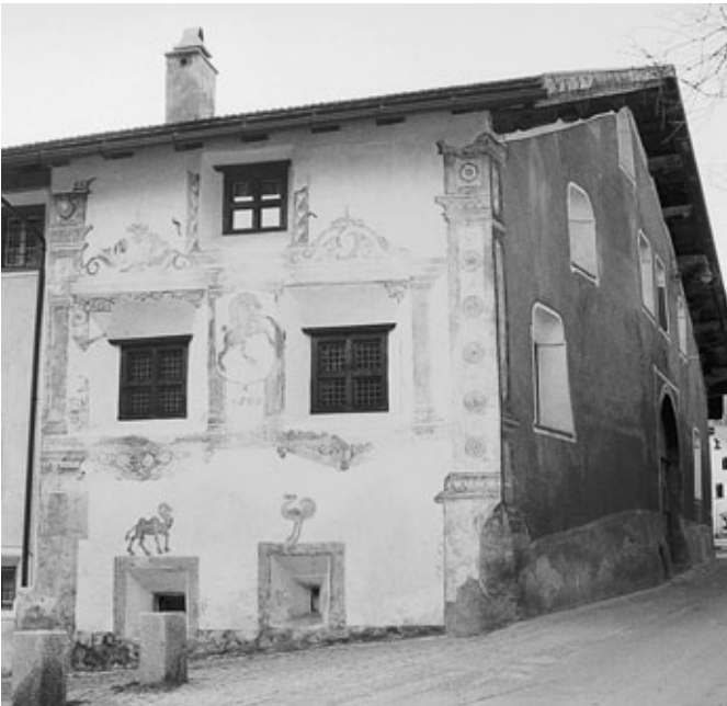
Filisur > Engadin style house with façade murals by Hans Ardüser, the 'peripatetic' master from Graubünden, dated 1595. Denkmalpflege Graubünden, Chur
