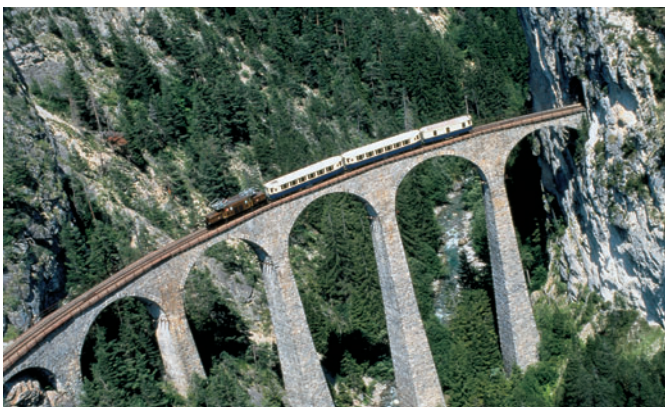
Albula line > A historical train composition, authentic in every detail, on the 100 year old Landwasser Viaduct. P. Donatsch / Rhaetian Railway
