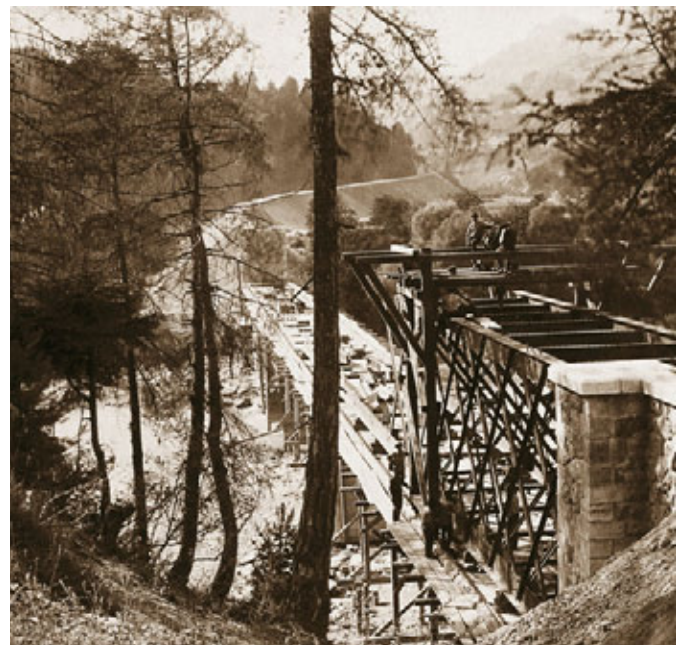
Chur–Thusis line > Construction of the steel bridge across the Hinterrhein at Reichenau. Taken in 1885. Rhaetian Railway
