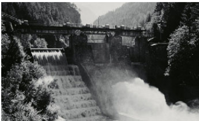
Nisellas > Running off floodwater at the Nisellas wier gate. Photograph from before 1980. Elektrizitätswerk der Stadt Zürich
