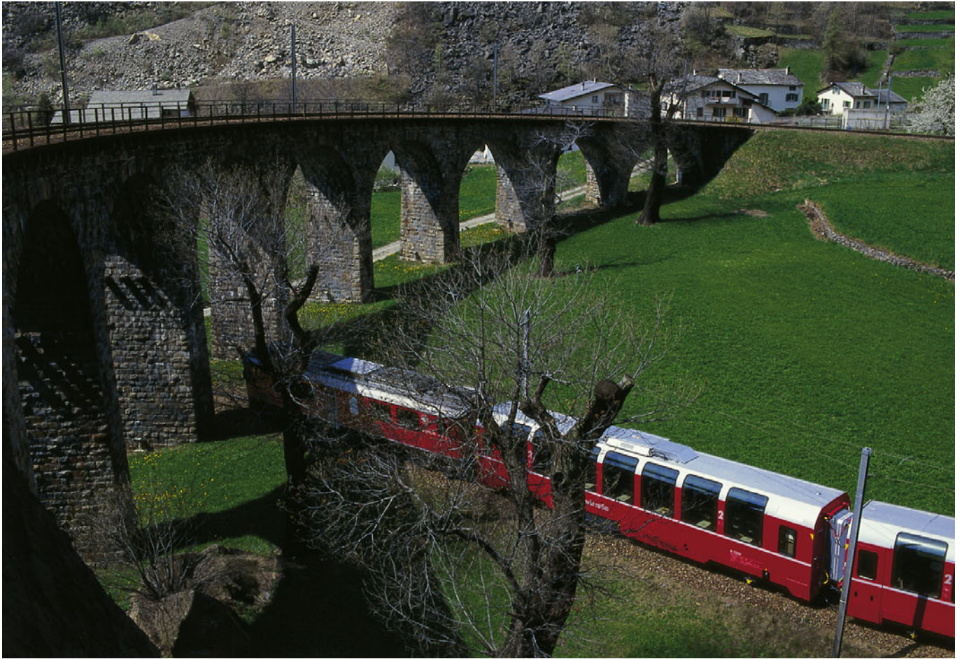
Bernina line > The Bernina Express on the Brusio circular viaduct which climbs on the same principle as a helical tunnel. P. Donatsch
