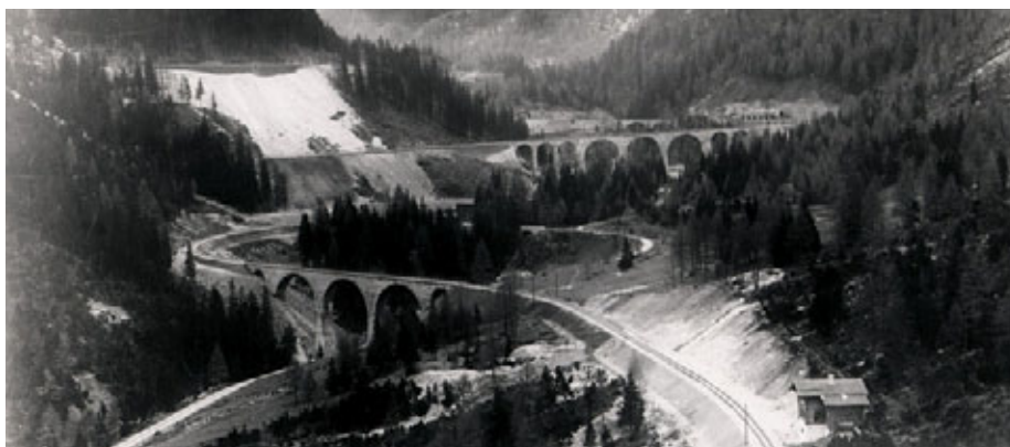
Albula line > The Albula Viaducts II ④ (foreground) and III ⑥ (behind) shortly after completion. Bottom right the Val Rots linesman's hut. Photographed in November 1902. Rhaetian Railway
