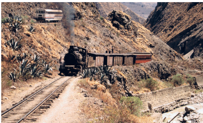
Guayaquil & Quito Railway > Zigzag alignment at the Devil's Nose. Photograph 1990. H.P. Bärtschi
