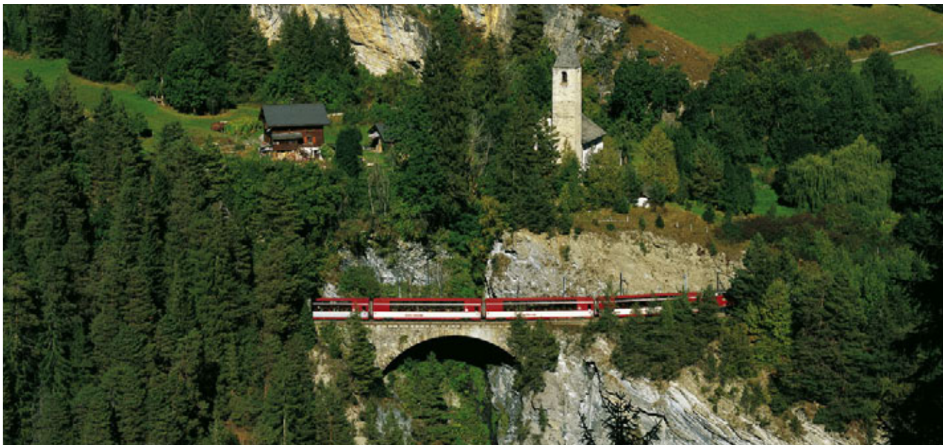
Albula line > The 27 m Mistail Viaduct is located immediately below the Carolingian church of St. Peter in Mistail at the upper end of the Schin gorge. B. Studer
