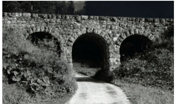
Albula line > Three arch overpass at Bergün. J. Conzett
