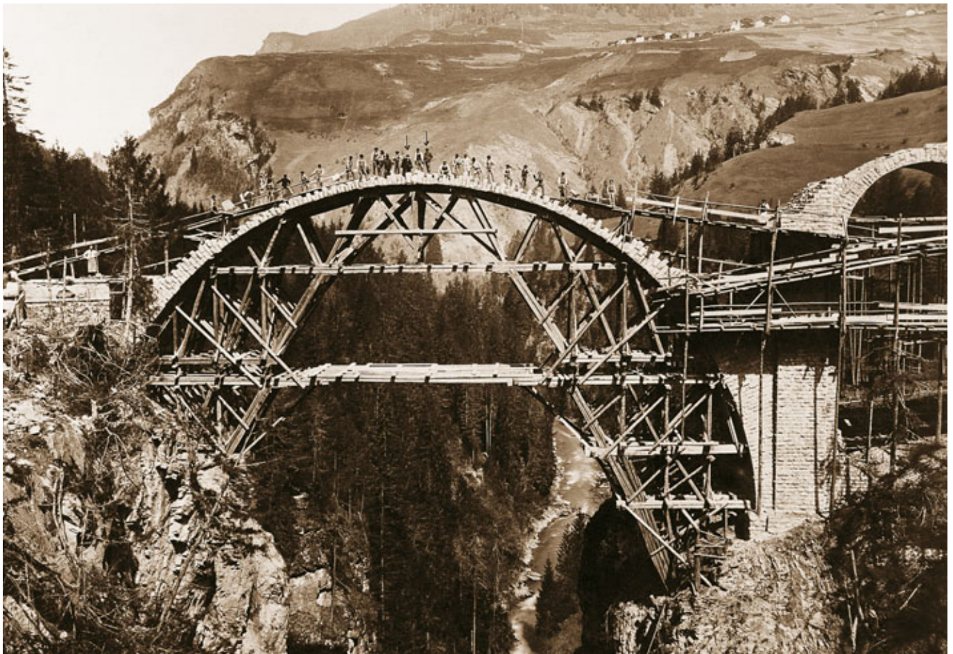
Albula line > The 42 m span of the Solis Viaduct under construction. Rhaetian Railway
