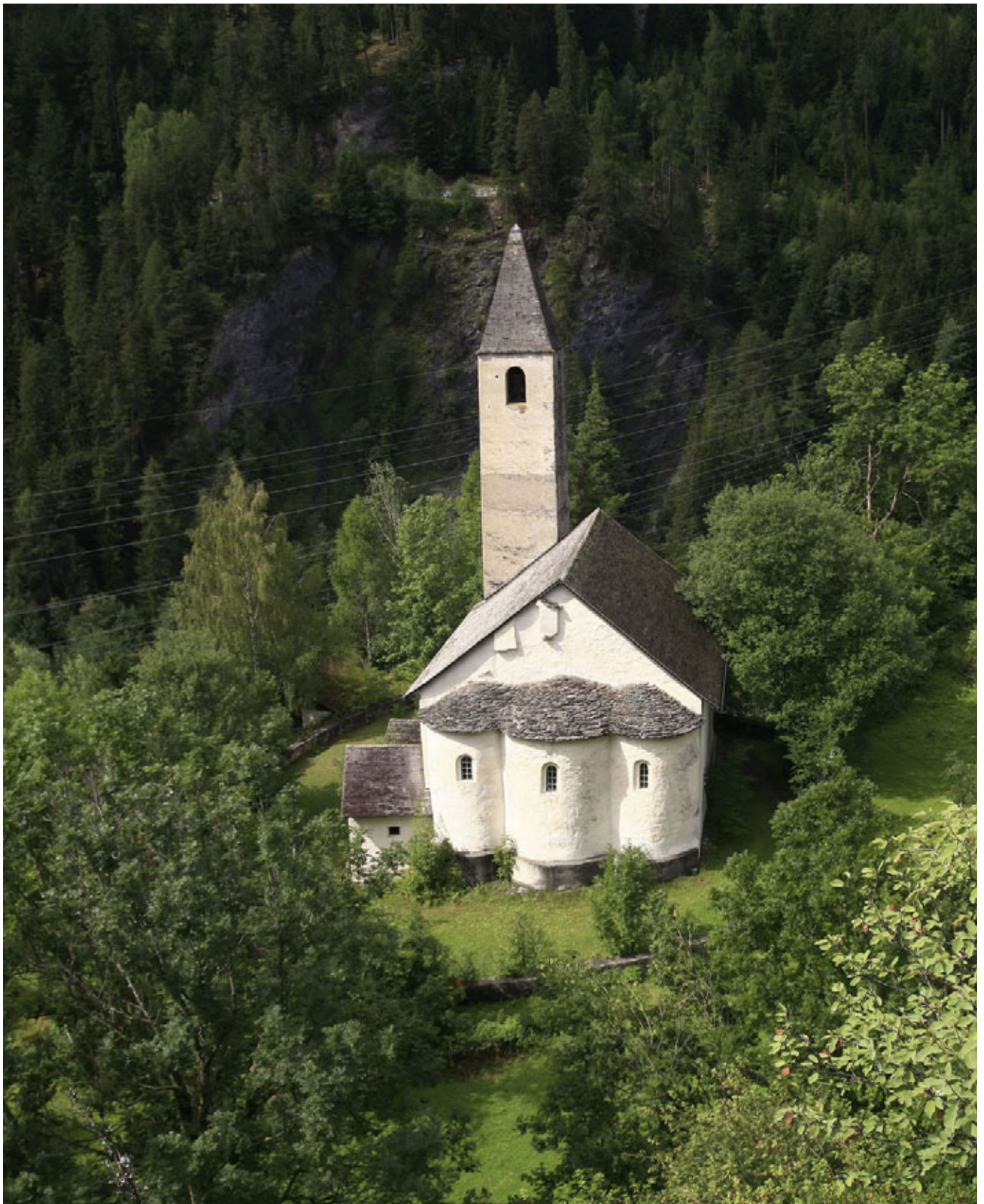
Alvaschein-Mistail > The Carolingian church of St. Peter with the characteristic three-apse ground plan. The former stonework bell yoke can still be recognised in the east gable, which was raised at a later date (the tower dates from the early 14th century). E. Süsskind
