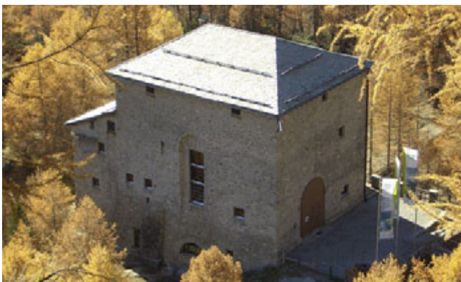
Palü power station > The tower-shaped machine house, designed by the architect Nicolaus Hartmann the Younger is reminiscent of the weirs built in the Middle Ages. L. Dosch
