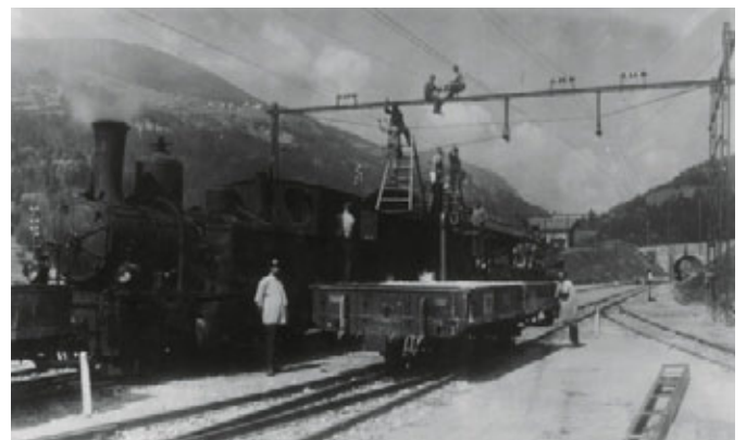
Electrification of the Albula line > Tiefencastel station: photograph 1919. Archives Hermann Kummeler
