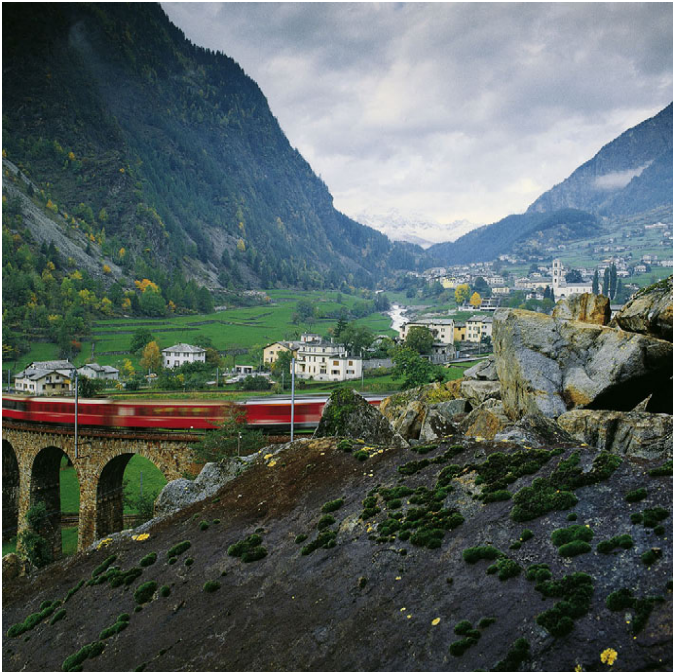
Bernina line > The Bernina railway on the circular viaduct at Brusio. R. Pedetti
