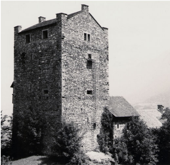
Sils i.D. > Ehrenfels Castle. Built in the first half of the 13th century. Renovated as a youth hostel in 1934. Ch. Meisser / Staatsarchiv, Chur
