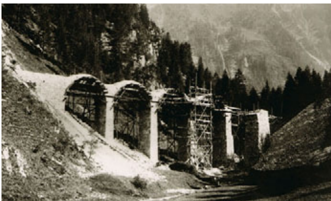
Albula line > Construction of the Clix Viaduct, 1902. Rhaetian Railway
