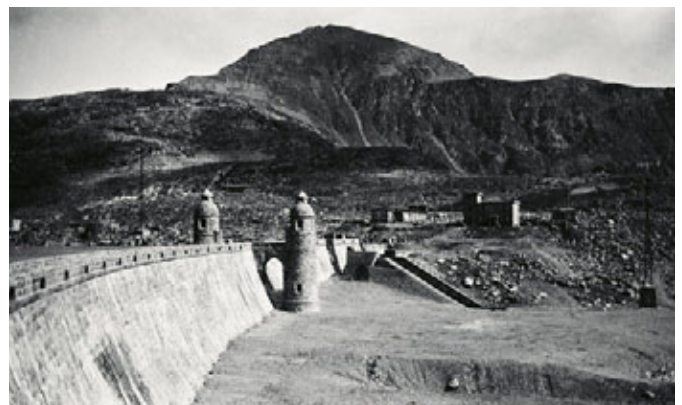
Lago Bianco > The south wall of the Lago Bianco with the 1911 valve tower (left) and the new valve tower built in 1927. Photograph before 1942. Rätia Energie AG, Poschiavo
