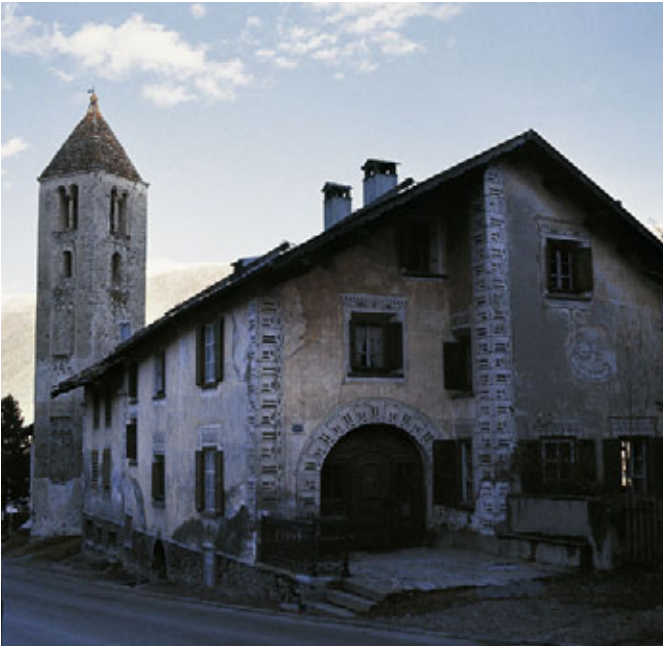
Celerina > Typical Engadin style house in the Crasta district (the tower of the Protestant St. Maria church in the background). Loaded hay carts could drive through the enormous door on the left of the façade straight into the barn. Denkmalpflege Graubünden, Chur
