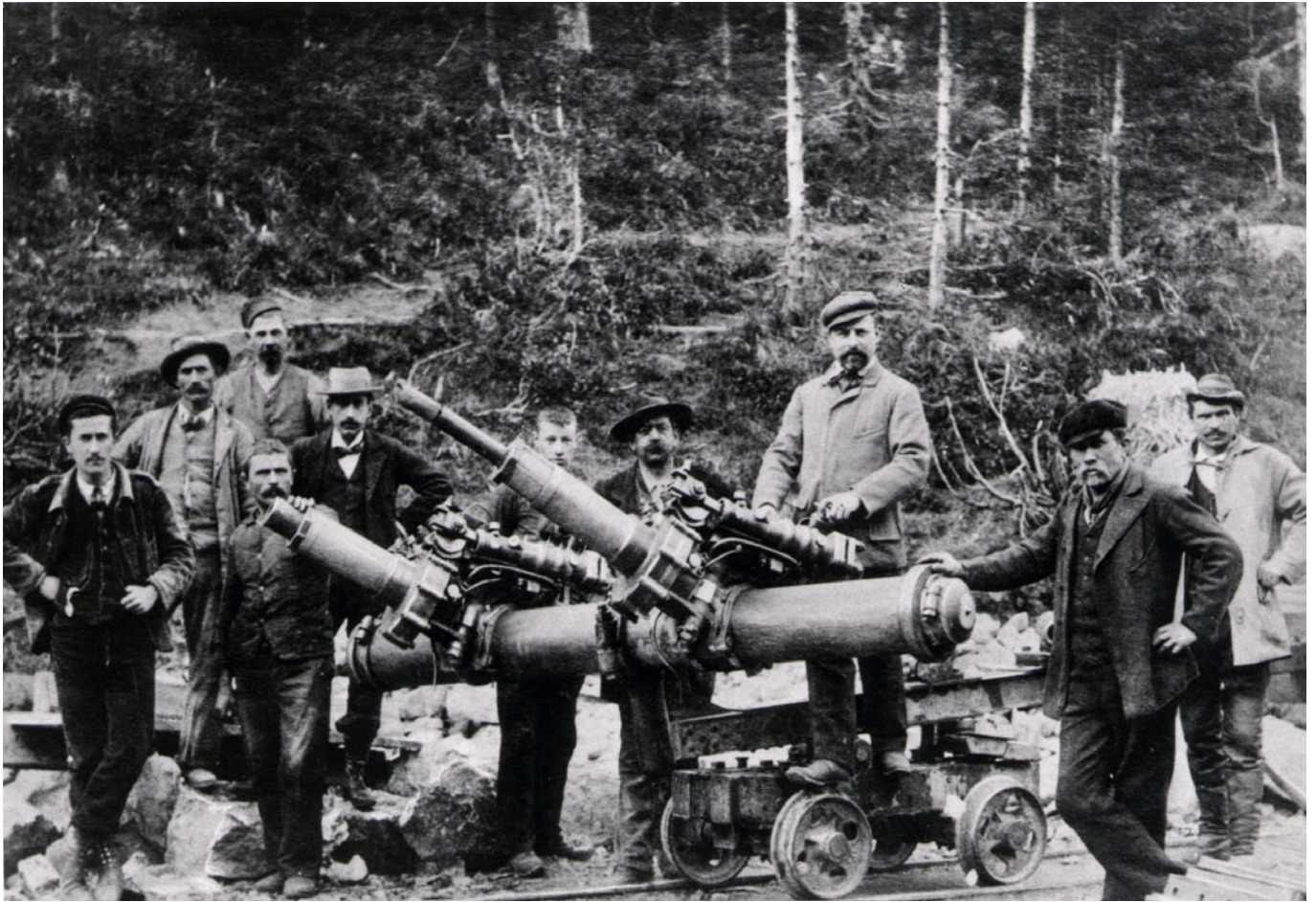
Albula Tunnel > Drilling team with the Brandt hydraulic drive drilling machine.
