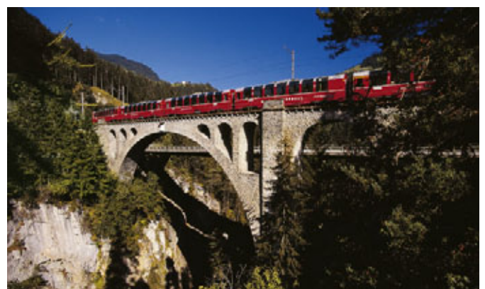
Solis > The Solis Viaduct is still in its original state. T. Keller
