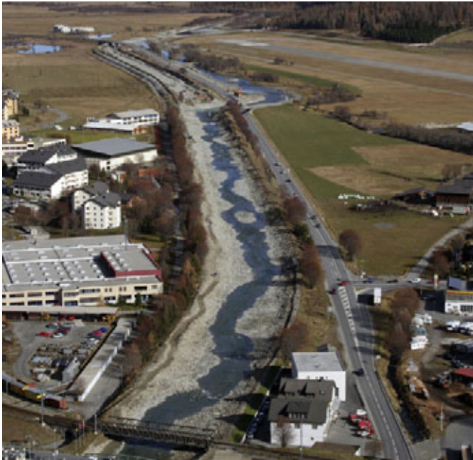
Samedan > The River Inn has been 'renaturalised' between Samedan and Gravatscha. Tiefbauamt Graubünden, Chur
