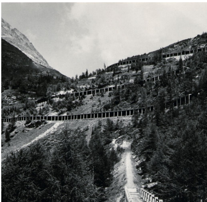
Bernina line > Galleries protect the three traverses across the Alp Grüm slope against avalanches. The photograph was taken later than 1951. Rhaetian Railway
