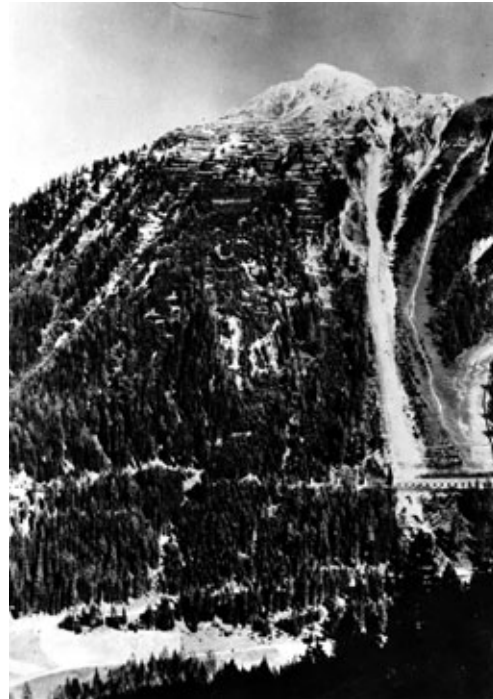
Muot avalanche baffle > Photograph 1938. Rhaetian Railway
