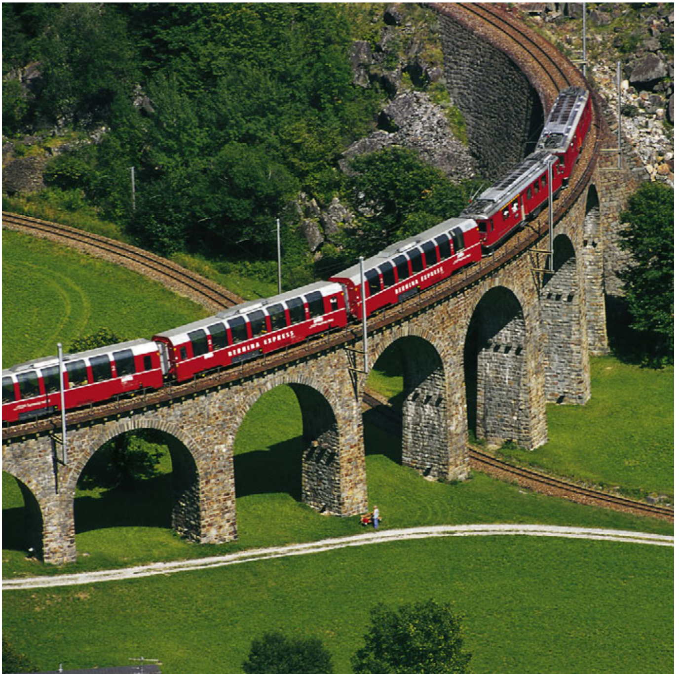
Bernina line > Circular Viaduct at Brusio. P. Donatsch
