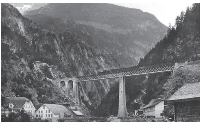
Gotthard Railway > Original Kerstelenbach steel truss bridge, about 1881. Collection G. Dinhobl
