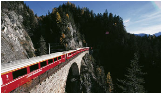
Albula line > The Stulsertobel Viaduct is one of the most striking viaducts between Filisur and the Bergünstein. T. Keller
