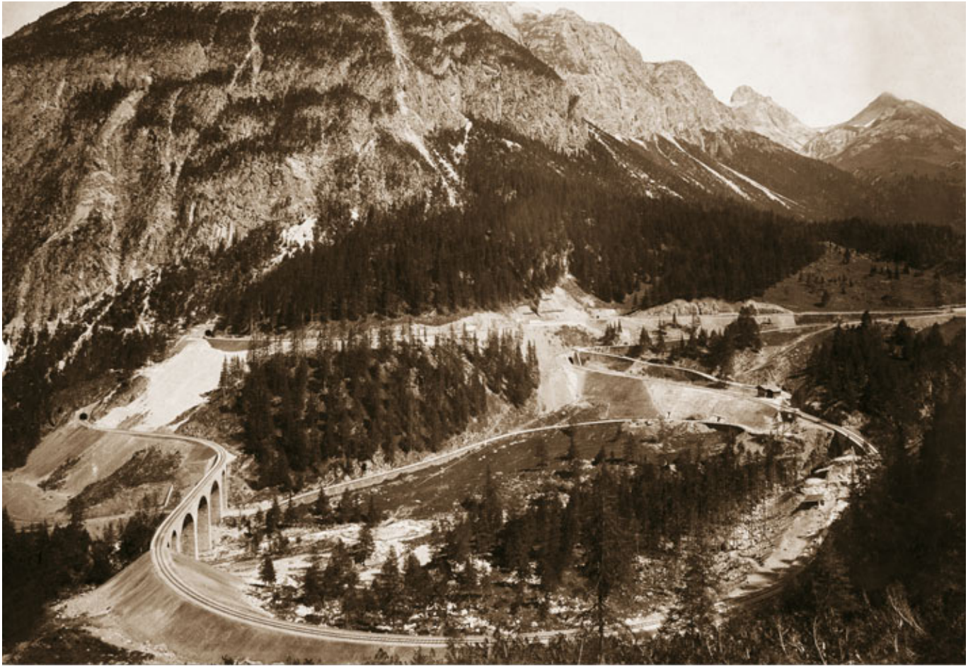
Albula line > Alignment between the Tuoa and Zuondra spiral tunnel, 1902. The terrain alterations necessary prior to construction are hardly visible today. Rhaetian Railway
