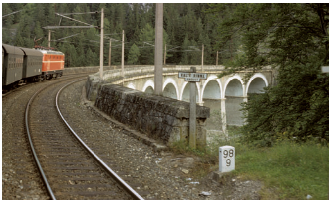
Semmering Railway > Stone arch viaduct across the Kalte Rinne. Photograph 1979. H.P. Bärtschi
