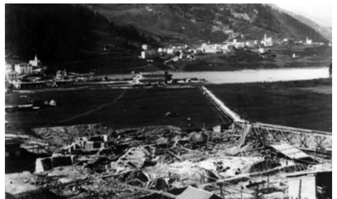
St. Moritz Bad > Construction of the Hotel Stahlbad, 1891/92. Dokumentationsbibliothek, St. Moritz
