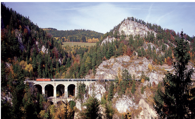
Semmering Railway > Viaduct across the Krauselklause. P. Glitzner
