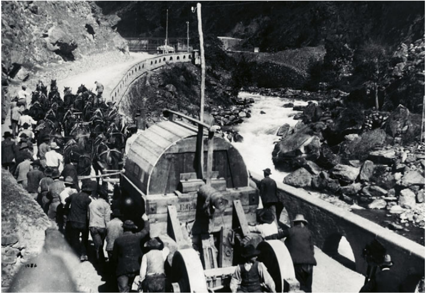
Transporting the pole wheel (rotating part of a generator) for a machine aggregate at Campocologno power station by horse and cart between Tirano and Campocologno. Photograph about 1906. Rätia Energie AG, Poschiavo
