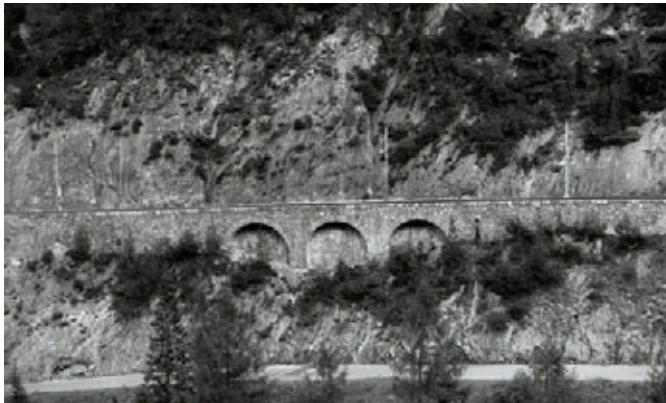
Albula line > Three arch design in the revetment wall at Fuegna ❶; the passengers can see it as the train emerges from the Rognux tunnel. J. Conzett
