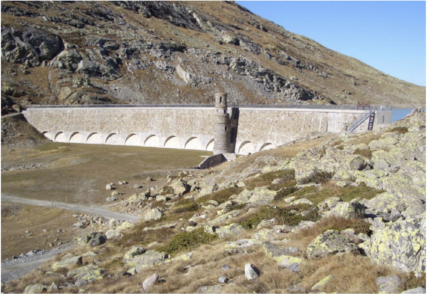
Diga Scala > The Lago Bianco south dam wall and service tower, clad in local stone, looks rather like a natural dam. L. Dosch
