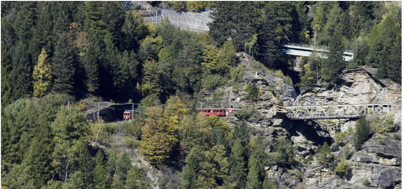
Bernina line > The two original bridges over the Cavagliasco river had to be replaced by steel bridges due to terrain movements. A. Badrutt
