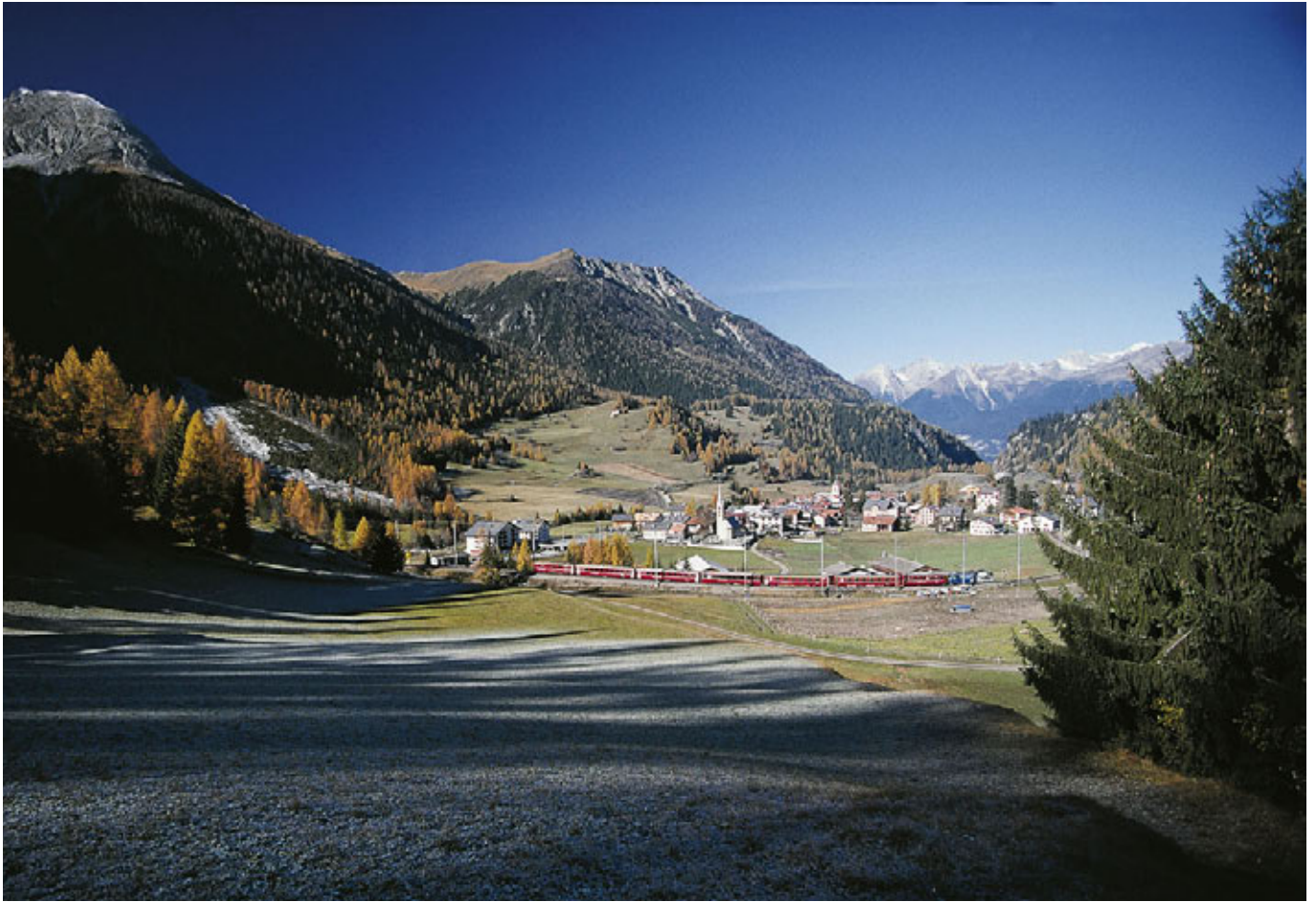
Albula line > The first elongation to overcome the natural step in the terrain between Bergün/Bravuogn and Preda is set in gently sloping meadows. T. Keller
