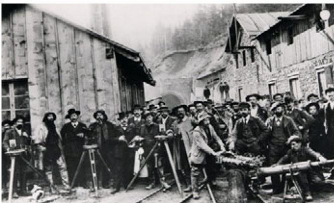
Albula Tunnel > The building team and the engineers collected in front of the building sheds at the Preda north portal for a photo session, 1902. Rhaetian Railway
