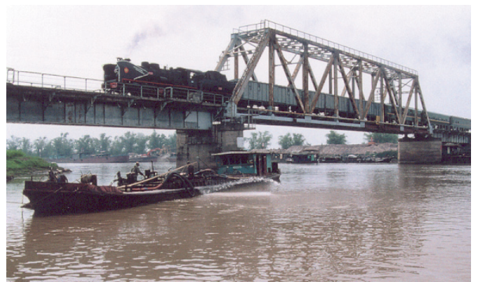
Yunnan Railway > Bridge on the delta of the Red River. Photograph 2003. H.P. Bärtschi
