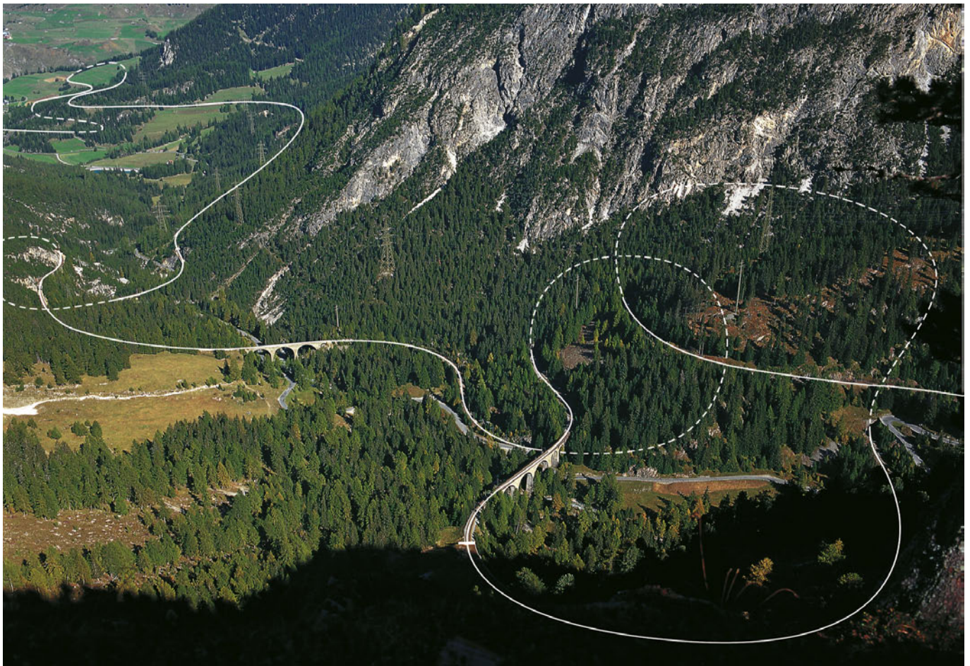
Albula line > Artificial elongation between Bergün/Bravuogn and Preda due to Viaducts and helical tunnel. The Albula Viaducts II (left) and III (right) can be seen clearly. Foto Geiger
