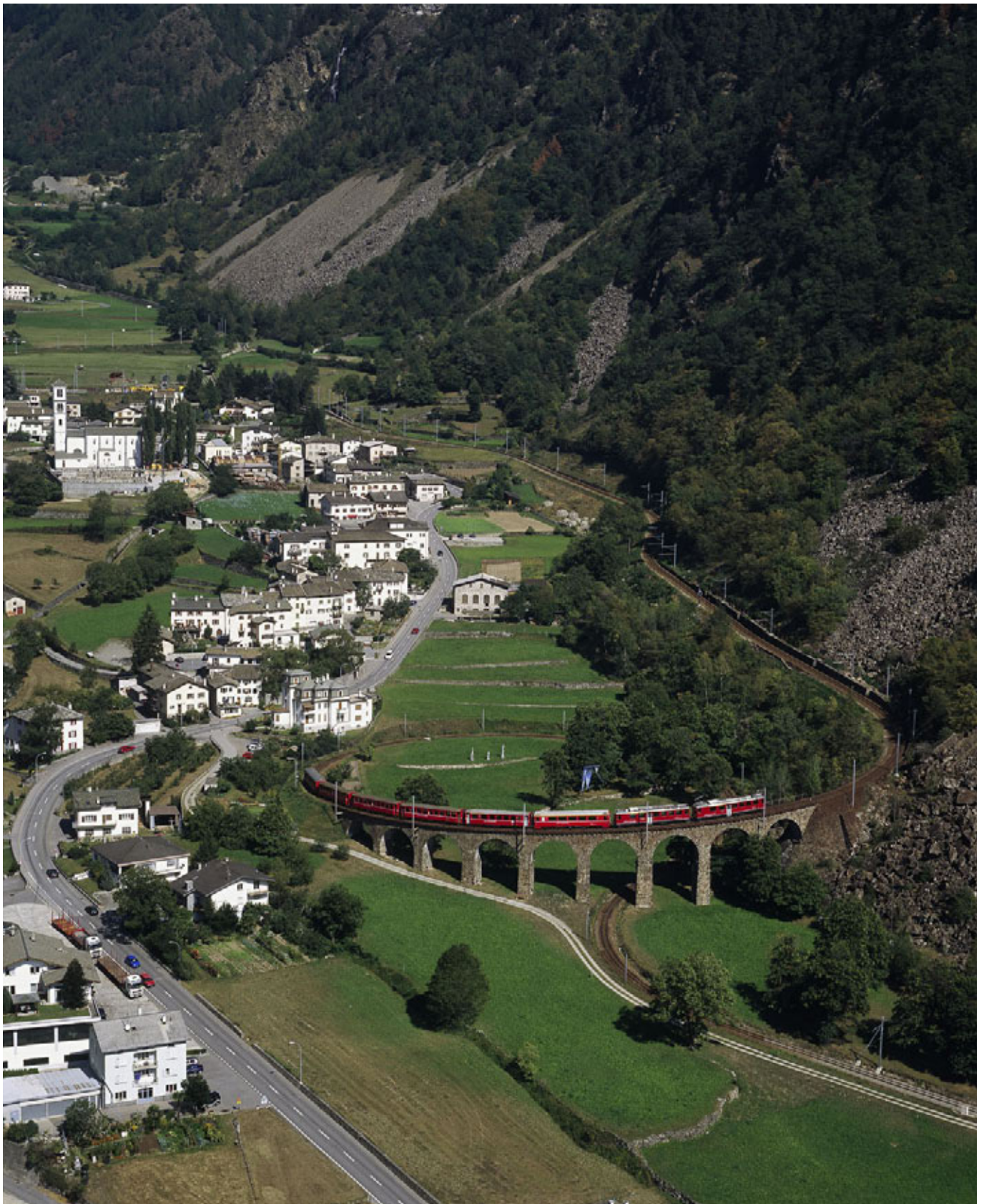
Bernina line > Aerial of the circular viaduct at Brusio. D. Enz/Rhaetian Railway
