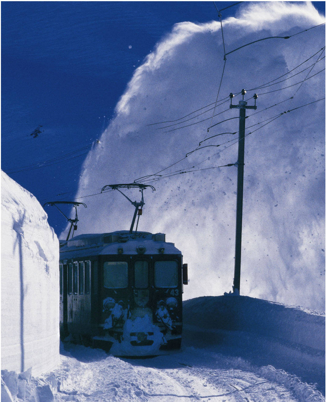
Bernina line > The railtrack is exposed to the elements, particularly in winter. P. Donatsch
