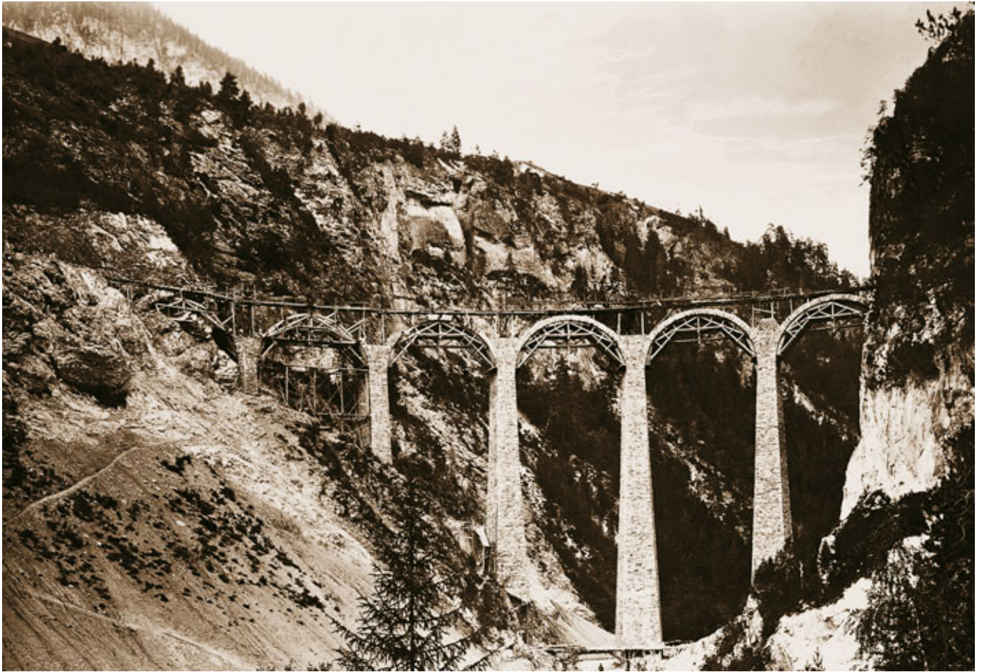
Albula line > Landwasser Viaduct near Filisur under construction, 1902. Rhaetian Railway
