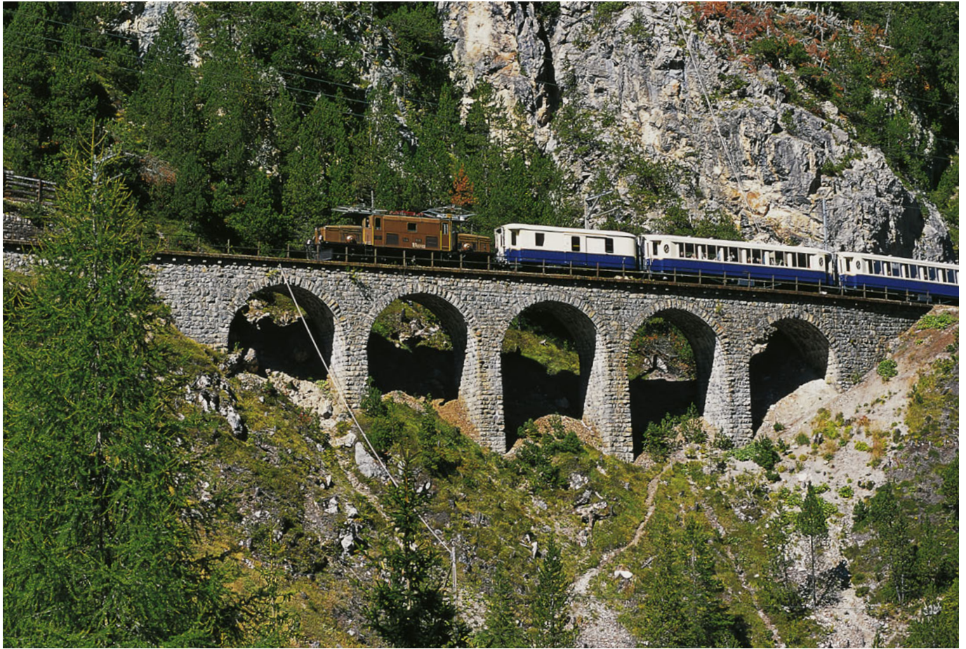
Albula line > Rognux inclined Viaduct. A "Crocodile" engine hauling the Pull- man Classic Express carriages. P. Donatsch
