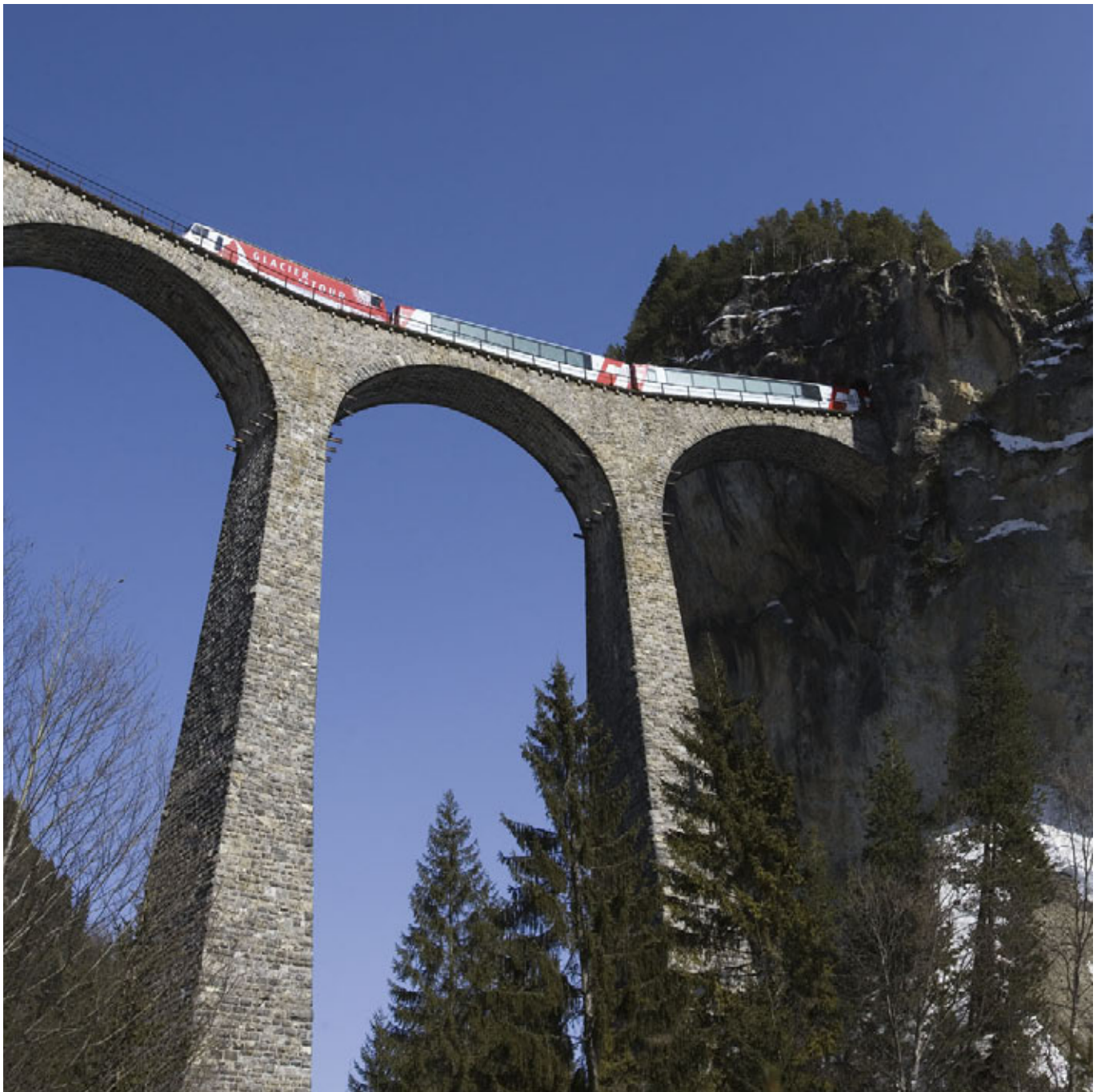
Albula line > The 65 m high Landwasser Viaduct, the most spectacular engineering structure between Thusis and St. Moritz. A. Badrutt/Rhaetian Railway
