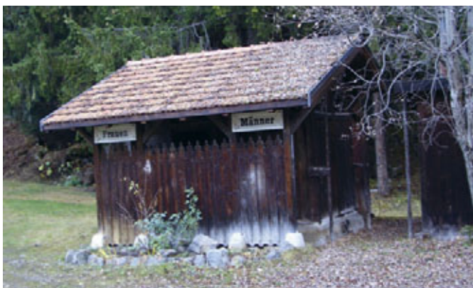
Albula line > Stugl/Stuls station. Passenger lavatory. L. Dosch
