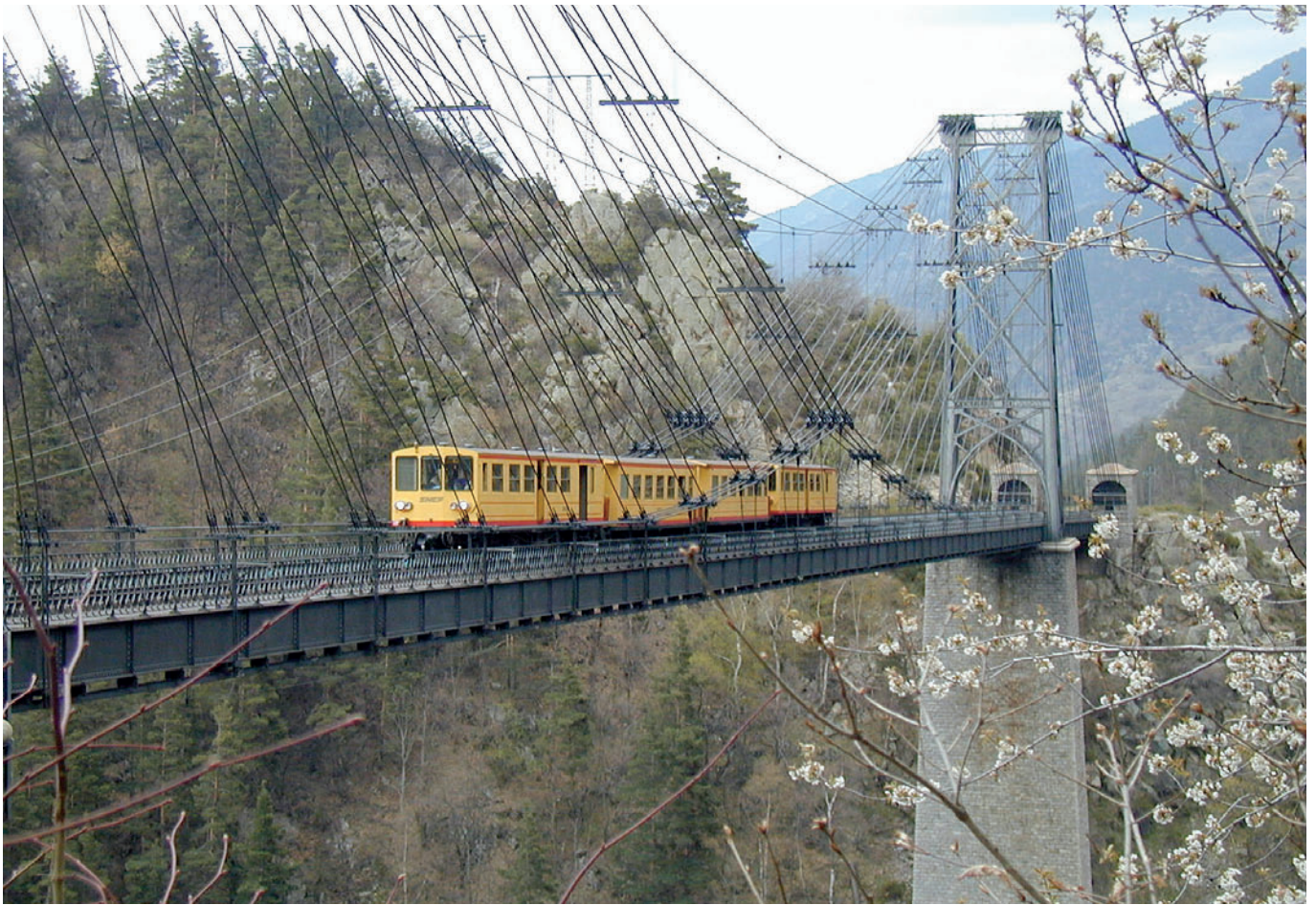
Train Jaune > "Pont suspendu Gislard" at La Cassagne. Photograph 2000. UTBM
