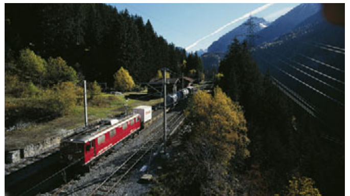
Albula line > The remote Stuls/Stugl crossing station is built on an outcrop high above the valley. T. Keller
