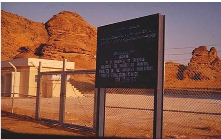
Figure 17. Guard house and sign board on the fenced site of Jubbah.
