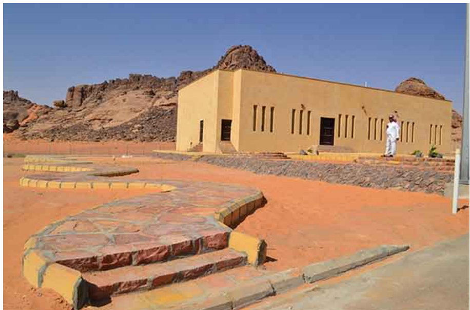
Figure 18. Visitors information centre at Jubbah.
