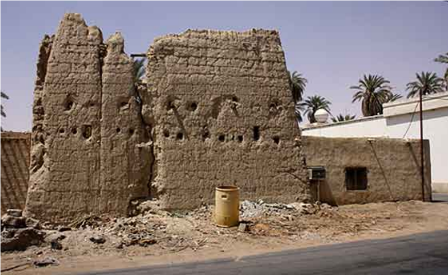
Figure 2.5. Decaying mud brick building in Jubbah in close proximity to the privately owned Al Naif Museum.
