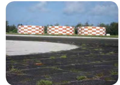
Water collection tanks
