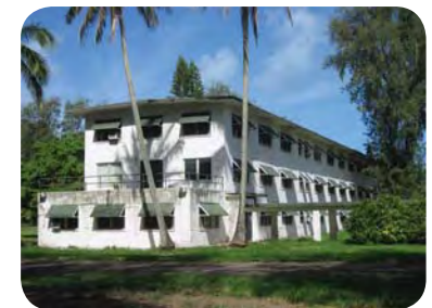
BEQ Barracks: replace with "green-designed" multi-plex units
