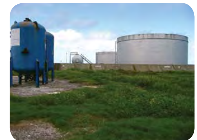
Old fuel tanks located in "no-dig" area
