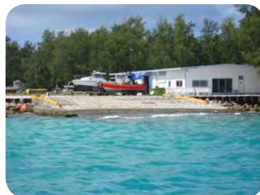
Historic seaplane ramp and existing boathouse
