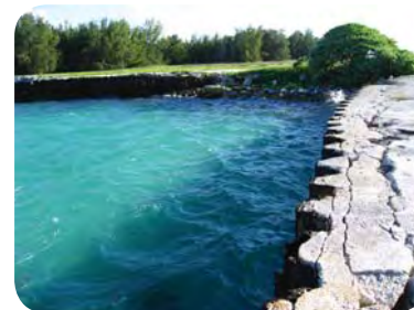
Inner Harbor seawall
