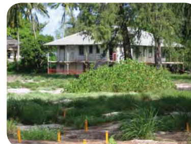
Cable Station building complex
