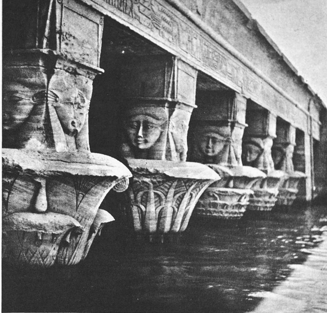
TOPS OF PILLARS are all that show of the Birth House on Philae when the gates of Aswan dam are opened in the month of October and the Nile slowly submerges the island's monuments.
