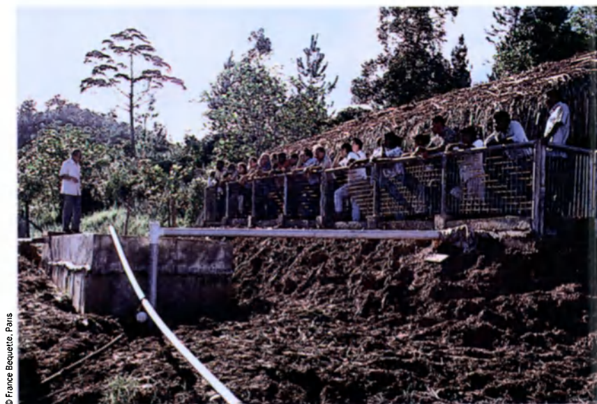
The nerve centre of the integrated farm is the biodigester (below), where plant waste and animal excrement ferment to produce biogas and residues for use as fertilizer.
