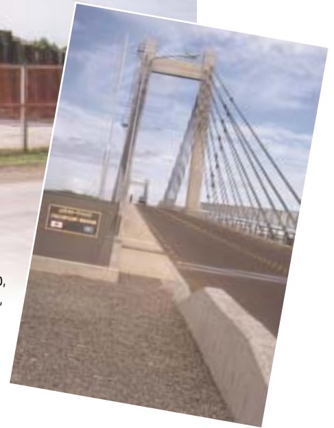
Batching plant for Palau's Compact Road, Babeldaob, and Friendship Bridge linking Koror to Babeldaob, Palau, February 2002.
