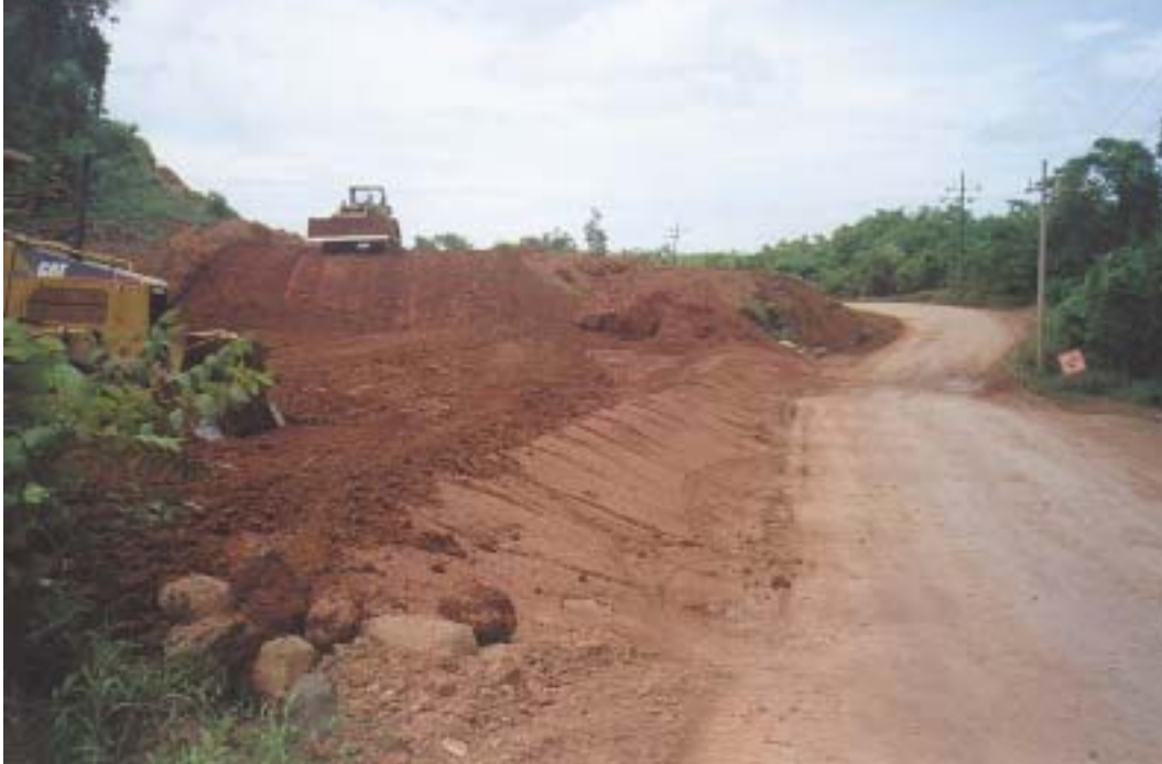
Many of the people working to build Palau's Compact Road are foreign workers, February 2002.
