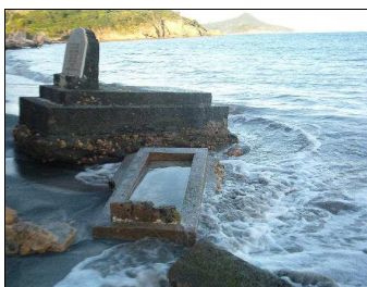
Graves in Carriacou being washed into the sea as a result of beach erosion
