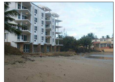
A great example of building too close to the sea from Puerto Rico
