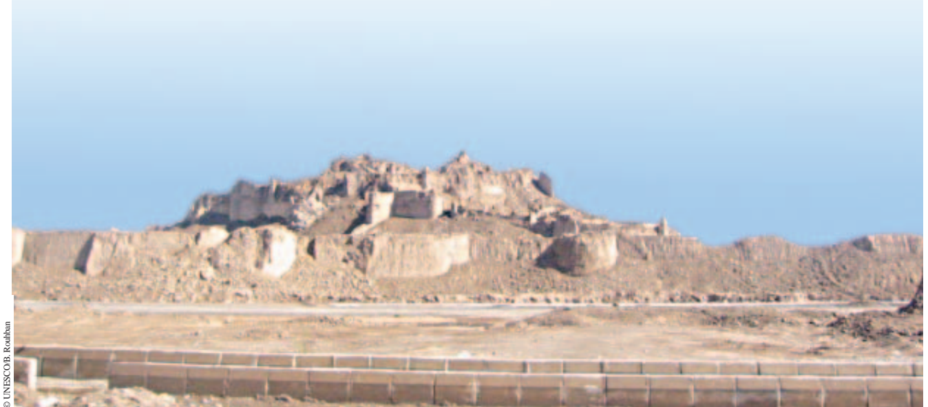
The badly damaged Bam Citadel (Arg-e-Bam)
