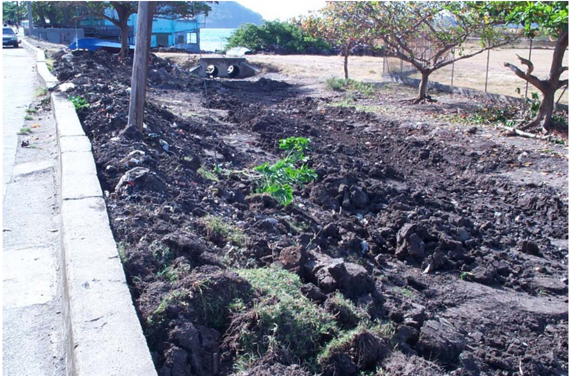
Trees and soil deposits being excavated
