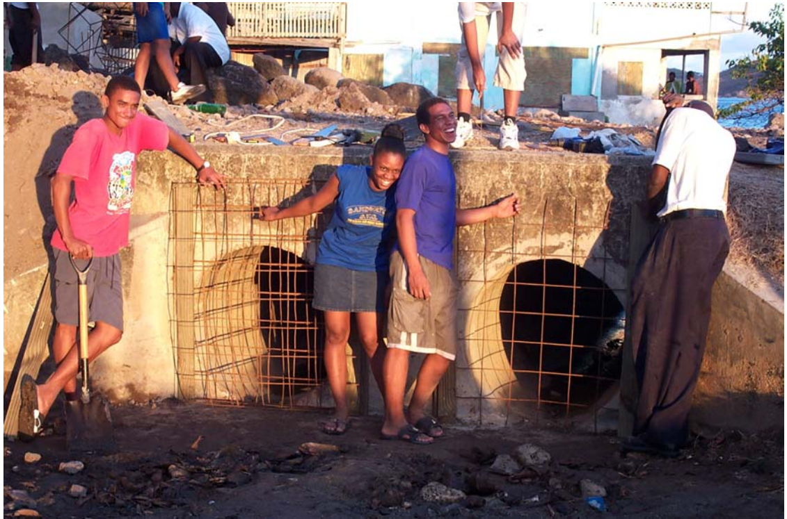
Constructing debris traps
