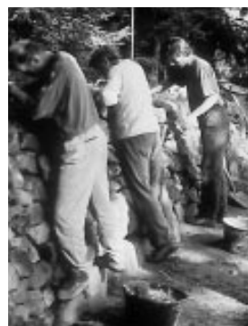
Rebuilding the drystone walls of the Cévennes terraces
