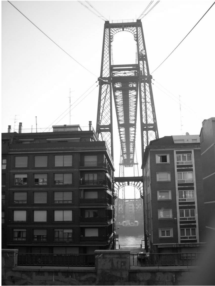
Bridge from the street
