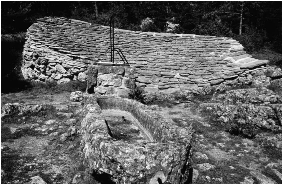
Roof shaped for collecting water (Saint Jean de Balme)
