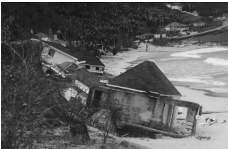
St Barthelemy: Hurricane damage, September, 1995
