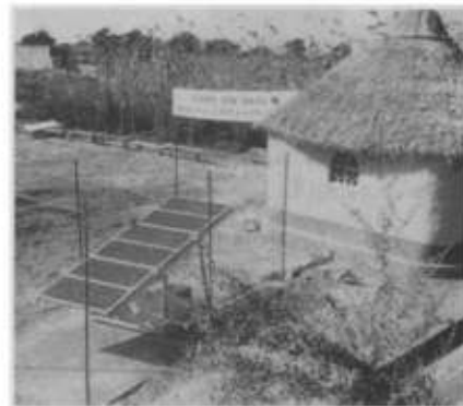
A photovoltaic generator supplies electricity for a refrigerator in Mali (Photo Jean-Luc Mabit/Total).
