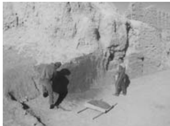
Protective plastering of the walls on both sides of the main gate
