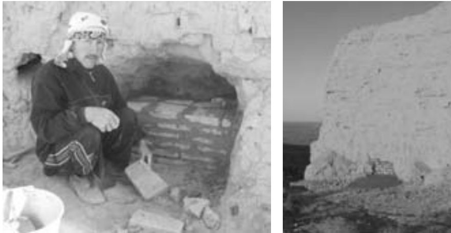
Sample reinforcement of standing walls
