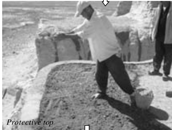
Backfilling of the tower
