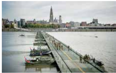
Pontoon bridge 2014 The Belgian and Dutch engineer battalions reconstructed the bridge (28 Sept 2013) to test technical and safety issues. © Jimmy Kets/Vredescentrum Antwerpen
