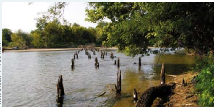
Foundation piles of the Medieval bridge at La Charité-sur-Loire.
