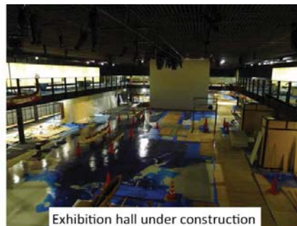
Exhibition hall under construction
