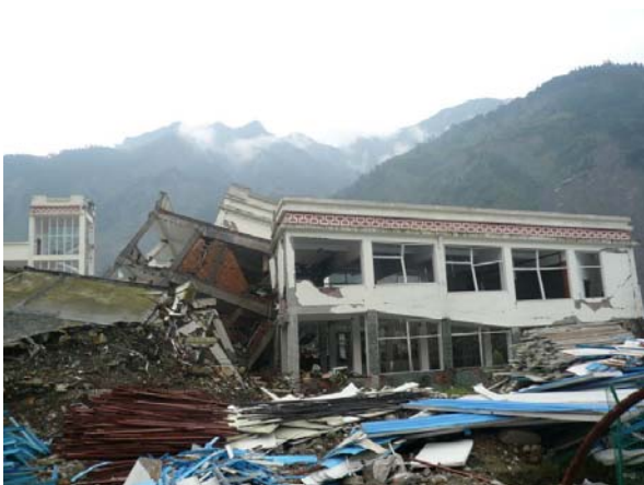
Figure 18. Collapsed junior high school buildings in Yingxiu (2008 ©T. Imamura)
