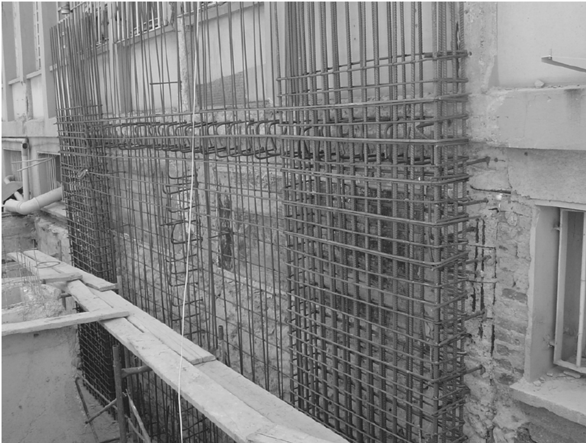
Figure 7. New added shear wall from exterior
