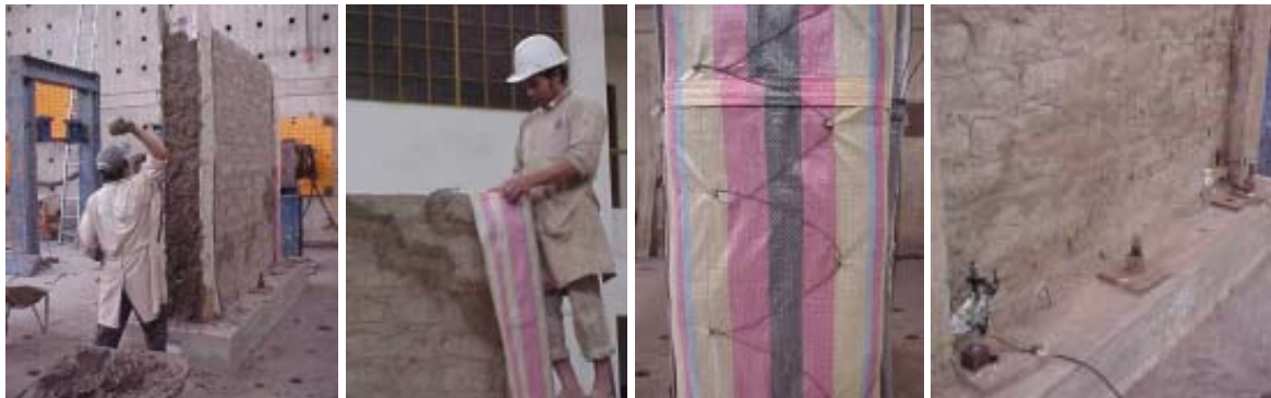
Figure 9. Four stages of reinforcement an adobe wall
