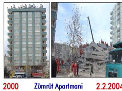
Figure 2. Zümrüt Apartment Building in Konya /Turkey collapsed due to gravity loads
