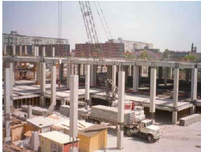
Figure 11. Commercial centers, totally prefabricated, Cost range 500 - 700 USD /m2
