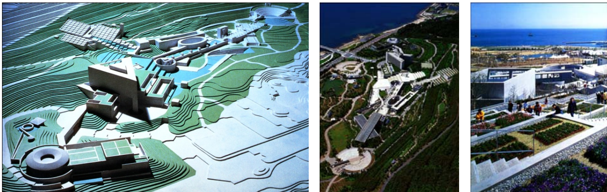
Figure 10. “Awaji Yumebutai” designed by Tadao Ando
