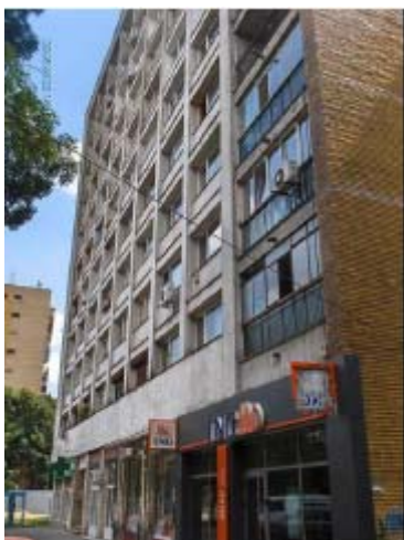
Figure 27. Soft and weak groundfloor RC building built in 1960's and retrofitting solution
