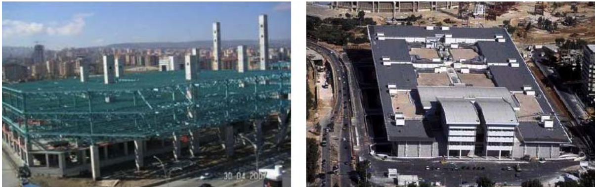
Figure 30. The Söğütözü Congress & Commercial Centre in Ankara (Turkey), isolated by means of 105 German SIP devices in 2007 (left), and the International Broadcasting Centre in Athens (Greece), isolated by means of 292 Italian HDRBs in 2003 (right)
