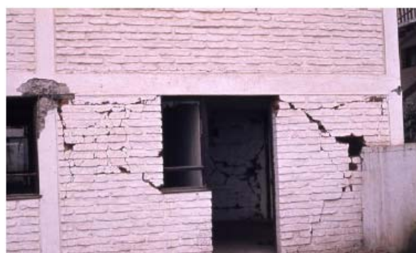
Figure A9. Reinforced / Confined Masonry building in Melipilla. Damage to unconfined masonry walls in the Ground floor Upper floors have little or no damage.
