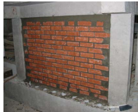
Figure 15. Strengthening of a bare frame by integrated high strength brick wall
