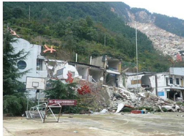
Figure 21. Collapsed elementary school buildings in Beichuan (2008 ©T. Imamura)
