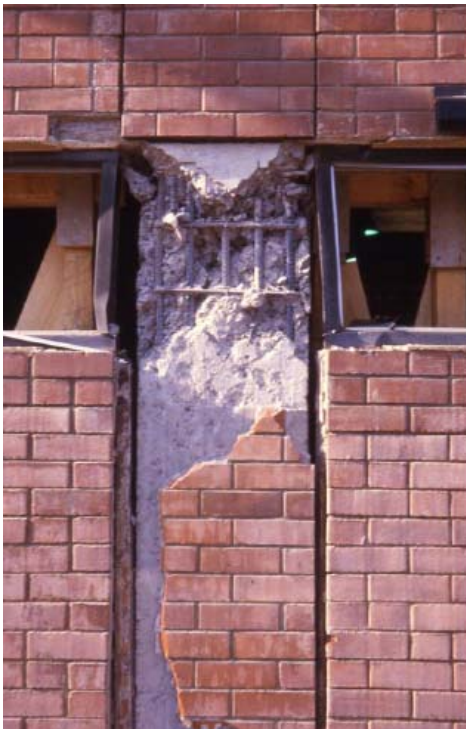
Figure A8. Fundacion Chile Building in Santiago. Damage to columns in a two story reinforced concrete frame building. “Short column effect” due to infill walls not properly separated.
