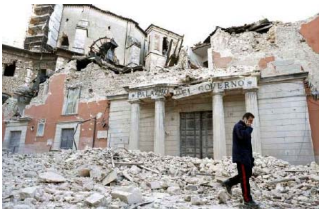
Figure 6. L'Aquila (April 2009): collapse of the town collapse of the prefecture, a symbol of lack of prevention
