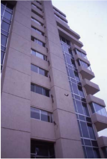
Figure A7. Don Jose Building in Vina del Mar. Reinforced concrete, shear walls and coupling beams. Damage to coupling beams (left) and to interior partitions (heavy and brittle). Note the large and heavy pieces of partition material damaging furniture.
