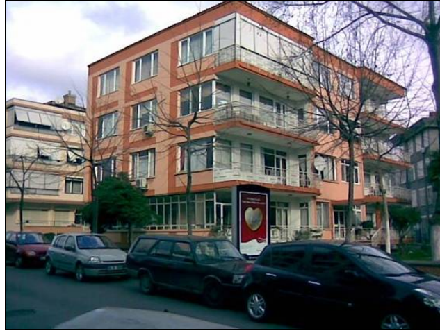
Figure 7. Appearance of a typical reinforced concrete frame building in the survey area
