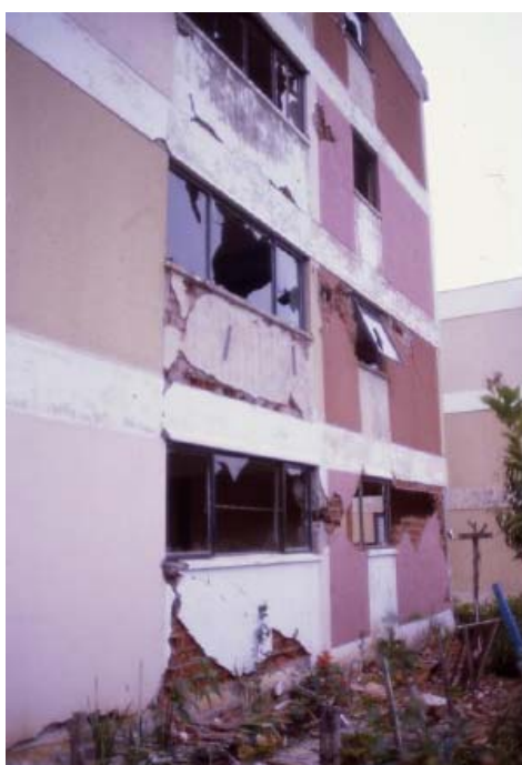
Figure A10. Confined Masonry / Reinforced Concrete building in Vina del Mar. Damage to unconfined masonry walls and to the shear walls in the Ground floor. Buildings are located on a hill side. Topographic effect is significant, as same buildings in a flat area did not have damage.
