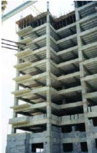
Figure 9. Engineered dwelling, middle-high economical level, built with partially prefabricated floor. Cost range 550 - 800 USD/m 2
