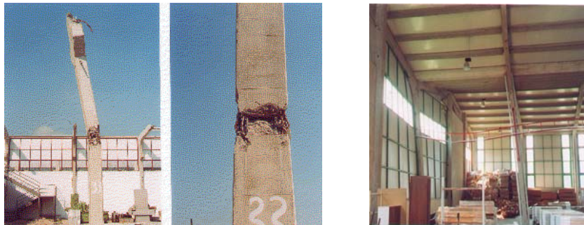
Figure 6. Industrial type simple precast buildings
