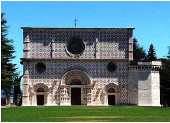
Figure 8. The Cathedral of Santa Maria di Collemaggio, a rare example of Abruzzo Romanic style, prior to the earthquake and the collapse of its roof in its baroque (not yet retrofitted) part. The façade, which had been protected by some elastic-plastic dampers (EPDs) installed on the roof some years ago (see Figure 25), survived the earthquake (however, a steel scaffold, recently erected for an already planned retrofit, certainly helped)
