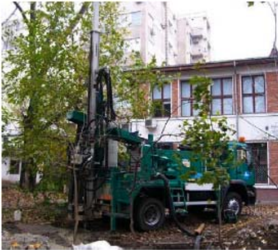
Figure 21. Drilling equipment on truck
