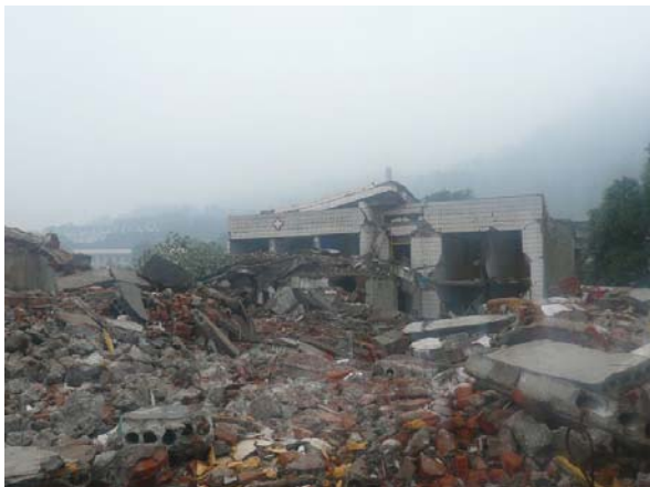
Figure 20. Heavily damaged hospital surrounded by debris in Hanwang (2008 ©T. Imamura)
