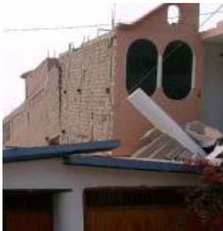
Figure 5. Non belt beam
