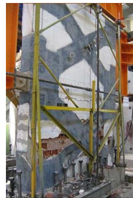
c) Observed damages at the end of testing
