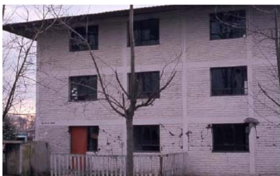
Figure A9. Reinforced / Confined Masonry building in Melipilla. Damage to unconfined masonry walls in the Ground floor Upper floors have little or no damage.
