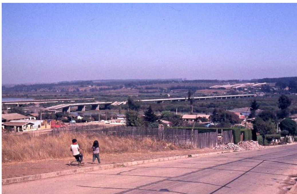
Figure A2. Llo-lleo-Santo Domingo Bridge. Several spans collapsed due to ground failure under the piers.
