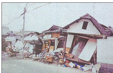
Figure 7. Collapsed houses in "Ashiya"
