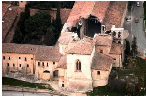
Figure 8. The Cathedral of Santa Maria di Collemaggio, a rare example of Abruzzo Romanic style, prior to the earthquake and the collapse of its roof in its baroque (not yet retrofitted) part. The façade, which had been protected by some elastic-plastic dampers (EPDs) installed on the roof some years ago (see Figure 25), survived the earthquake (however, a steel scaffold, recently erected for an already planned retrofit, certainly helped)
