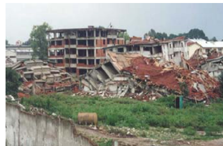
Figure 5. Total collapse of low cost-low rise reinforced concrete buildings
