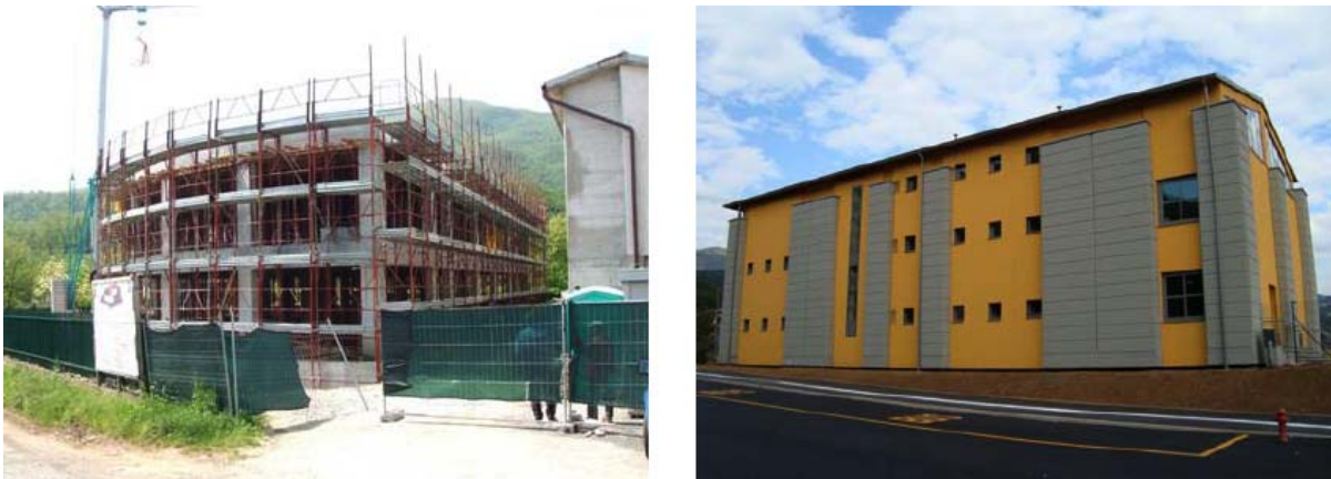
Figure 16. The first new school building of Mulazzo (Massa Carrara), protected by Lead Rubber Bearings (LRBs) and SDs (right) and the new primary and secondary school of Galliciano (Lucca), protected by HDRBs and completed in September 2009. They are two of the 5 schools reconstructed (3) or being reconstructed with SI in Tuscany, in seismic zones 2 (safety of the Mulazzo school will be certified by A. Martelli)
