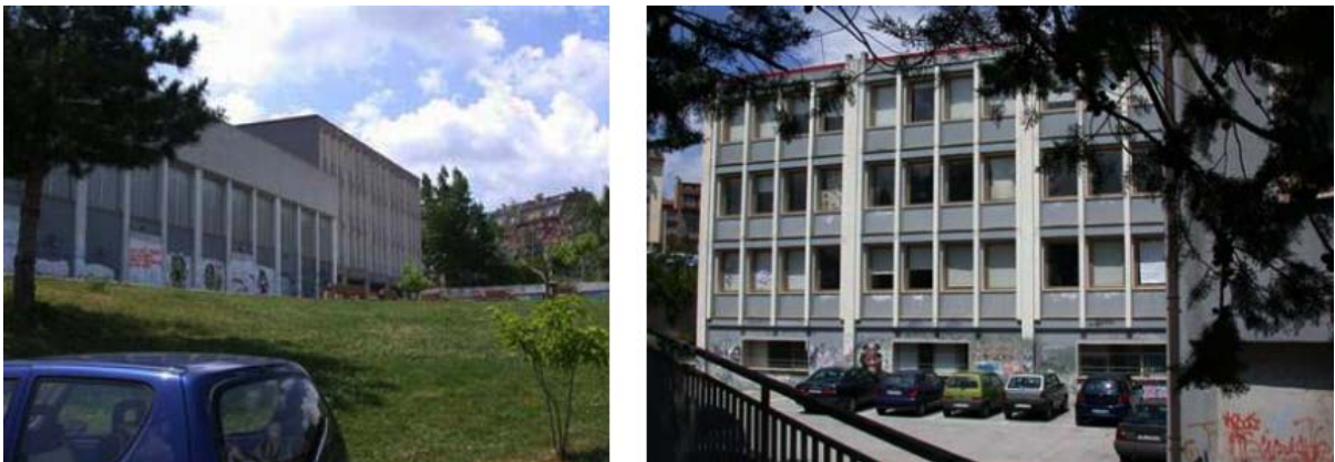
Figure 18. Romita High School for scientific studies of Campobasso (hosting about 1,300 students), in seismic zone 2, which is at last now being partly demolished and will be reconstructed with SI, due to its very poor concrete quality (as demonstrated by a study of ENEA, performed after the 2002 Molise and Puglia earthquake). Safety of the new seismically isolated buildings will be certified by A. Martelli
