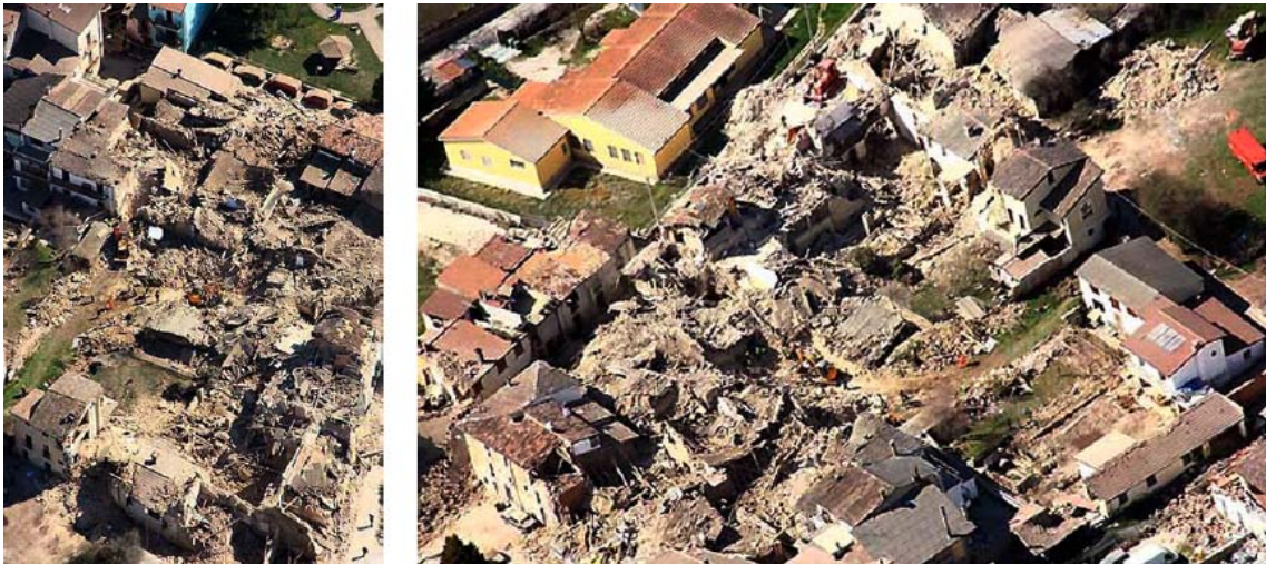
Figure 5. L'Aquila (April 2009): aerial views of some parts of the town where buildings collapsed or were heavily damaged
