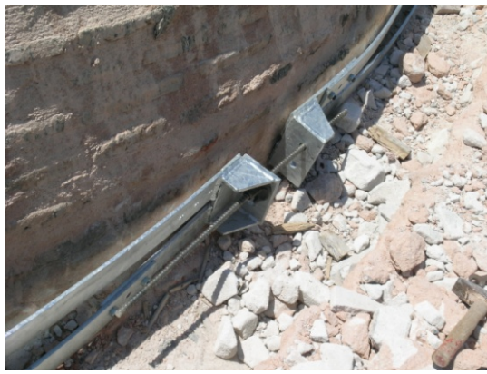
Figure 4. Applied steel ring detail
