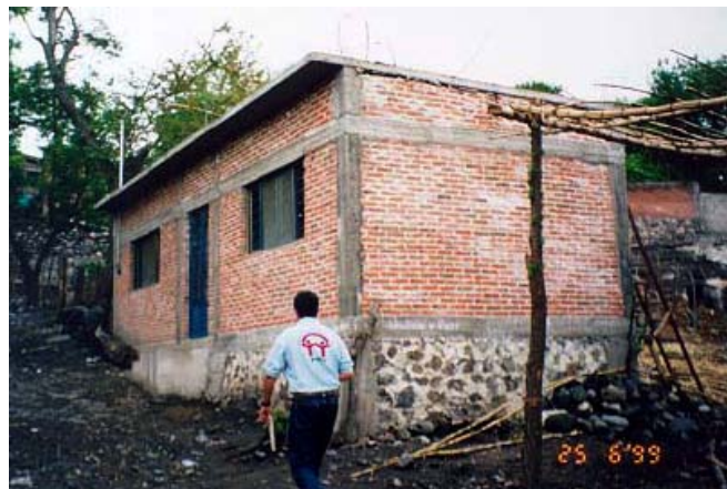
Figure 6. Non-engineered house, generally by self construction used by a single family. Construction average cost is 100 USD/m 2
