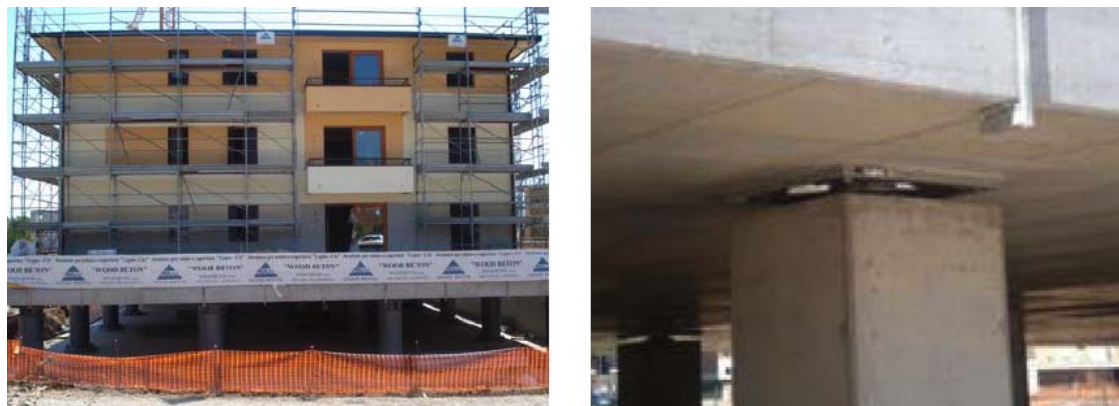
Figure 24. One of the 184 seismically isolated pre-fabricated houses erected at L’Aquila for the homeless residents and a Sliding Isolation Pendulum (SIP) device installed to isolate its supporting slab
