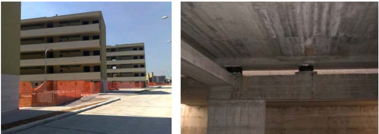
Figure 21. The 4 r.c. dwelling buildings of the new San Samuele Quarter of Cerignola (Foggia), in seismic zone 2, first application of the new Italian seismic code to isolated dwelling buildings, completed with 124 HDRBs (right) in May 2009, with safety certification of A. Martelli.
