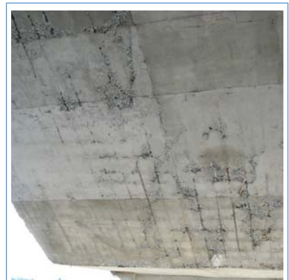
(b) A cast in situ stairway
