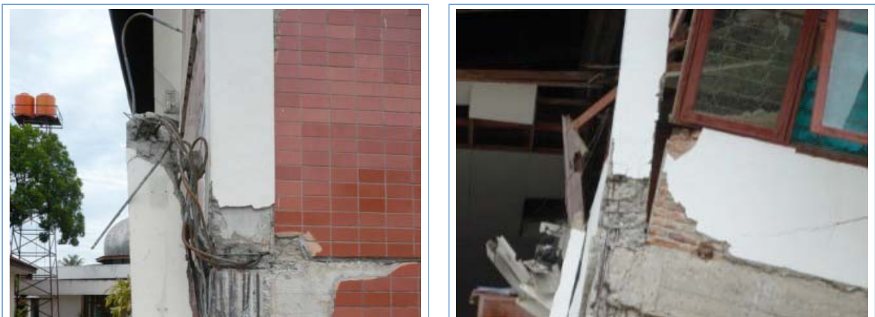
Figure 6 “Strong beam, weak column”
