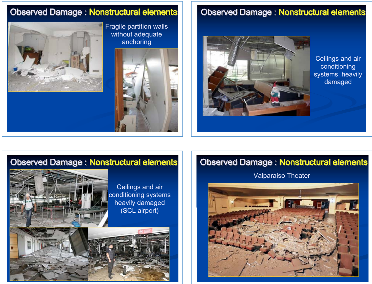
Figure 16 Typical damage to non-structural elements
