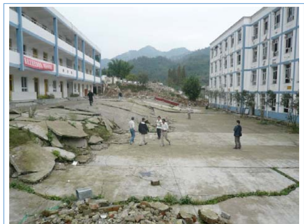
Figure 23 School building (left) raised 2 m by the fault in Bailu (© 2008 T. Imamura)
