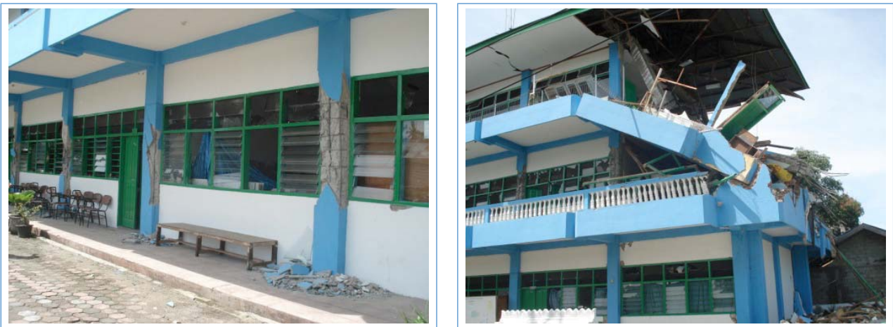
Figure 7 Short column effect
