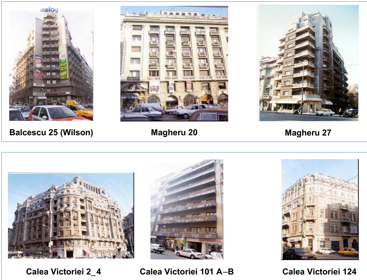
Figure 10 Architectural heritage buildings in central Bucharest: examples of tall RC buildings built before 1940 in the city centre
