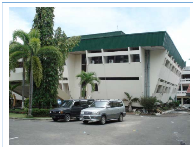
Figure 8 Poor distribution of mass
