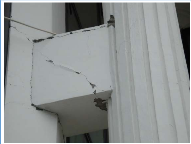
Figure 3 Structural damage to beams and columns
