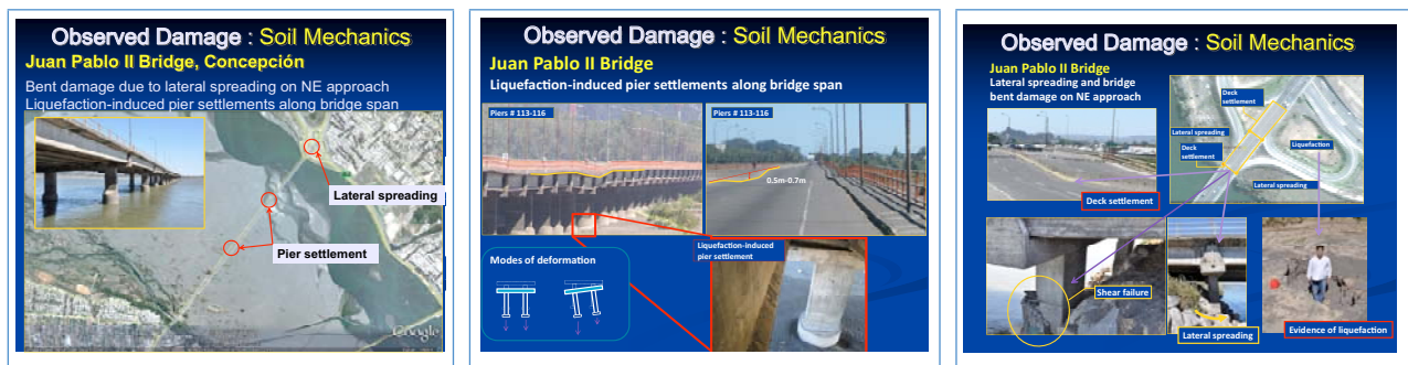
Figure 19 Bridge failure due to liquefaction and settling
