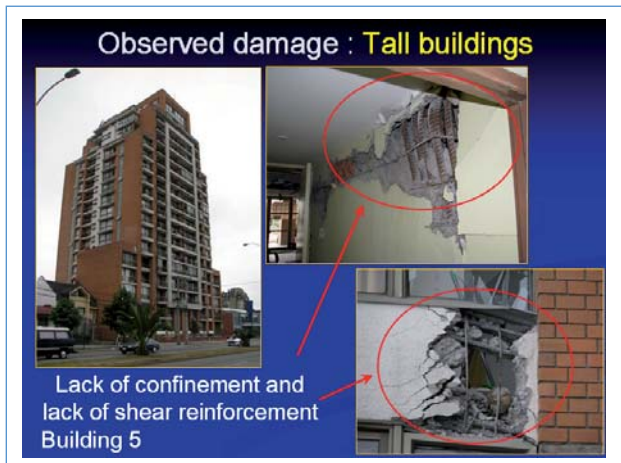
Figure 14 Typical failure due to lack of confinement in compressed wall heads
