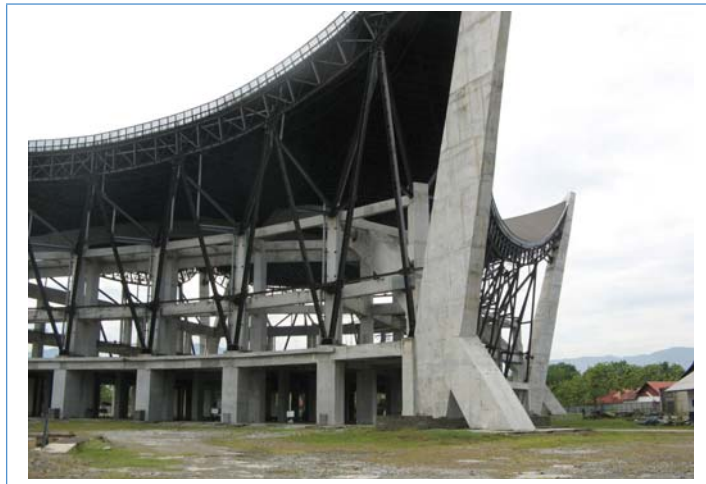
Figure 2 Mosque under construction, surviving intact
