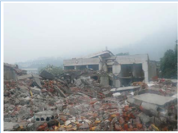
Figure 24 Heavily damaged hospital surrounded by debris in Hanwang (© 2008 T. Imamura)
