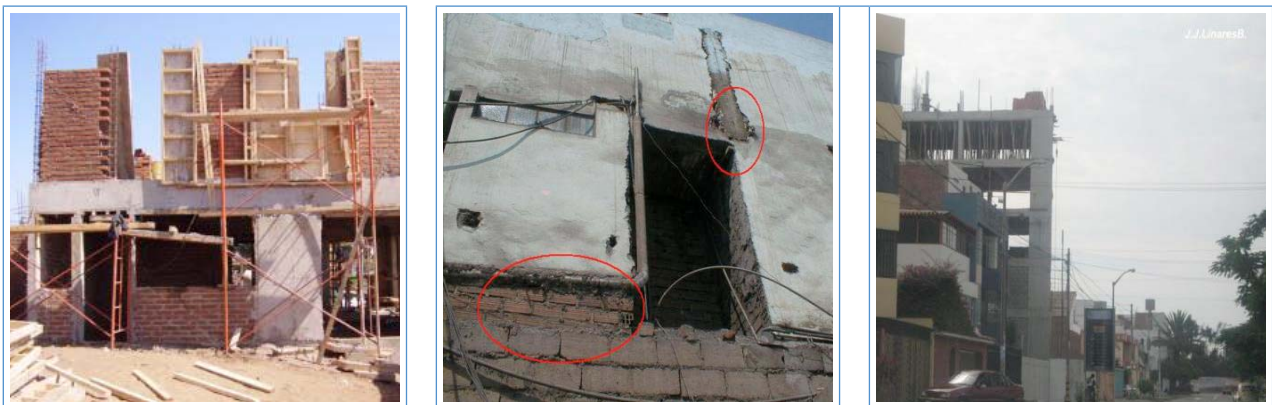
Figure 9 Typical non-engineered buildings in Peru (Photos by CISMID-UNI Peru)
