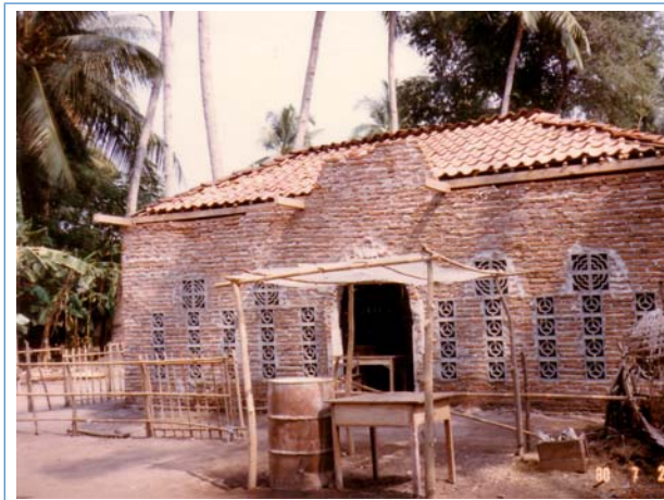
(a) Unreinforced brick masonry (Indonesia)
