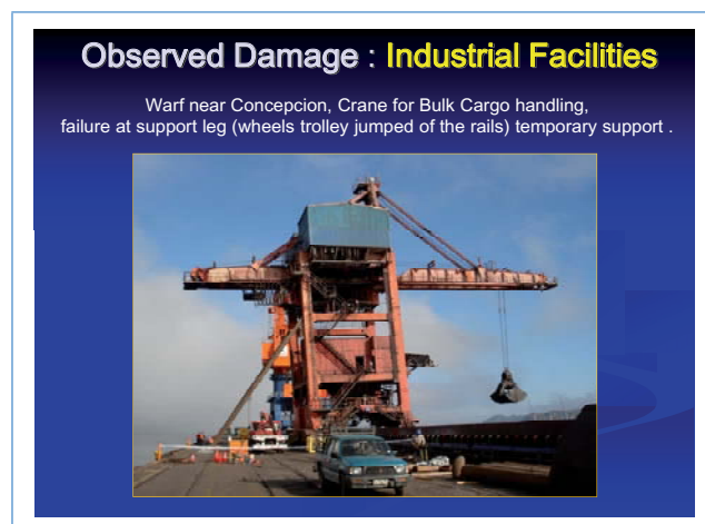
Figure 24 Crane on a wharf near Concepción with failure of the support leg
