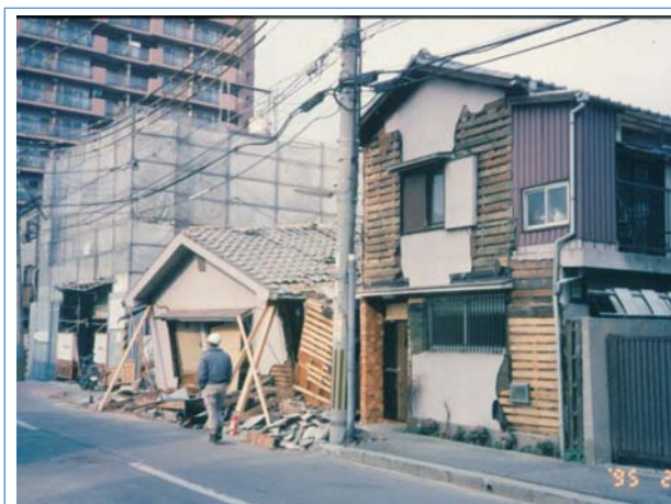
(a) Damaged wooden house (Japan)
