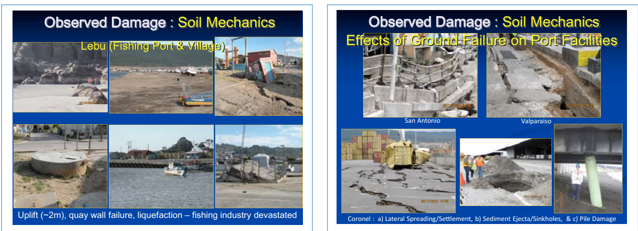
Figure 21 Soil failures in port facilities.
