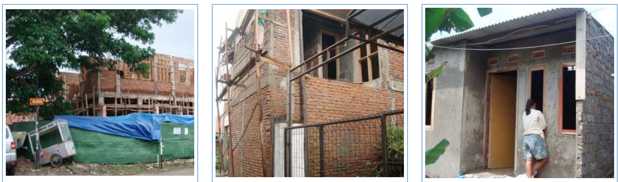
Figure 7 Typical non-engineered buildings in Indonesia (Photos by CDM ITB, Indonesia)
