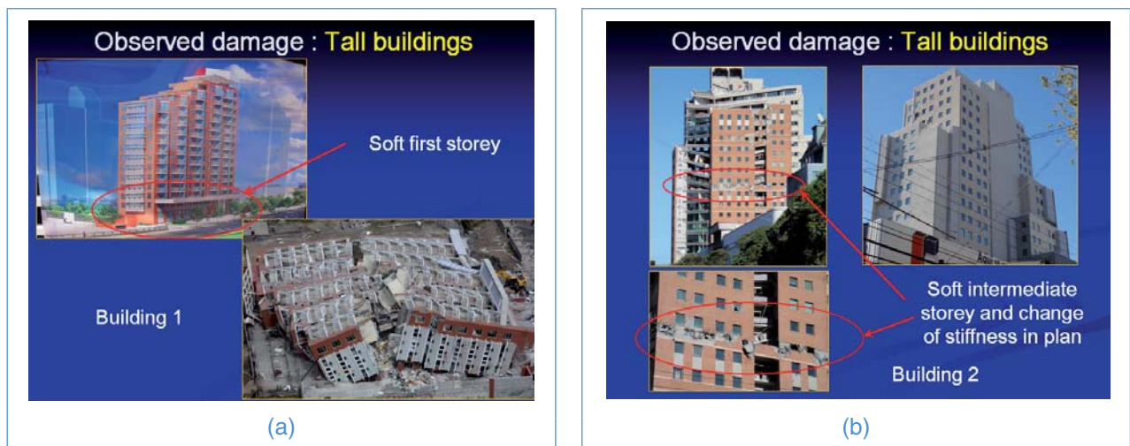
Figure 13 (a) Collapsed building with soft first storey, and (b) building with partially collapsed soft intermediate storey
