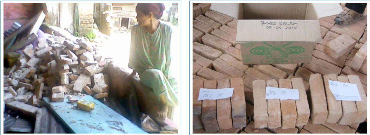
Figure 2 Brick samples from collapsed houses
