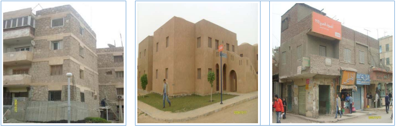
Figure 10 Typical non-engineered buildings in Egypt (Photos by NRIAG, Egypt)
