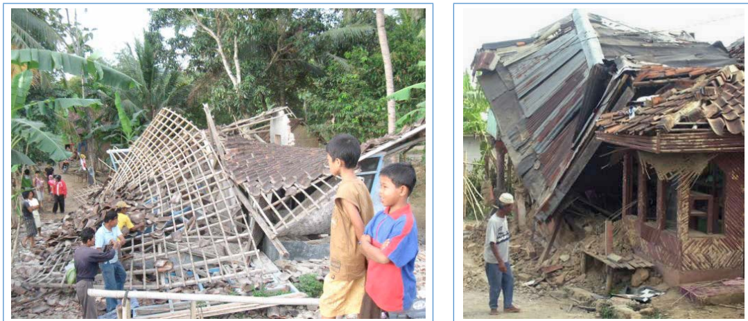
Figure 2 Houses collapsed after the Jogjakarta earthquake
