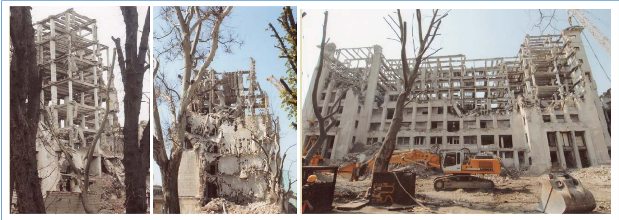
Figure 16. MICM building demolished in 2007, Calea Victoriei, Bucharest
