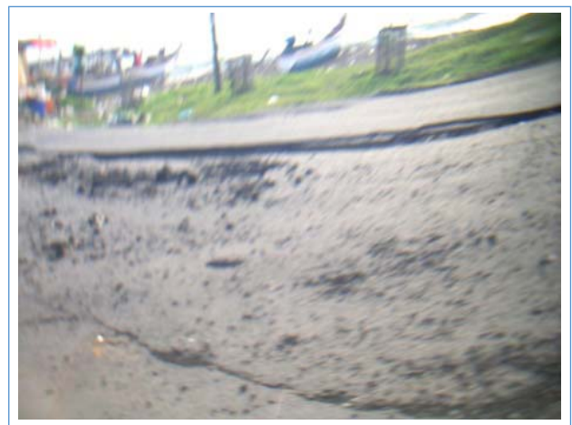
Figure 3 Liquefaction: (a) lateral movement causing a road to crack, Jl. Samudera, and (b) sand from the bottom of a road experiencing landslides, Jl. Samudera
