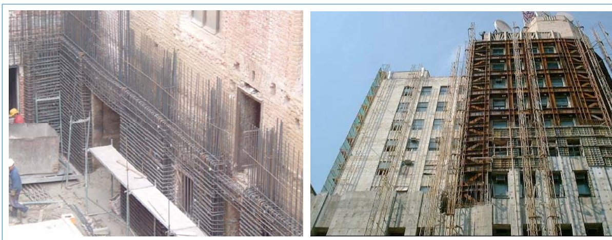
Figure 12 Retrofitting of (a) the Justice Palace, 2006, and (b) the Telephone Palace, 2002
