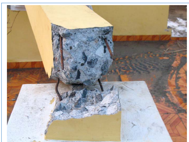
Figure 1 Column component after collapsing during the aftershock
