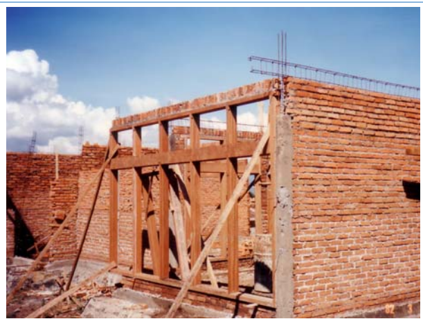
(b) Confined masonry under construction (Indonesia)
