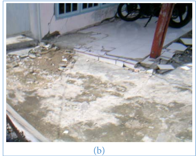
Figure 1 Liquefaction: (a) soil settlement at Jl. Gereja, and (b) sand ejected from the fissure floor in the residential complex at the National University of Padang
