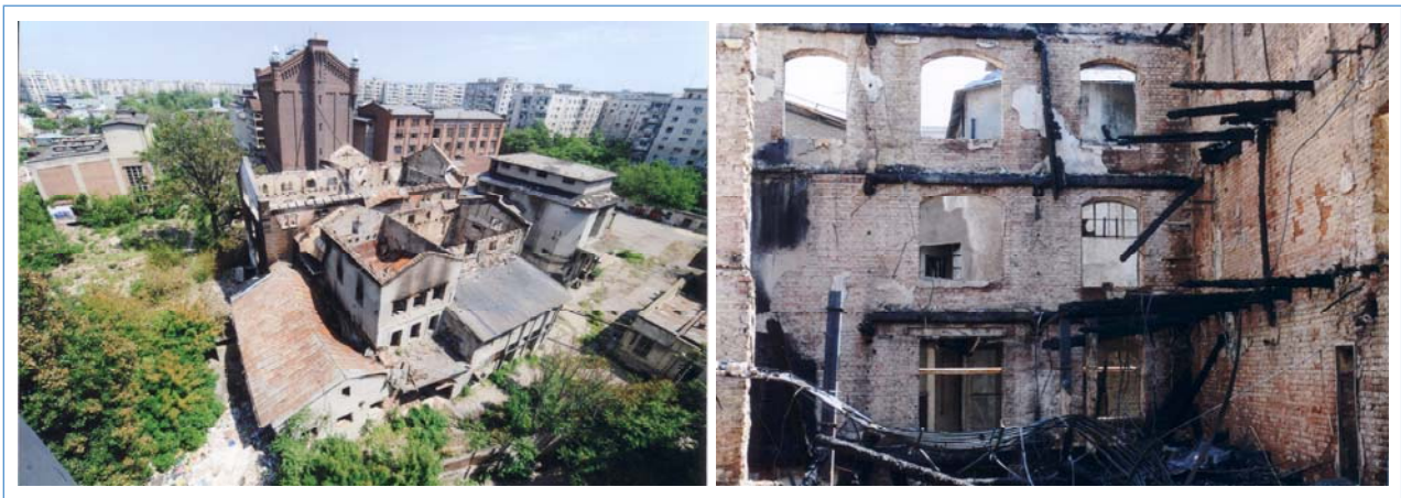
Figure 17. Arson and vandalism precipitated the self-collapse of the Asan Mill, industrial heritage, Bucharest, 1853
