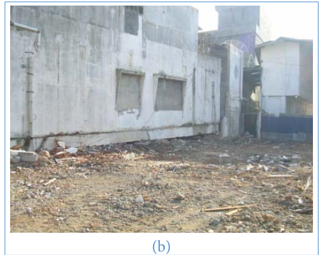
Figure 2 Liquefaction: (a) deformation of the soil layer due to the river wall breaking, Jl. Gereja, and (b) differential settlement of subgrade foundations
