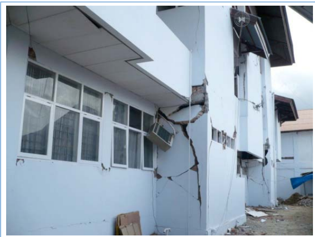
Figure 4 Damage to partition walls
