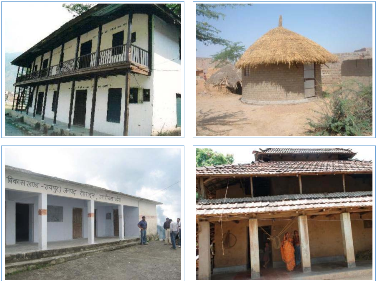
Figure 6 Typical non-engineered buildings in India (Photos by SEEDS Technical Services, India)
