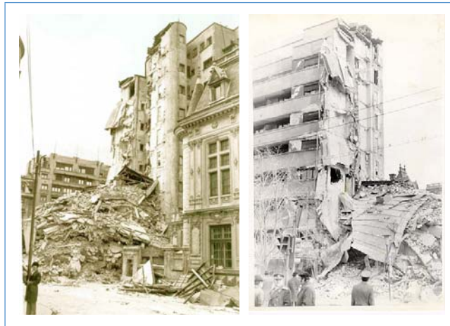
Figure 6 Typical collapse of pre-war tall reinforced-concrete buildings
