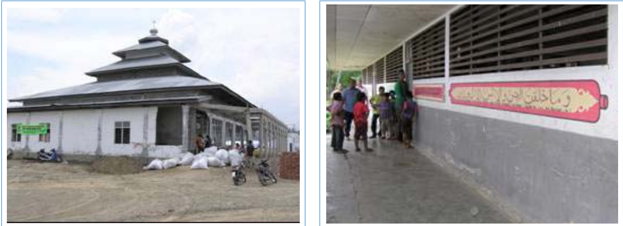
Figure 1 Examples of surviving masonry structures
