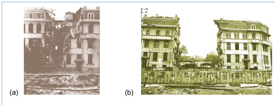
Figure 8 Bucharest, 4 March 1977: heavy damage to two University buildings built at the end of the nineteenth century. (a) Effect of bombing during the Second World War – (b) 1977 earthquake impact on the Faculty of Chemistry (photo © UTCB D. Lungu)
