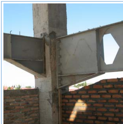
(a) Castellated beams in a bolted steel frame and concrete encased columns
