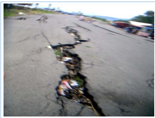
Figure 3 Liquefaction: (a) lateral movement causing a road to crack, Jl. Samudera, and (b) sand from the bottom of a road experiencing landslides, Jl. Samudera
