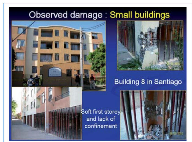
Figure 15 Typical failures due to lack of confinement in compressed wall heads and thin walls
