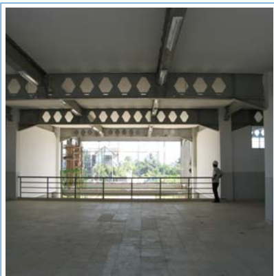
(a) Castellated beams in a bolted steel frame and concrete encased columns
