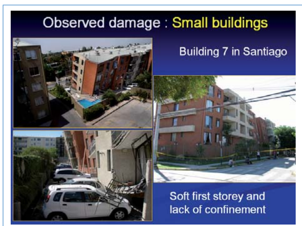
Figure 15 Typical failures due to lack of confinement in compressed wall heads and thin walls
