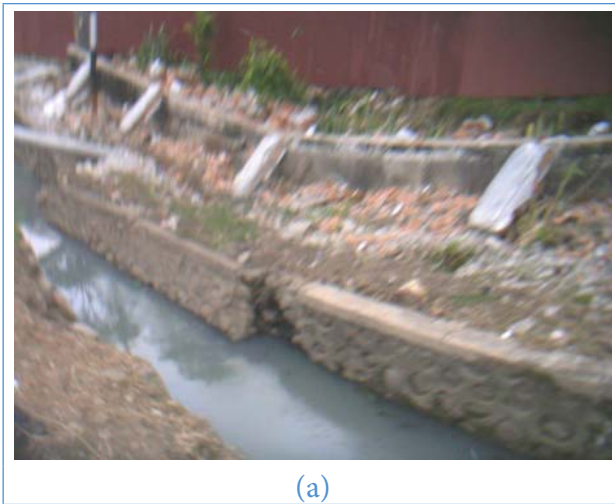
Figure 2 Liquefaction: (a) deformation of the soil layer due to the river wall breaking, Jl. Gereja, and (b) differential settlement of subgrade foundations
