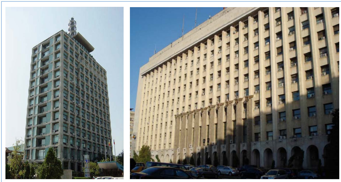
Figure 11 (a) National Romanian Television building, and (b) a reinforced-concrete flexible building built in the 1960s and the Ministry of Transport, Construction and Tourism, built in the 1930s
