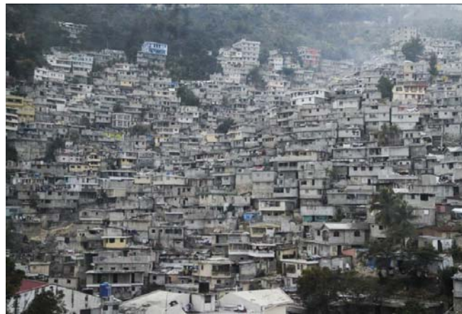
Figure 3. The chaotic urban development in Port-au-Prince has led to increased vulnerability of slope stability under seismic demand, as well as under gravitational load (Photo by Eduardo Miranda, 2010)
