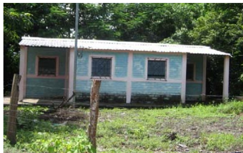
Figure 3. Intermediate beam used in confined masonry in El Salvador
