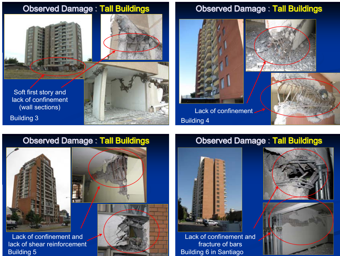
Figure 5. Typical observed failures due to the poor confinement in shear wall boundary elements.
