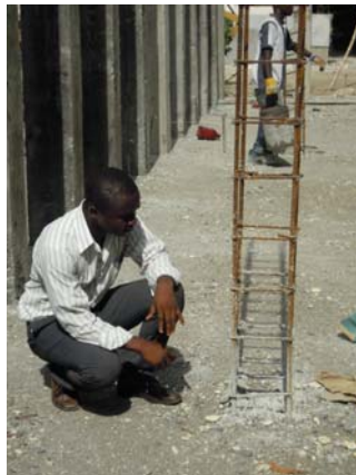
Figure 2. The reinforcement detail in the Haitian Construction Code is not adequate for medium to severe seismic demands
