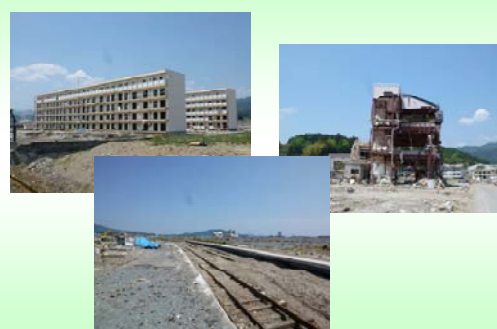
Figure 20. Tsunami-induced damage in Rikuzentakata city, Iwate (2011 ©T. Imamura)
