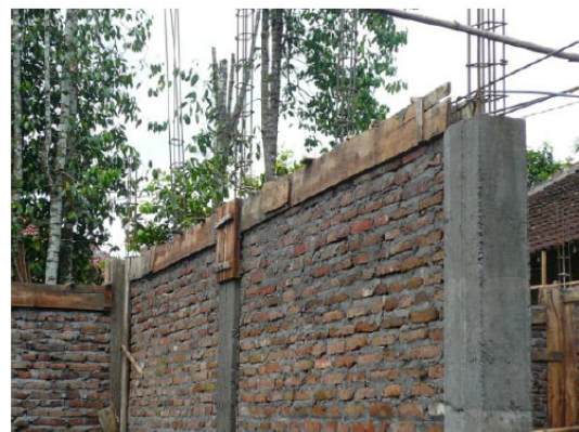
(b) Two storey house under construction (Jawa)
