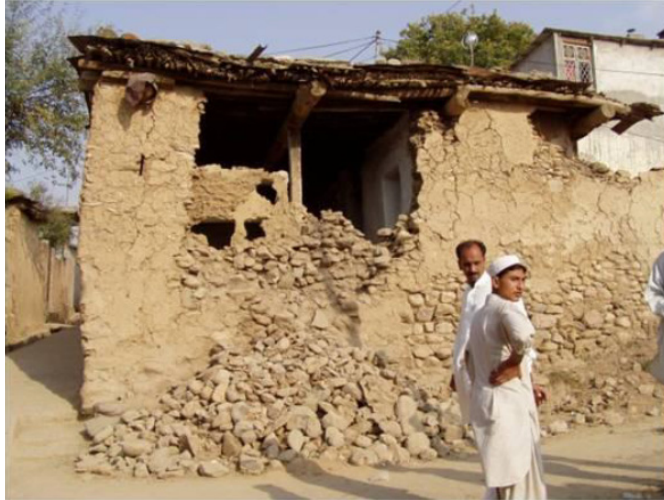
(a) Unreinforced stone masonry
