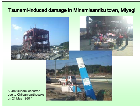
Figure 22. Tsunami-induced damage in Minamisanriku town, Miyagi (2011 ©T. Imamura)
