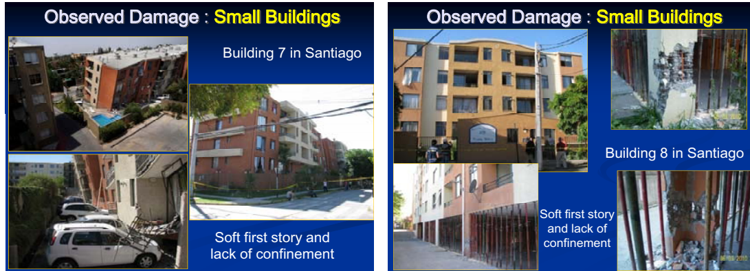
Figure 6. Typical observed failures: poor confinement in shear wall boundary element, vertical reinforcing steel buckling, and development or splice length failures in thin shear walls.
