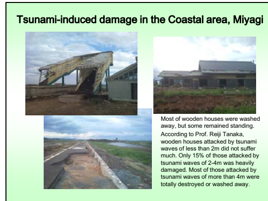
Figure 24. Tsunami-induced damage in the coastal area, Miyagi (2011 ©T. Imamura)
