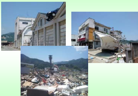
Figure 19. Tsunami-induced damage in Oofunato city, Iwate (2011 ©T. Imamura)
