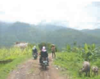
Rugged road condition
