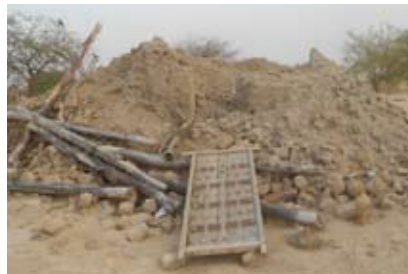
Destroyed Cheick Sidi Aboulkhasoum Mausoleum © DNPC
