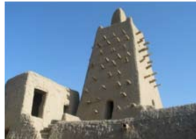
Djingareyber Mosque, Timbuktu © DNPC
