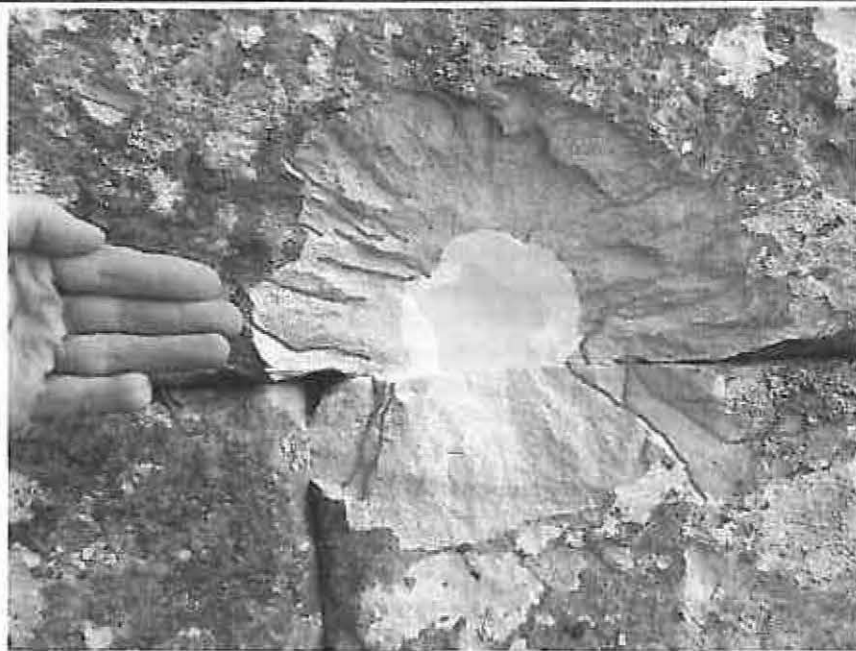
Fig. 2 Mapping indicating the different forms of damage caused by the impact of a projectile at Preah Vihear.
