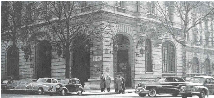
Former UNESCO Headquarters – Avenue Kleber, Paris
