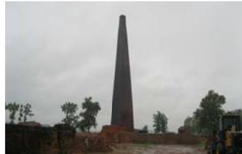
Photo 7. Smoke Stack of Brick Factory (Due to heavy rainfall the factory was closed during the field visit)
