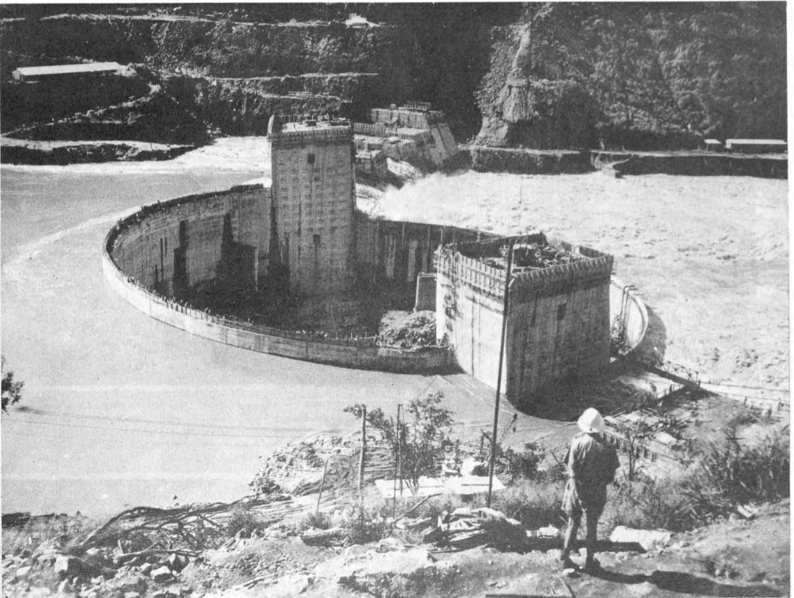
A few days after this picture was taken in March 1958, the swirling flood waters of the Zambezi River broke over the wall of the coffer dam erected in midstream for the giant Kariba Dam hydro-electric power station being built in the Federation of Rhodesia and Nyasaland (photo of flooded coffer dam is shown next page). For the Kariba Dam, one of the world's most ambitious engineering projects, the International Bank for Reconstruction and Development has made loans totalling $80 million, the World Bank's largest loan in Africa, and its largest for a single undertaking to date.
