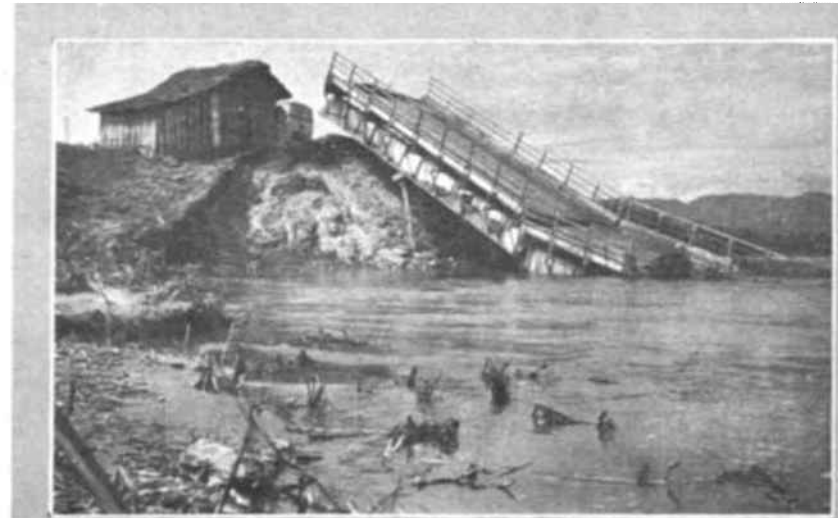
Ranganadi Bridge, (above) near the town of North Lakhimpur, was swept away by a giant wall of water after the river, blocked by boulders in the hills, had burst its way free. This 1,100 foot bridge was of vital importance, being the longest in Assam.
