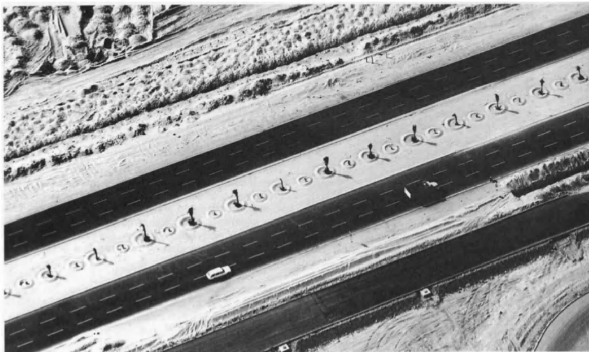
A new super highway rakes across the desert in Abu Dhabi, United Arab Emirates. The construction of adequate networks of roads and highways is a key factor in the development process, but the burden of road maintenance weighs heavily on the developing countries (see box below).
