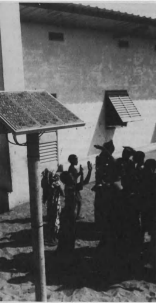
Photo Stambolis © Unesco. From Solar Energy for Educational Buildings , by C. Stambolis with P. Vastardis, Heliotechnic Press, London 1981
